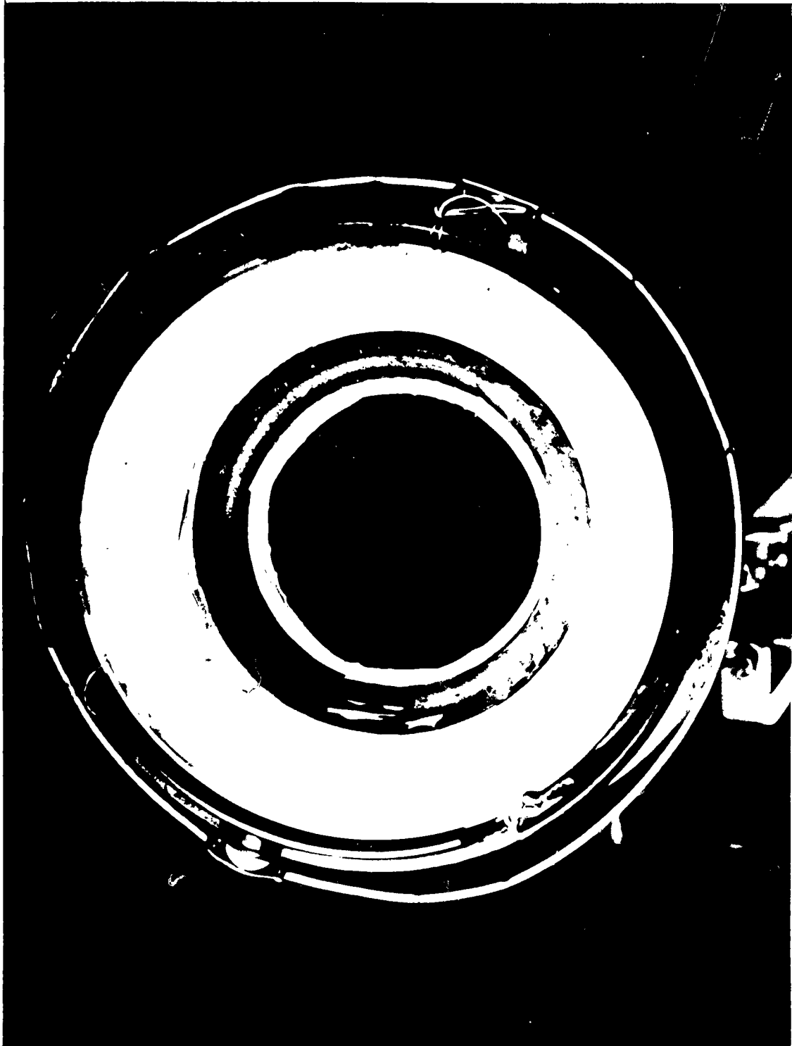
FIGURE 10. Masking Tape Applied Around Area to Receive Sealing Compound.
