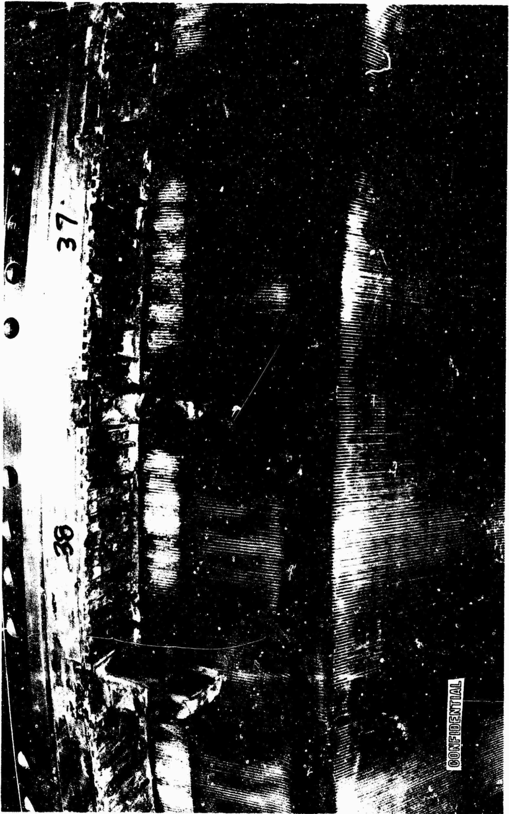
Figure 336. Eroded Baffles
