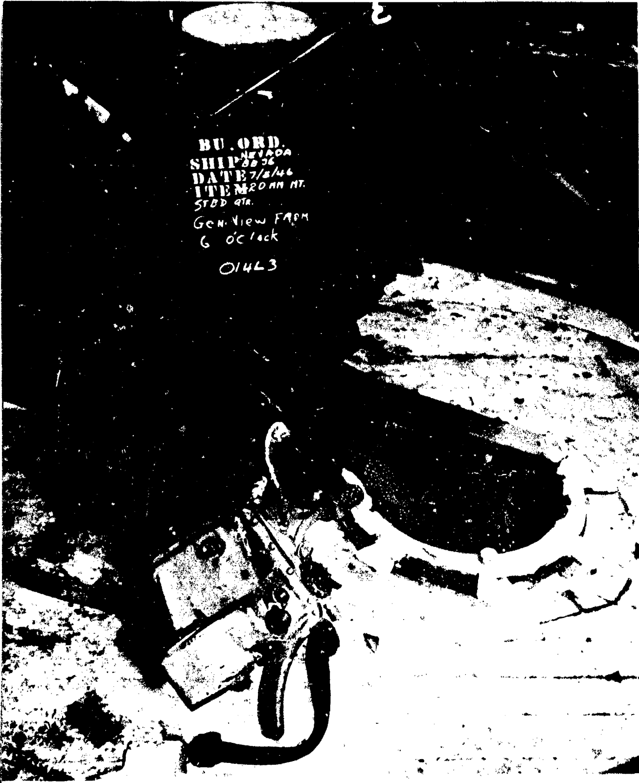
U.S.S. NEVADA (SS-36) - After Able General view of 20 MM twin Mt. No. 7 showing the demolished stand. Photo. No. 4A-6K-97-1939-3.
