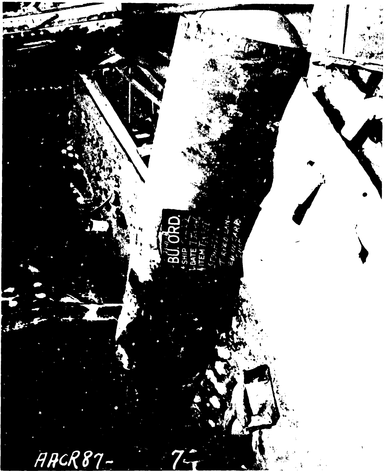
U.S.S. INDEPENDENCE (CVL-22) - After Able Service Load Torpedoes in normal stowage. Torpedo landed in carpenter shop. Photo. No. AA-CR-87-21 A-7.
