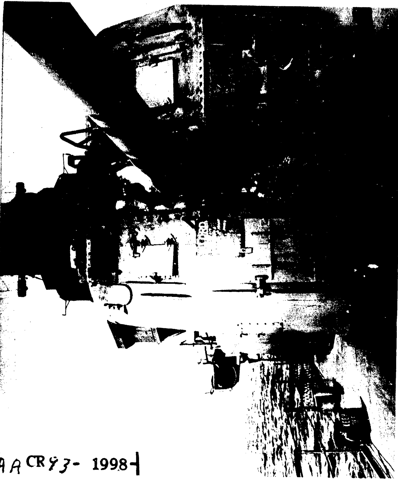
U.S.S. WAINWRIGHT (DD-219) - After Able General view of 5"/38 Mt. No. 1, Showing burned gun port gas seal and scorched exterior paint caused by burning Gun Port bloomer. Photo. No. AA-CR-93-1998-7.
