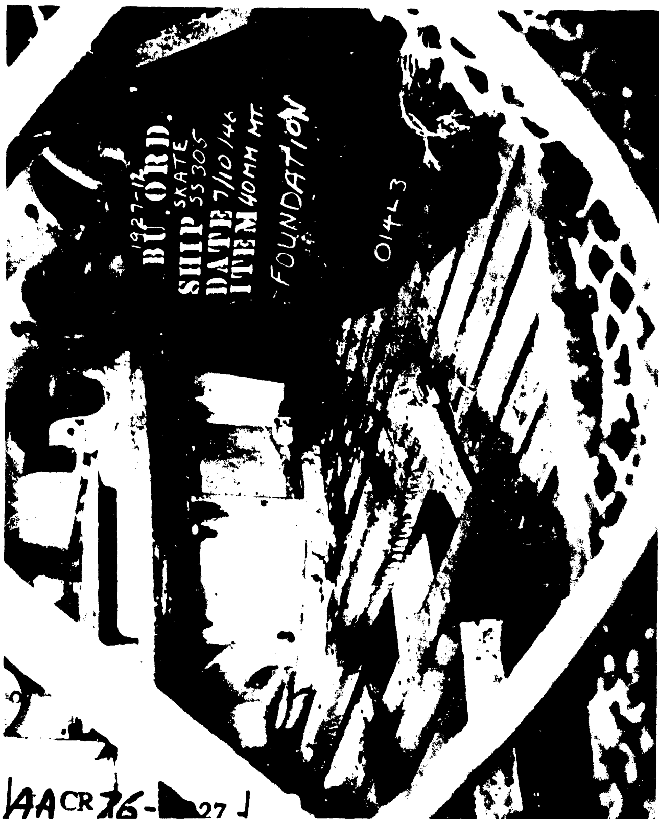
U.S.S. SKATE (SS-305) - After Able View of 40 MM Single Mt., showing the foundation intact. Photo. No. AA-CR-76-1927-12.
