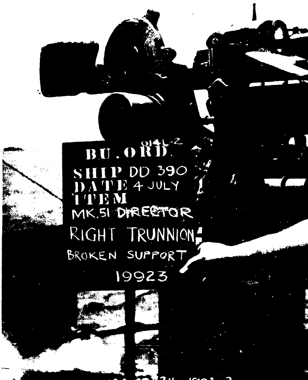
U.S.S. BELLEFLORE (DD-390) - After Action Gun Director, Mk. 51, No. 1, Serial No. 246 (Atop the After Deck House) Showing the broken trunion support of the gun sight, Mk. 14, Mod. 8, Serial No. 112801, and the location point on right-hand side of the gun sight. Photo. No. AA-01-237-1992-3.
