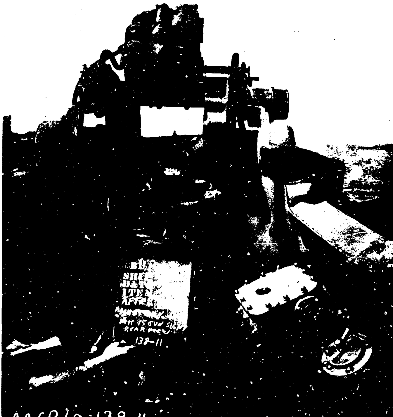
U.S.S. ARKANSAS (BB-33) - After Able Gun Director, Mk. 51, Mod. 3 (Starboard after air defense) Showing bent splinter shield and broken air drier fitting. Photo. No. AA-CR-60-138-11.
