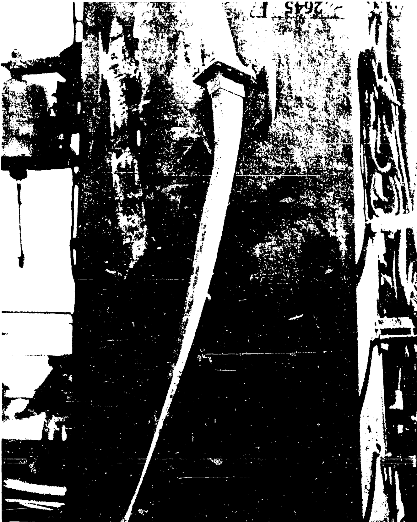
POST ABLE - FOREMAST. Close-up of flattened and twisted SG waveguide.
