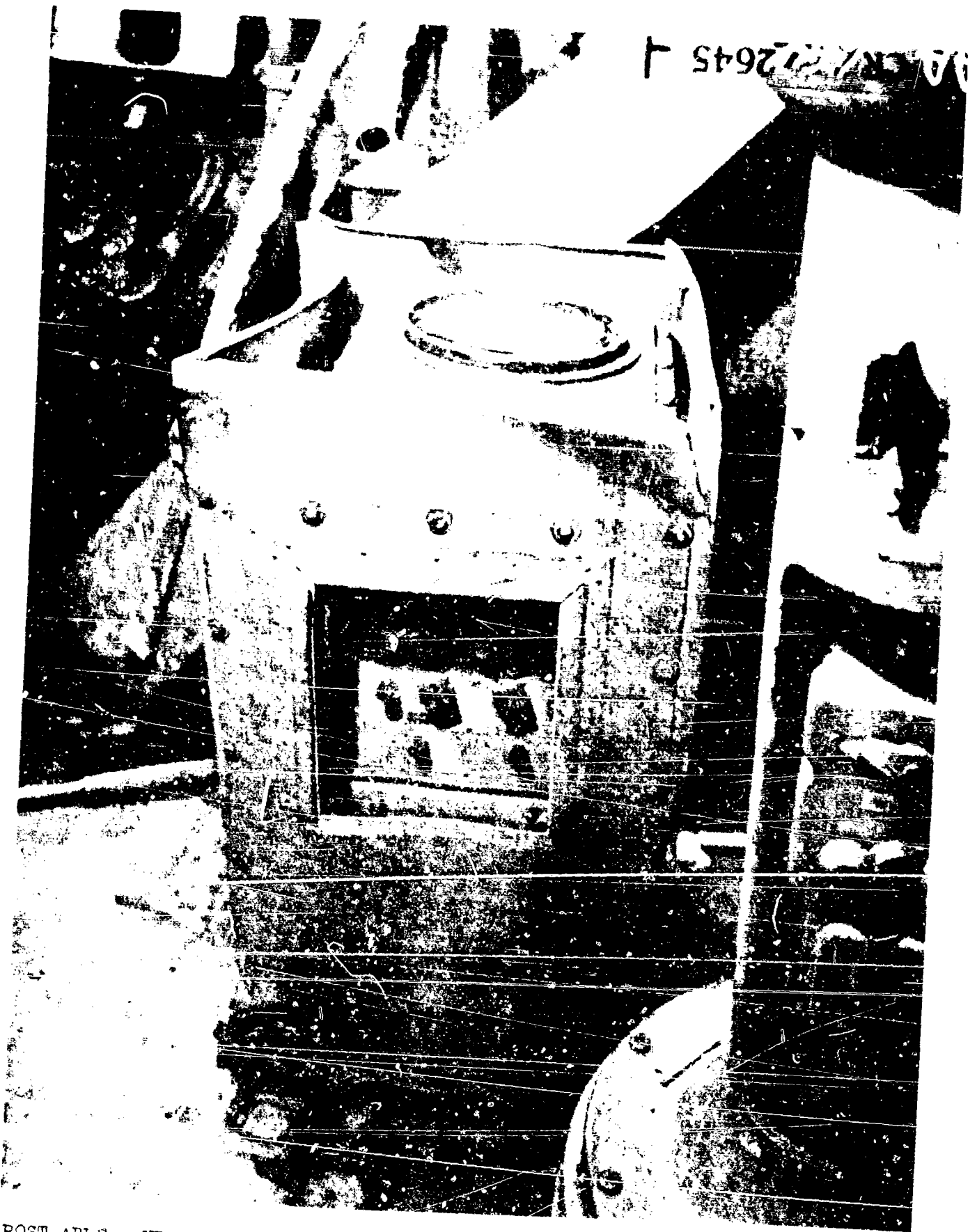
POST ABLE - VD-2 Equipment on open bridge. Welds parted on foundations, and subsequent movement of VD-2 parted cables. Housing sides were warped and top blown off, but VD-2 was apparently undamaged.
