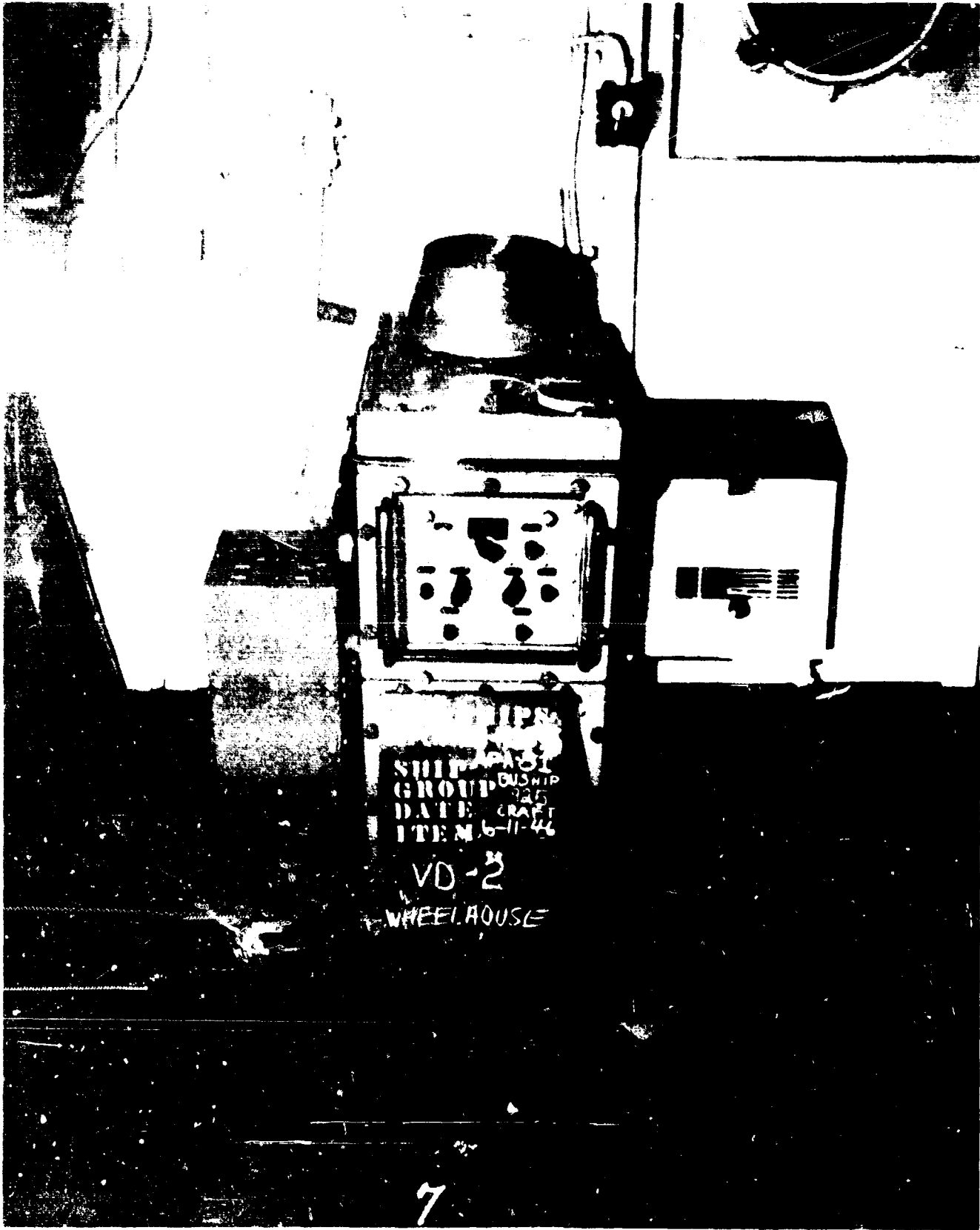
PRE BAKER - VD-2 FRONT VIEW. This equipment was undamaged during Test Able.
