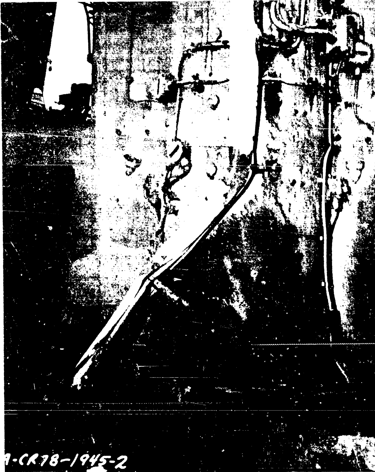
POSSIBLE - COAXIAL LINE. The MK 4 coax was broken and bent by the blast.
