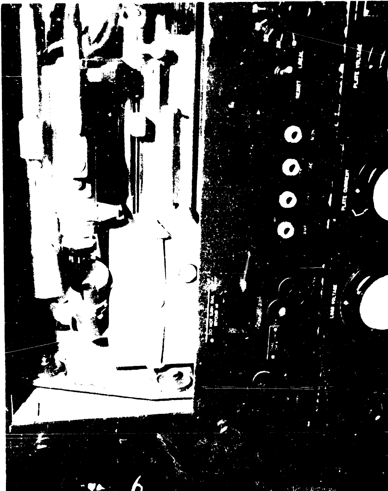
POST BAKER - FORWARD MK 4 RADAR RF AMPLIFIER UNIT. Socket was knocked off and bent. This main frame was not shock mounted.
