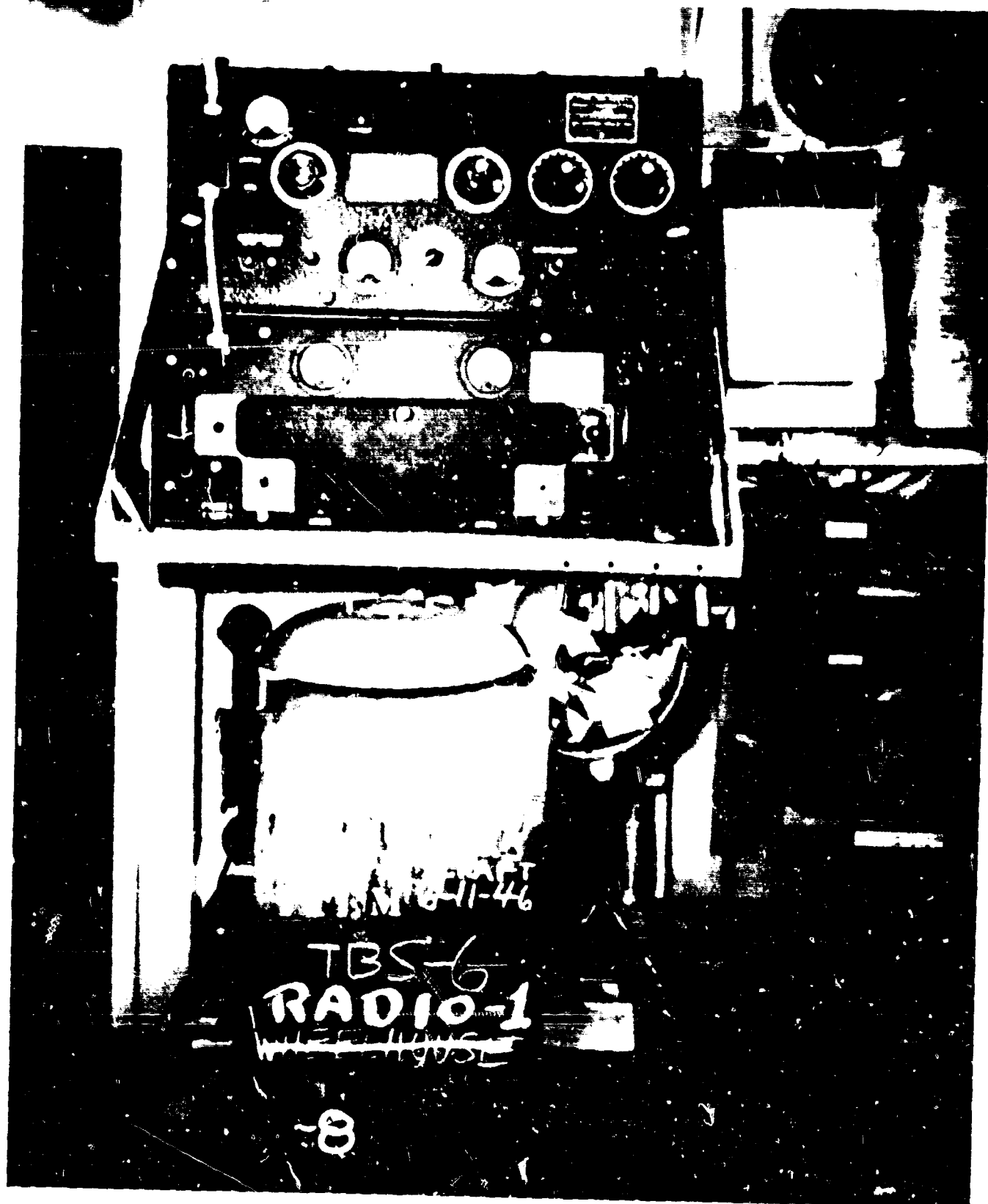
PRE BAKER - RADIO I. View of TBS-6. This equipment was undamaged during Test Able.
