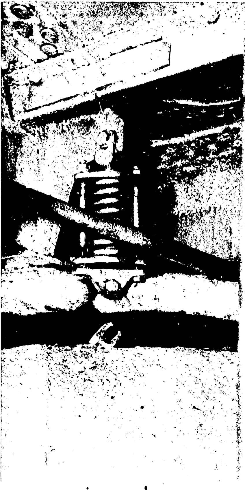
AB-CR-68-2951-7. Showing broken hanger on 7" main steam line to L.P. turbine, No. 1 engine room.
