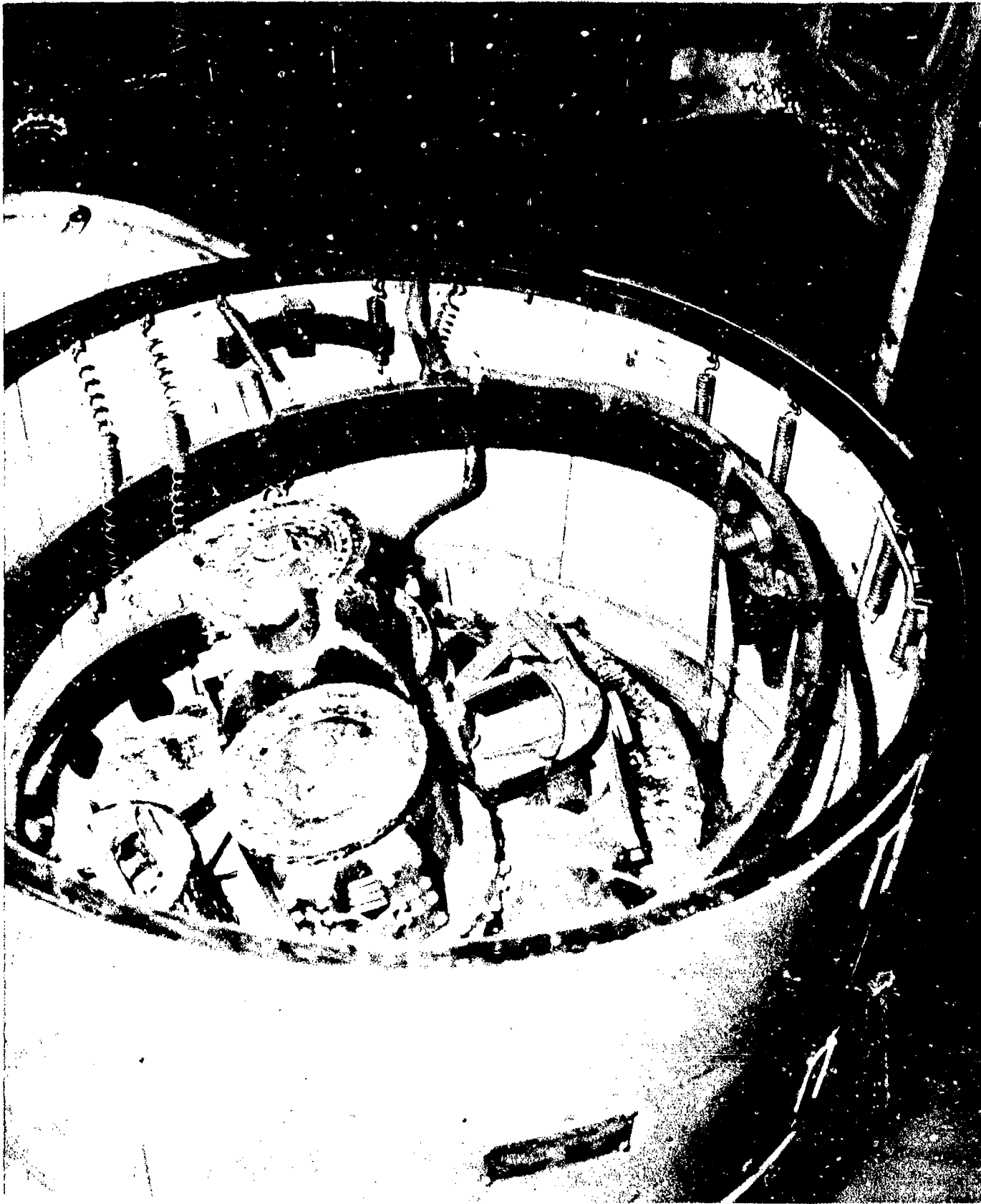
AB-CR-76-1934-1. Gyro compass mounted in the I.C. room. Shows damage to the gimbal mount, and gyro element dropped to the bottom of the binnacle. Dirt and silt were caused by flooding of the space.
