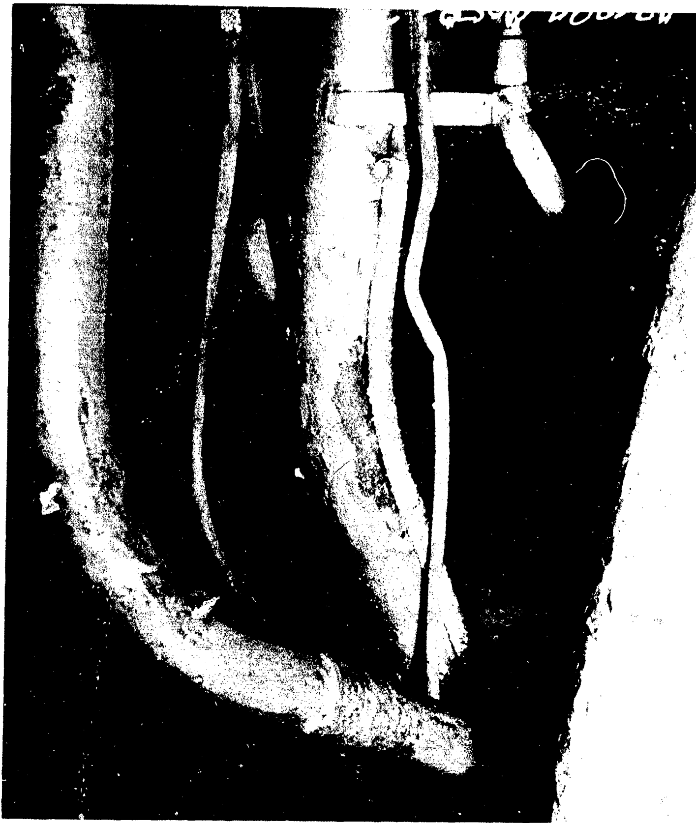
AB-CR-97-4058-2. Aft engine room, B-4-1. The center 3 1/2'' diameter pipe is a buckled surge tank support located at starboard of centerline at frame 129, looking aft.
