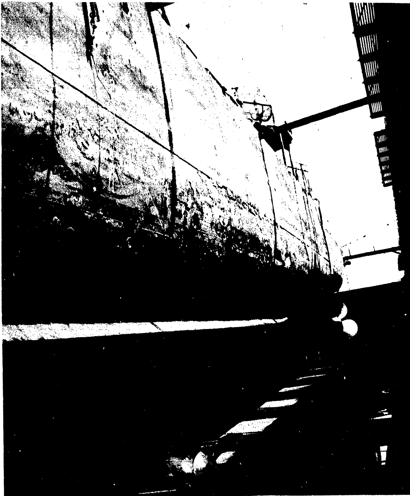
AB-CR-97-4057-1. Port shell looking aft, frames 100-130.
