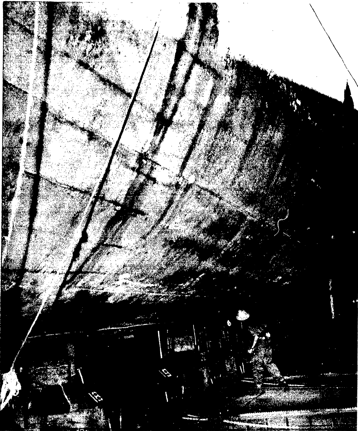
AB-CR-97-4048-3. Port shell looking aft, frames 40-60.
