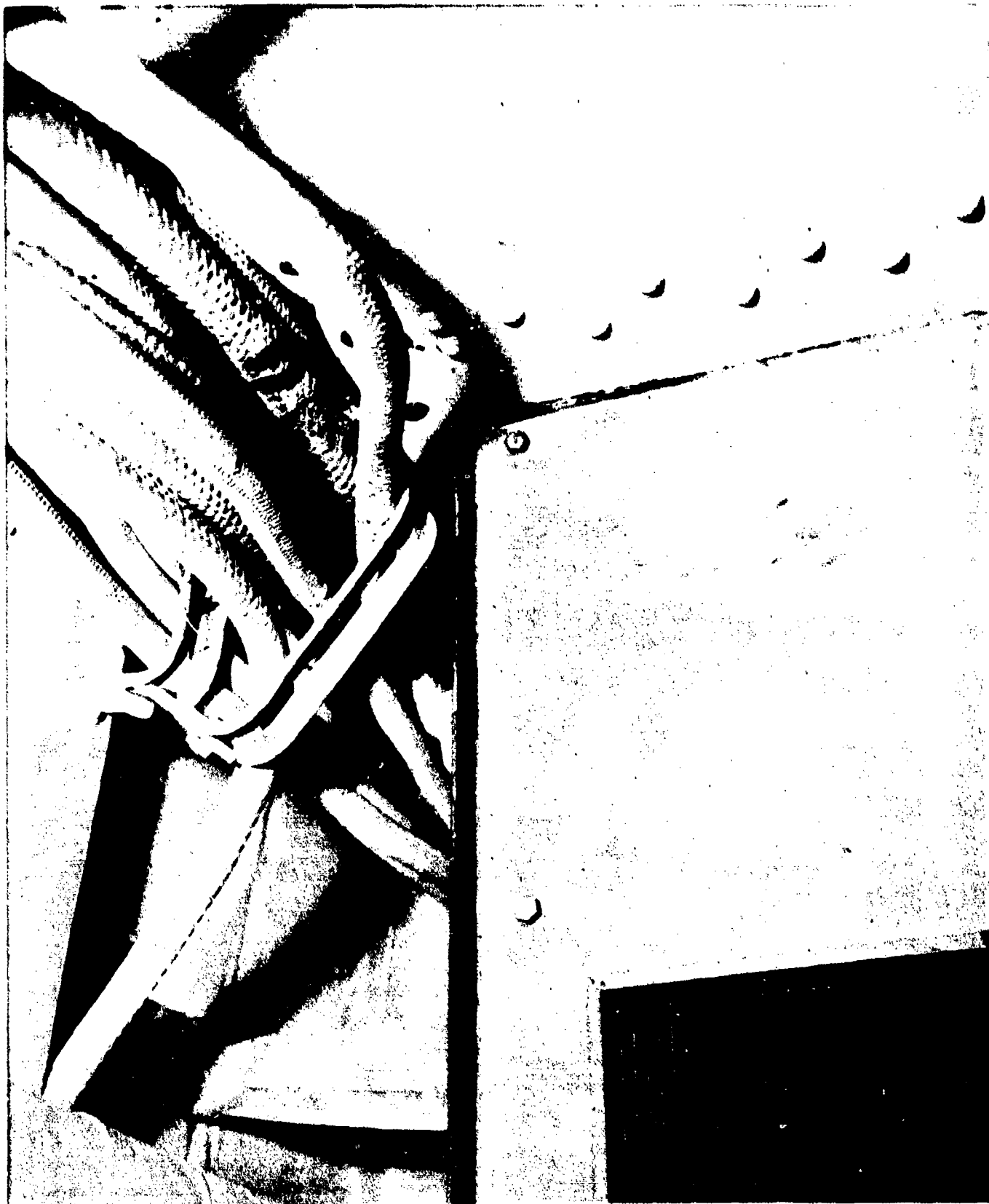
AB-CR-76-1932-10. Longitudinal wireway in battery charging and electric workshop. Shows damaged wireway support. Cables obscure sheared strap bolt. Picture taken looking to port.
