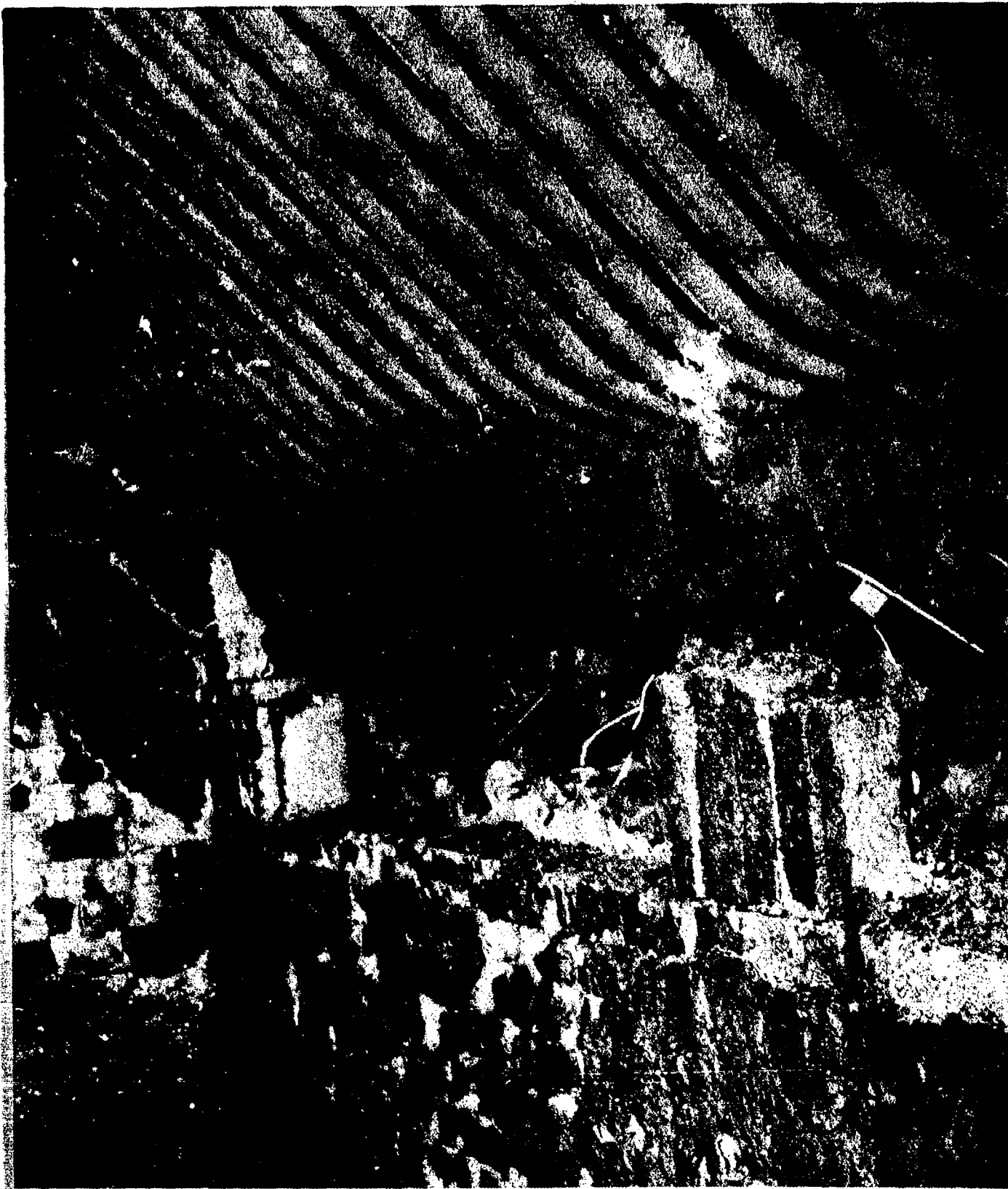
AB-CR-68-2951-11. Interior, saturated side No. 1 boiler, showing displaced brickwork.
