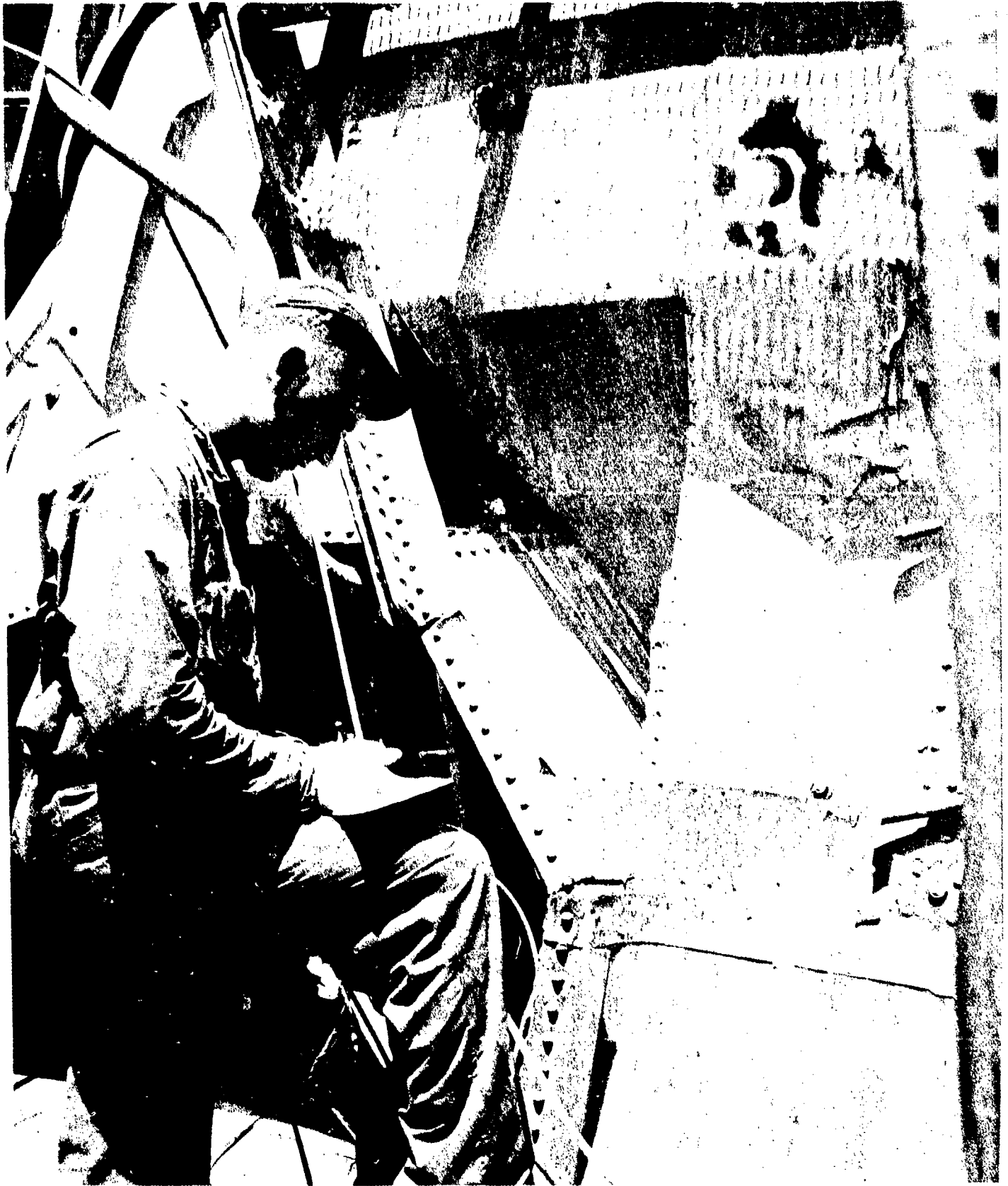
AB-CR-76-2078-1. No. 2 boiler uptake, port side.
