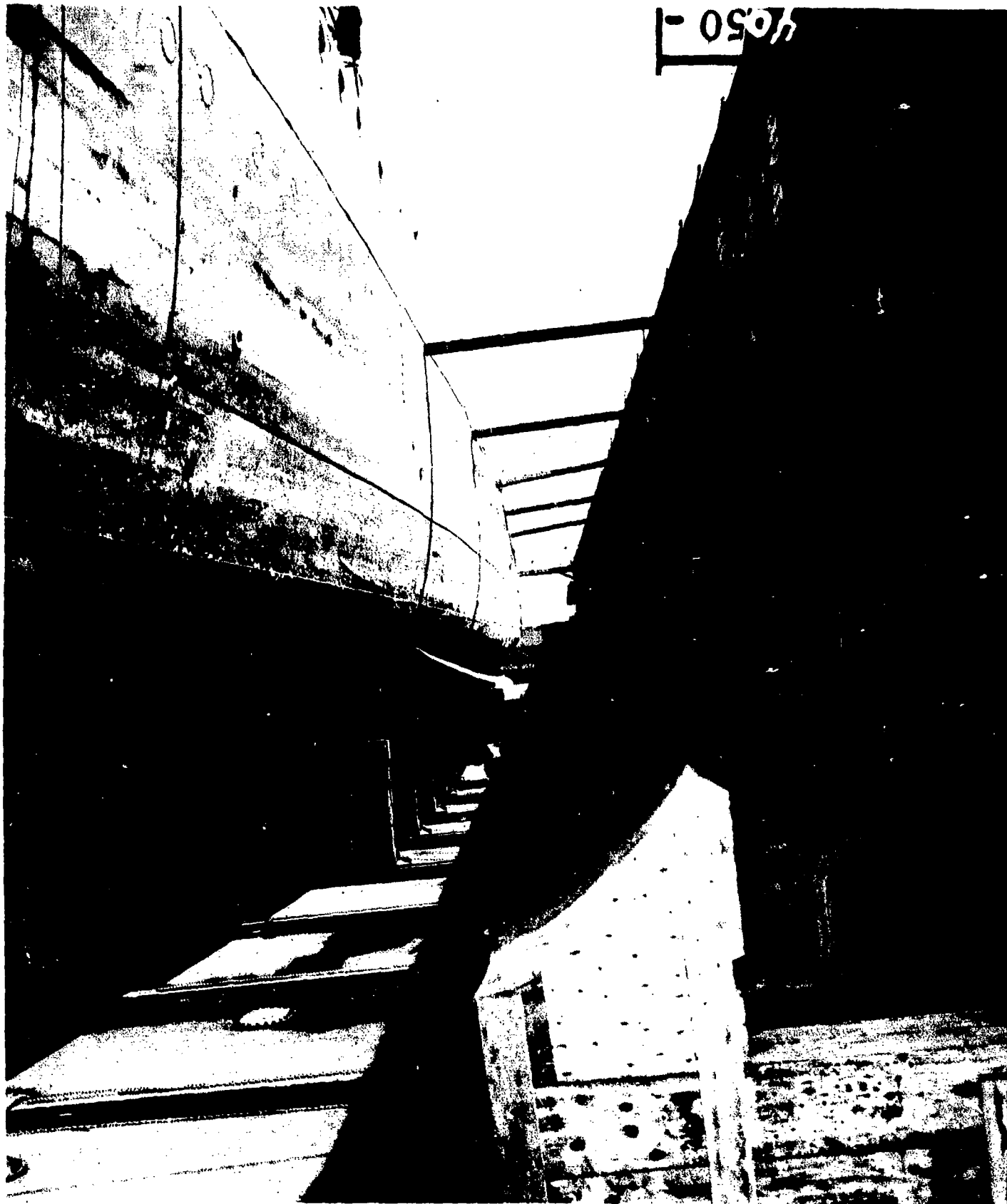
AB-CR-97-4050-10. Port shell looking aft, frames 40-60.
