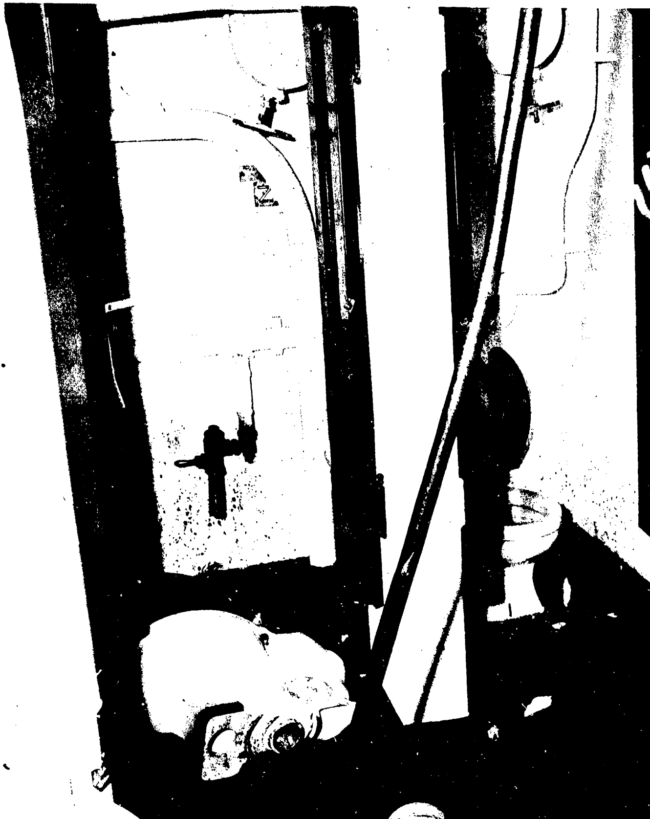
AB-CR-100-4211-4. Looking forward on main deck port side, to bulkhead 25 showing broken toilet bowl, piping and ammunition cans.
