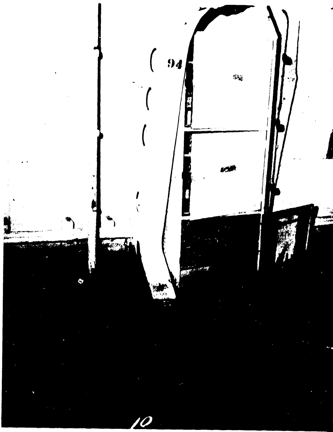
AB-CR-76-2081-10. Second deck, looking outboard and to starboard at frame 94.
