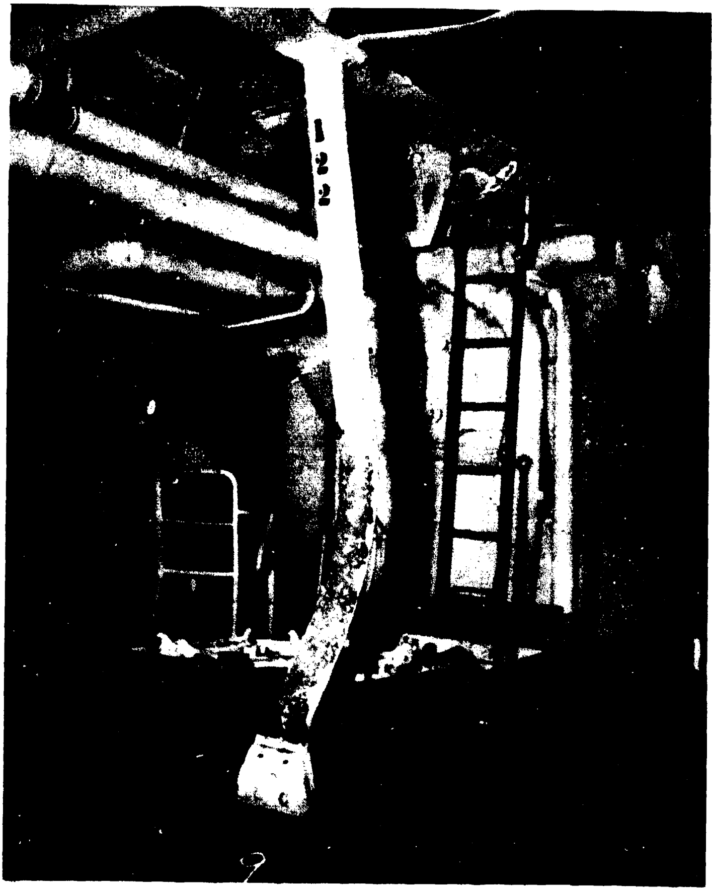
AA-CR-175-2178-9. D-203-L. Test able damage. Looking aft and to port at quarter span stanchion, frame 122, starboard. Compare with 2082-2.
