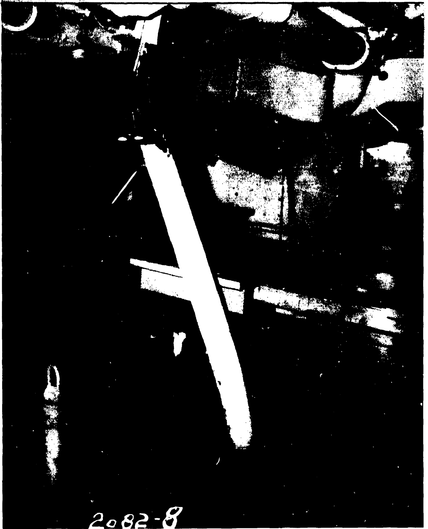
AB-CR-76-2082-8. D-203-2L. Looking forward and to port at centerline stanchion, frame 130. Compare with test able damage shown in 2179-4.
