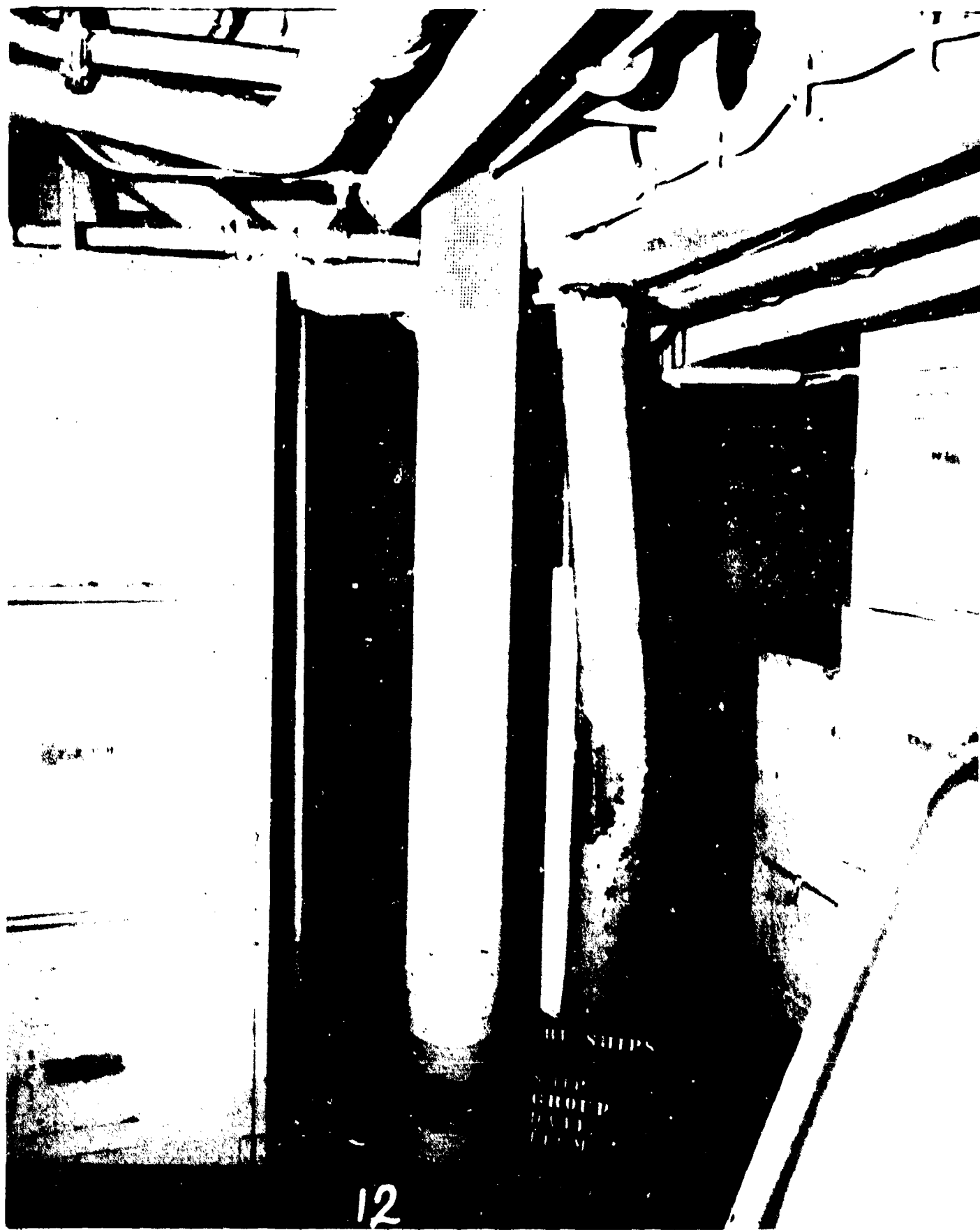
AA-CR-90-574-12. C-202-L. Second deck frame 97, port side. Note deformation of stanchions and crack around top under beam.
