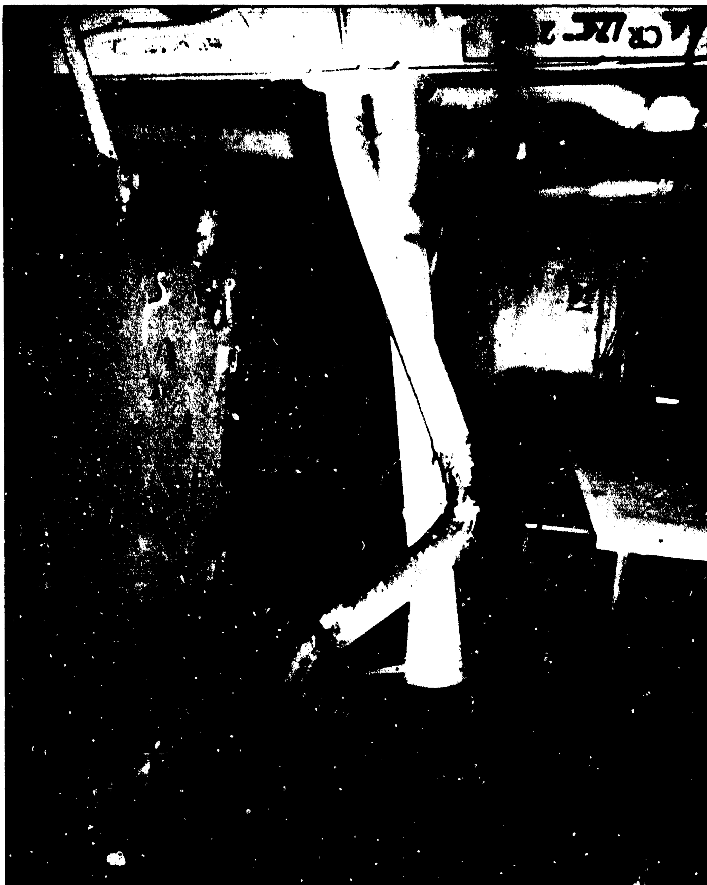
AA-CR-175-2178-2. Second deck, starboard outboard stanchion. Frame 125. Test able damage.
