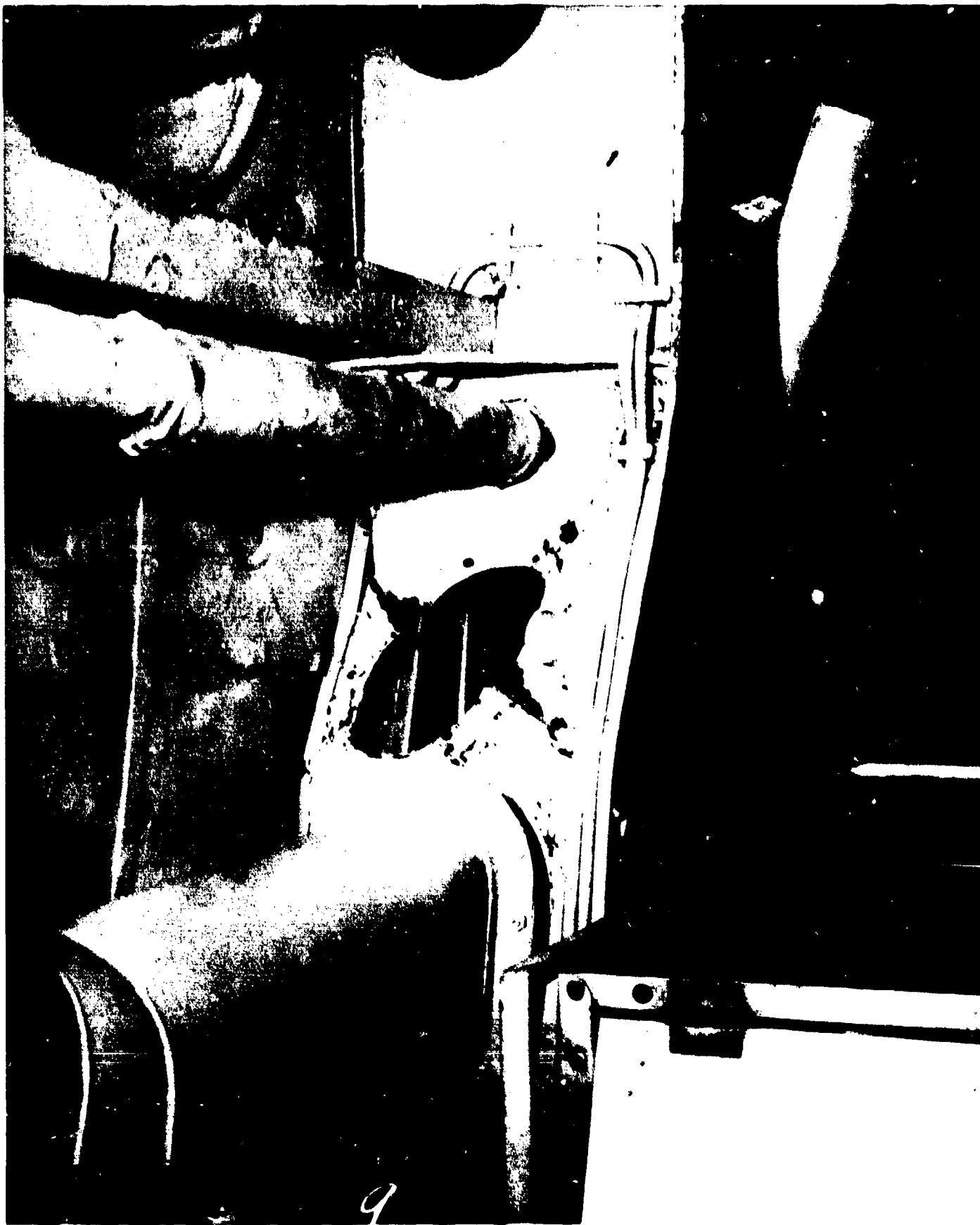
AB-CR-76-2082-9. D-204-L. Looking aft at failure of transverse girder in way of lightening hole. Frame 135, compare with test able damage shown in 2174-7.
