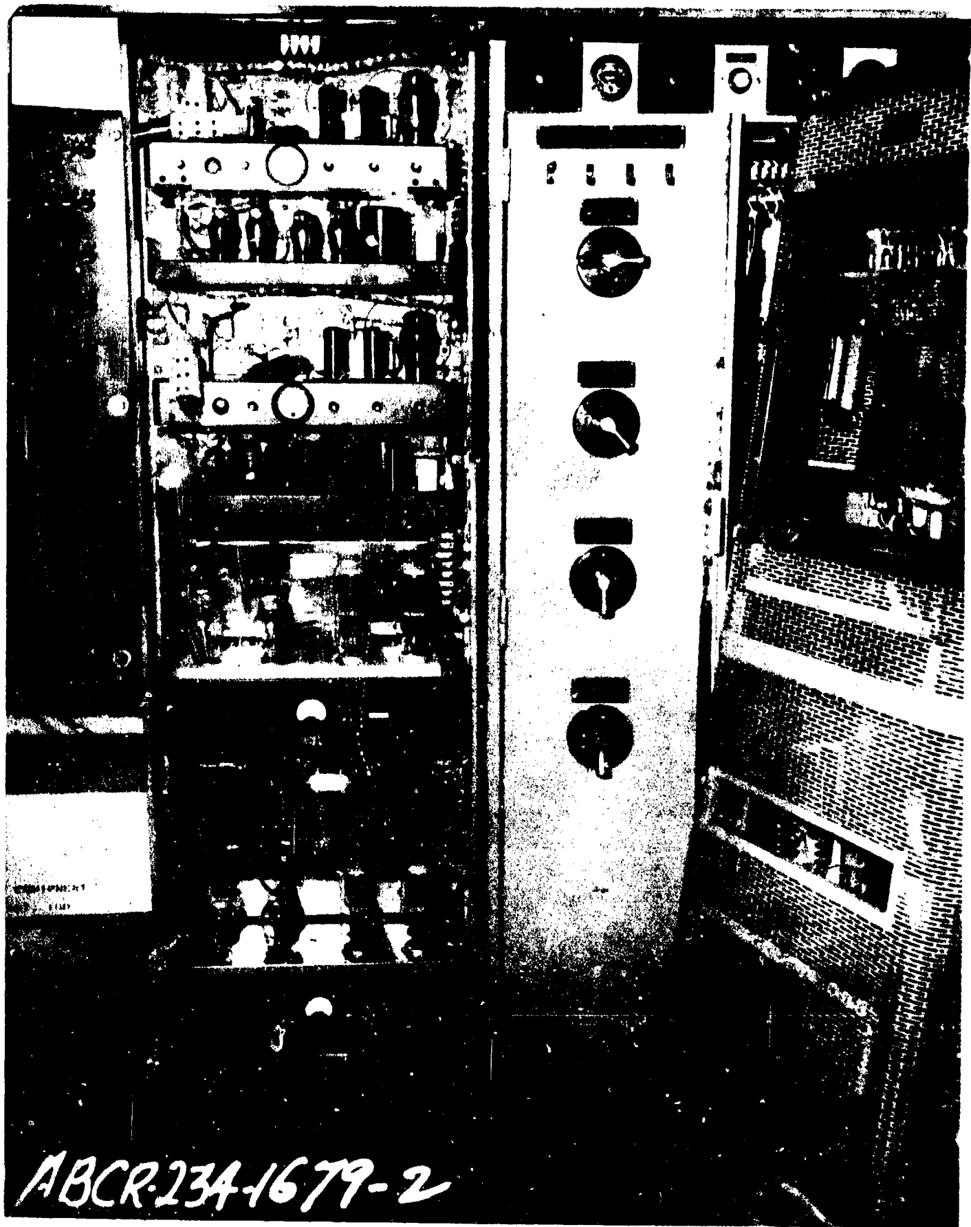
AB-CR-234-1679-2. Front view of MC amplifier rack with dislodged vacuum tubes. Located in central station.
