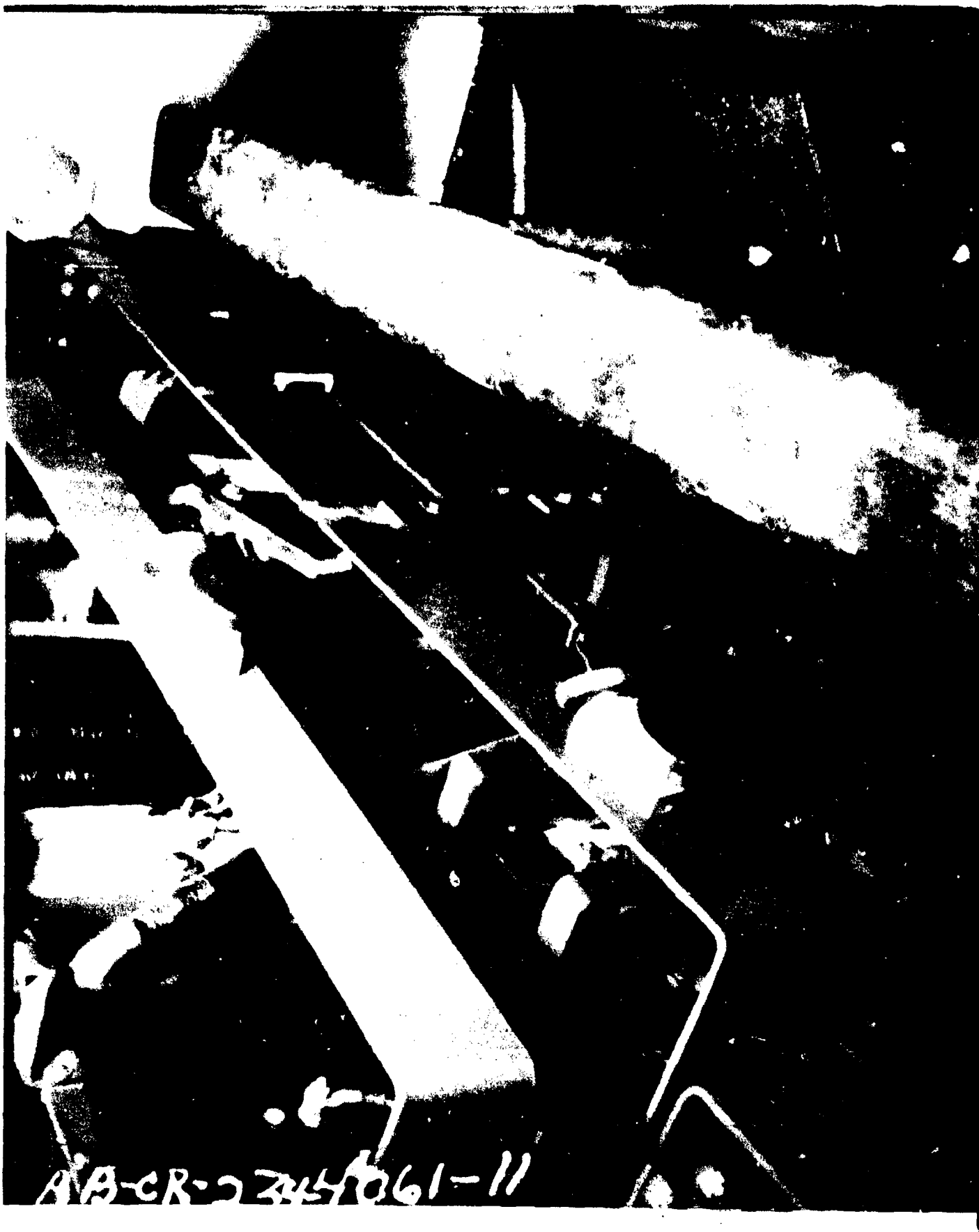
AB-CR-234-4061-11. Ebony asbestos blocks installed behind the forward ship's service generator to prevent vibration of busses. Blocks were broken. Taken behind switchboard looking to starboard near outboard end of switchboard.
