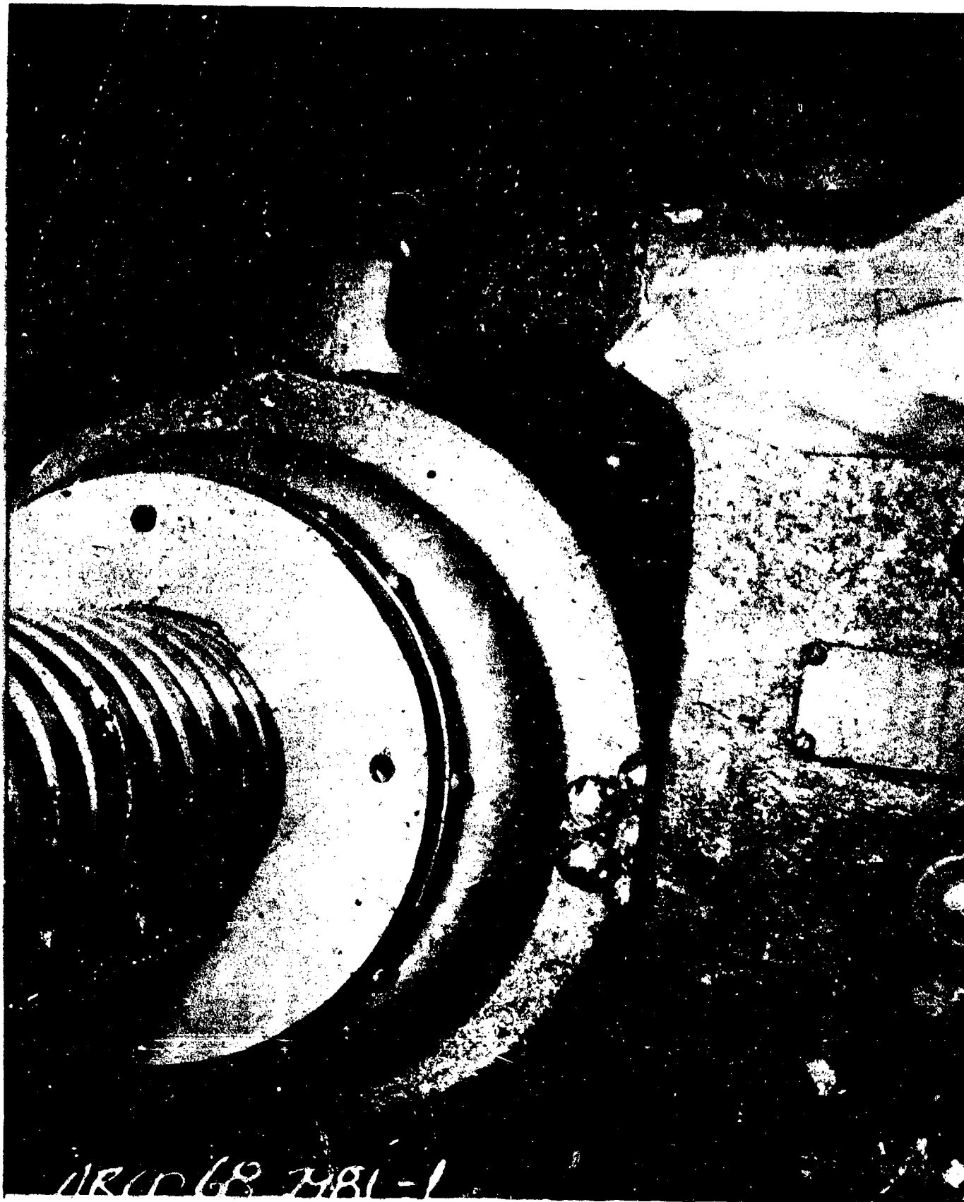
AB-CR-68-2981-1. Right gun of Turret 3, elevating screw oscillating bearing, looking down and to front showing top assembly pulled out of position and ball bearings scattered.
