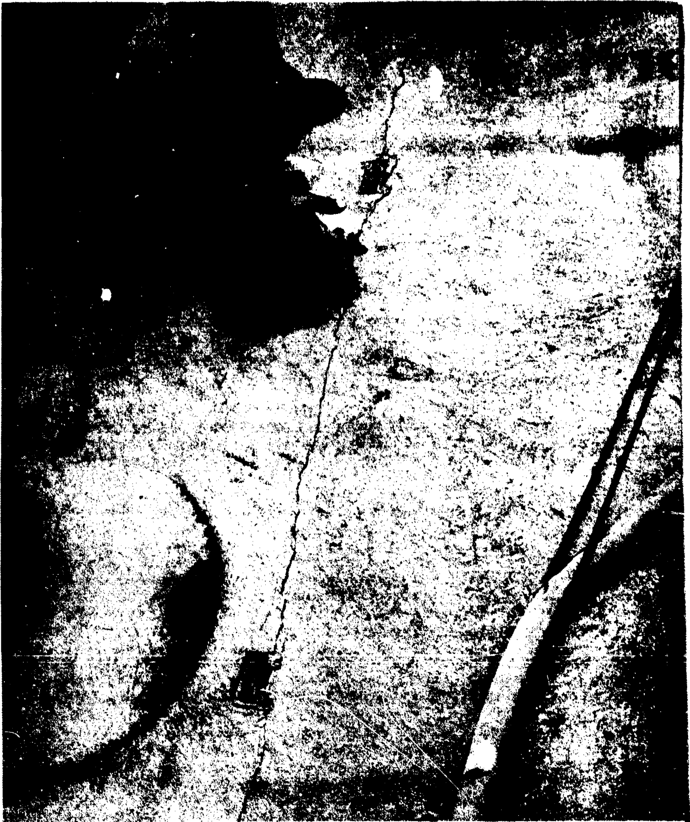
AA-CR-98-1964-1. View of crack in port "A" deck.
