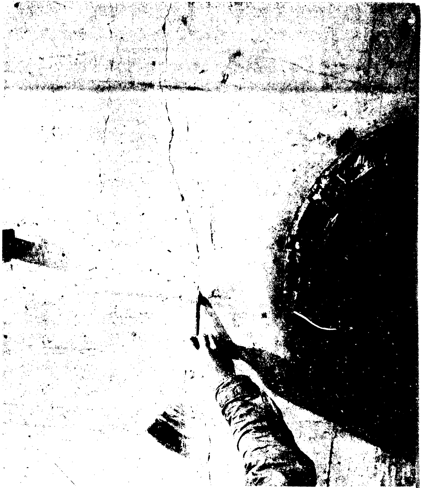
AA-CR-98-1963-5. View of crack in after inside face of starboard wing wall.
