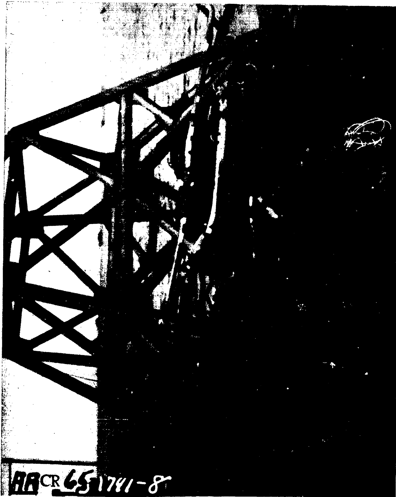
AA-CR-65-1741-8. Looking forward and to starboard, on starboard side of signal bridge, showing damage to railings, in way of starboard flagbag location. The flagbag was blown to the level below.
