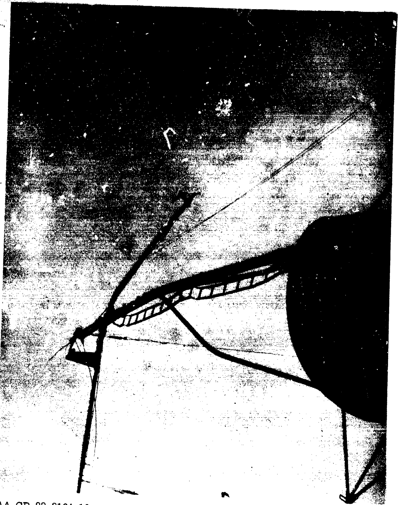
AA-CR-88-2104-10. Looking up, aft, and to port, showing damaged signal mast and yardarm at forward edge of forward stack.
