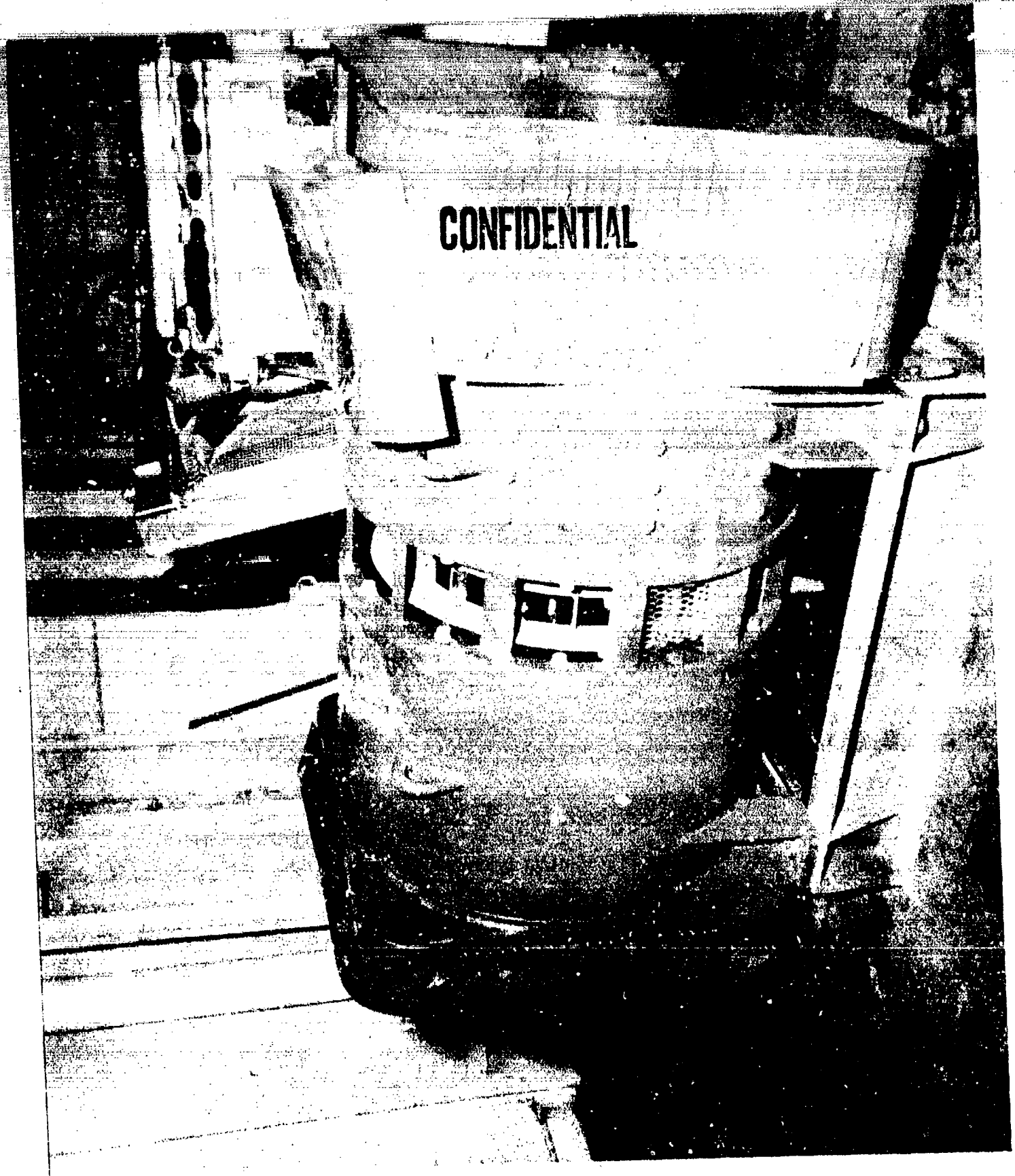
AA-CR-78-127-7. 75 K.W. M-G set located in the forward cargo hold. Shown after the debris was cleared away. Code 660, 12E4.
