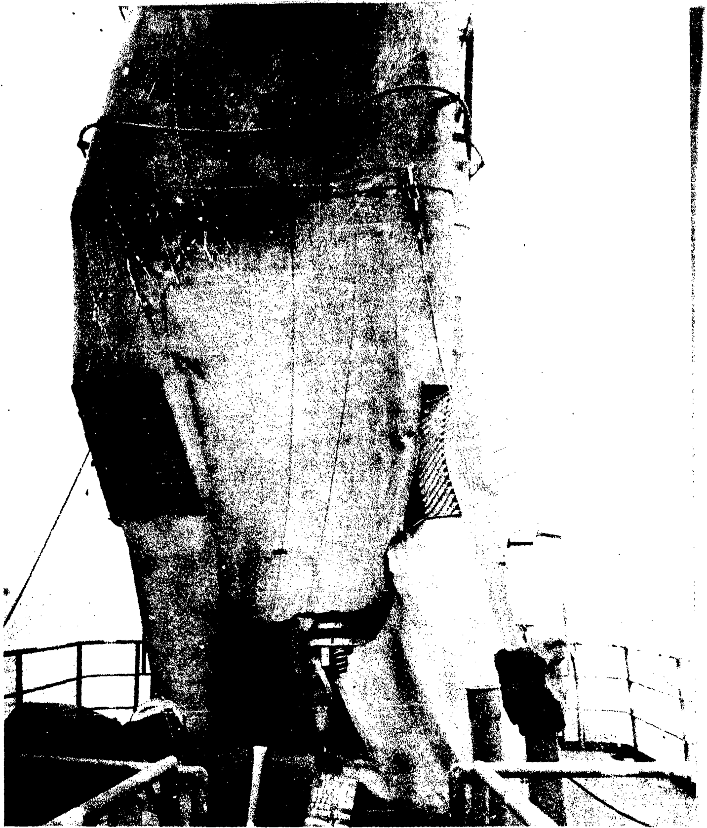
AA-CR-62-1878-4. Looking aft at damage to after stack.
