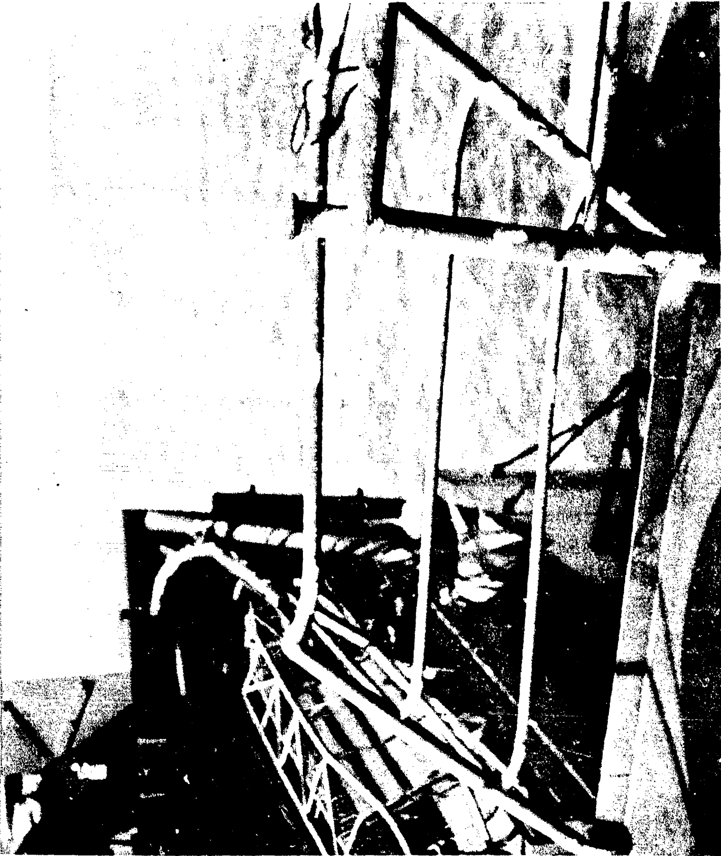
AA-CR-59-2058-8. Looking to starboard and forward on starboard wing of signal bridge showing distortion of railings.
