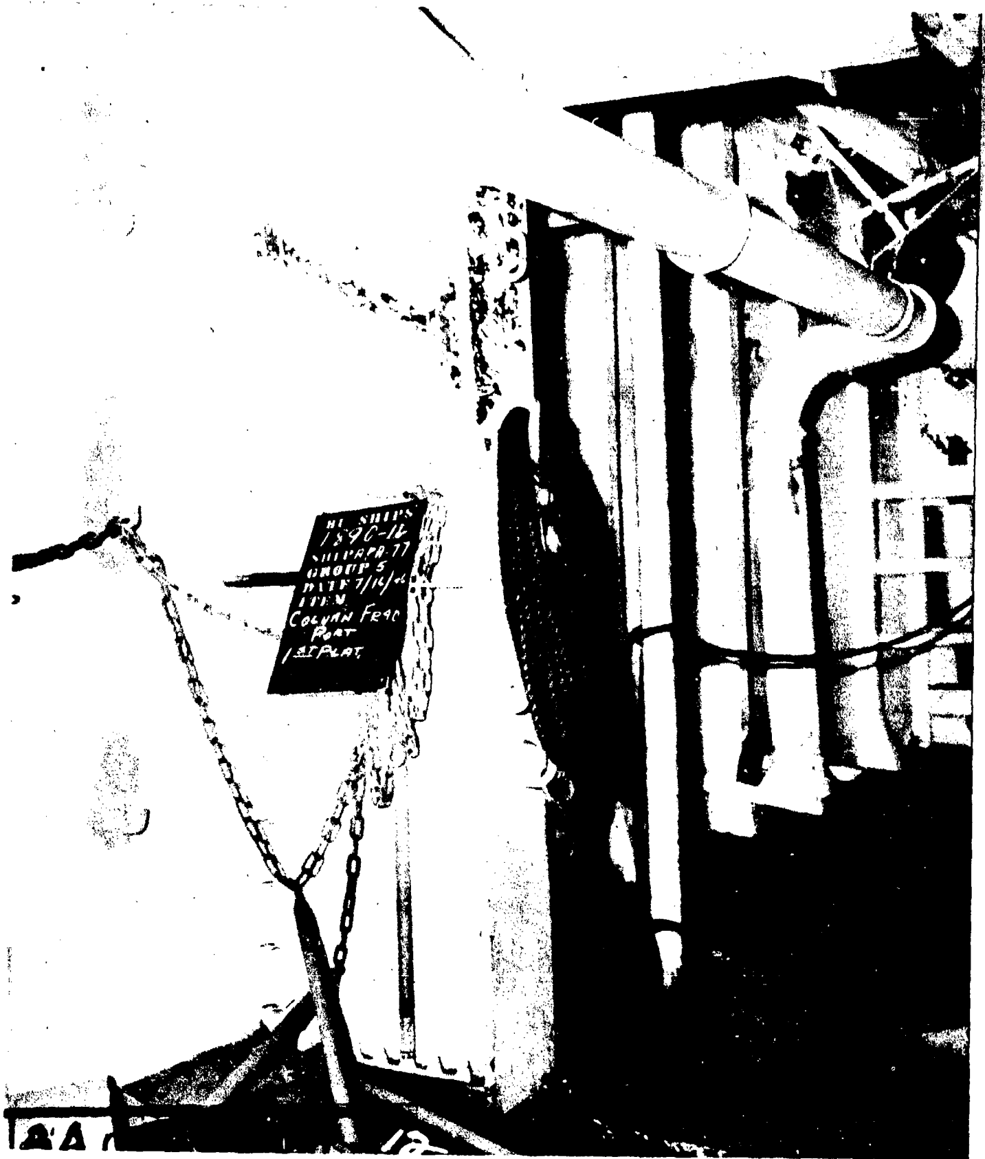
AA-CR-100-1890-12. Looking forward and to starboard along bulkhead 40 on first platform in forward cargo hatch area showing damage to column in way of port edge of hatch.
