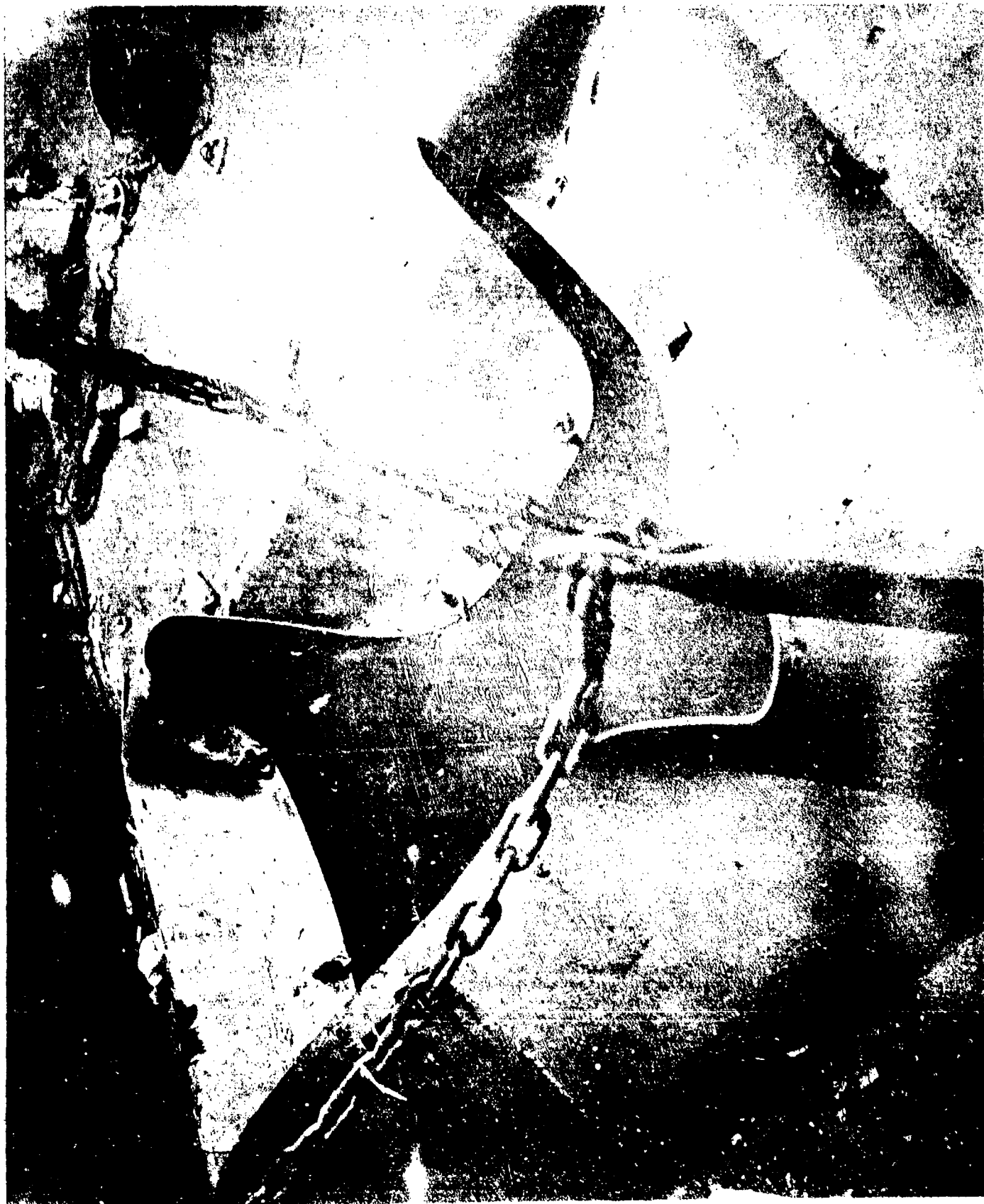
AA-CR-98-1961-1. Looking aft and to port on upper deck showing damage - to coaming of ammunition trunk hatch.
