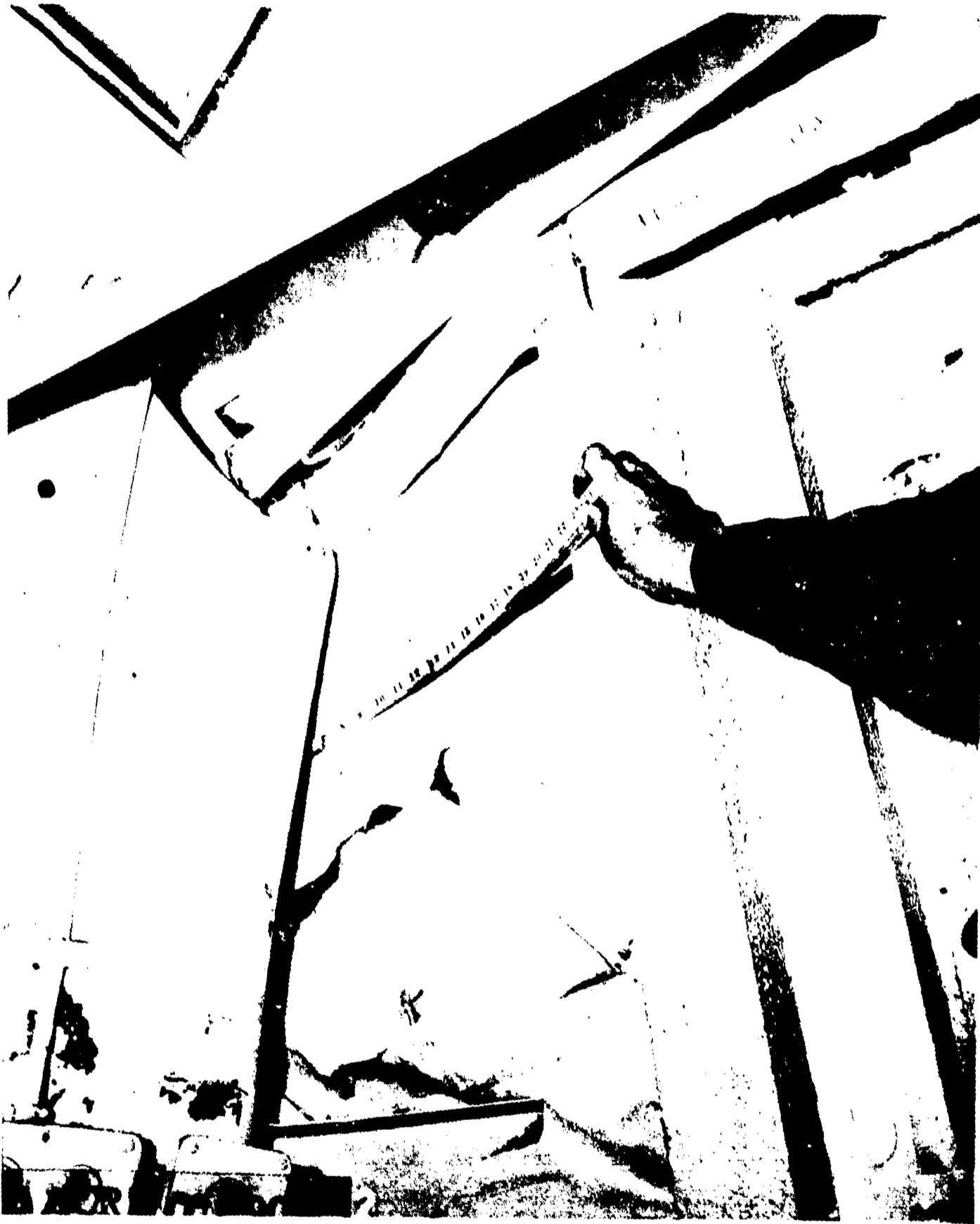
AA-CR-80-1906-2. Damage at port forward corner of captains pantry, superstructure deck.
