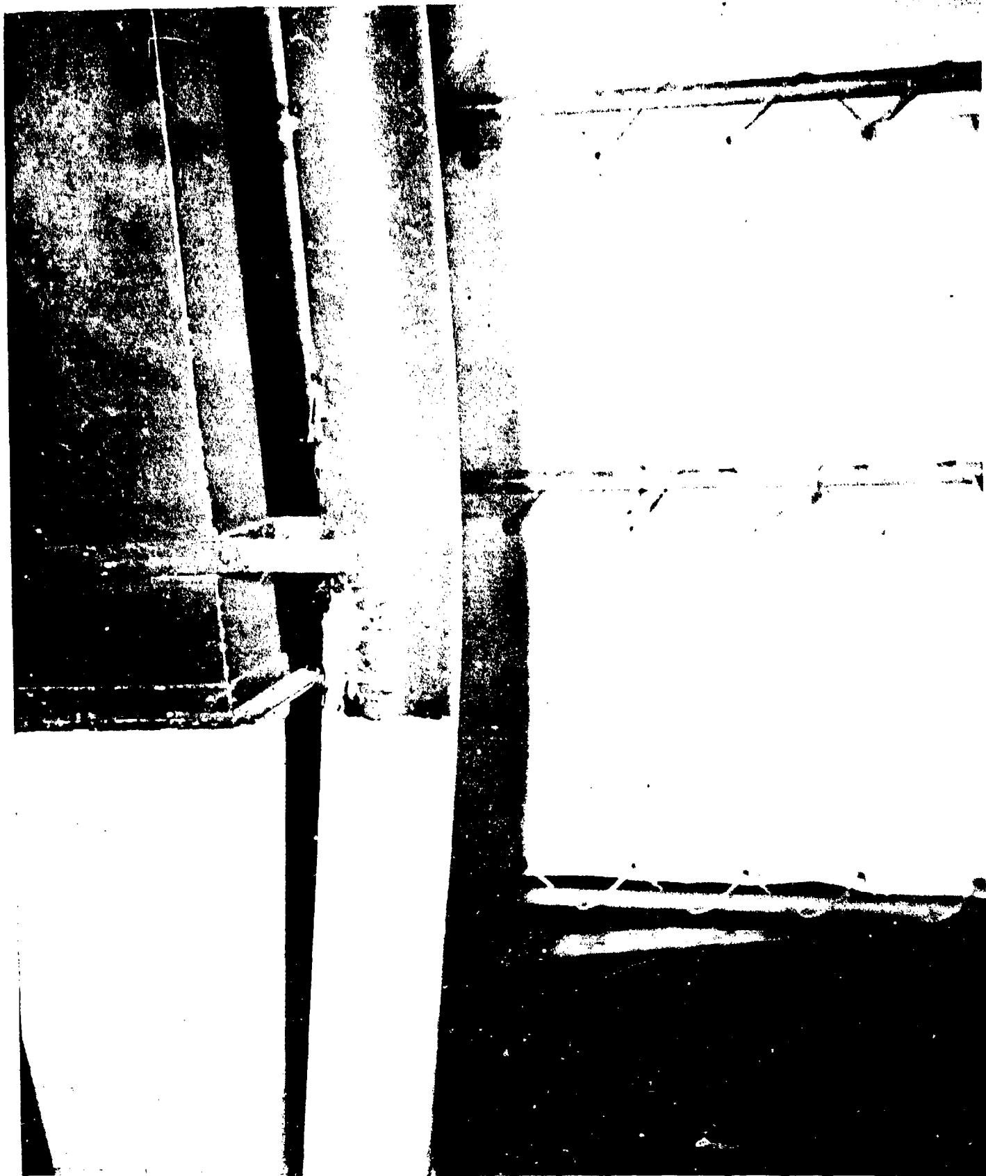
AA-CR-80-1908-9. Looking to port on main deck in after troop berthing space showing deflection of port stanchion at frame 129.
