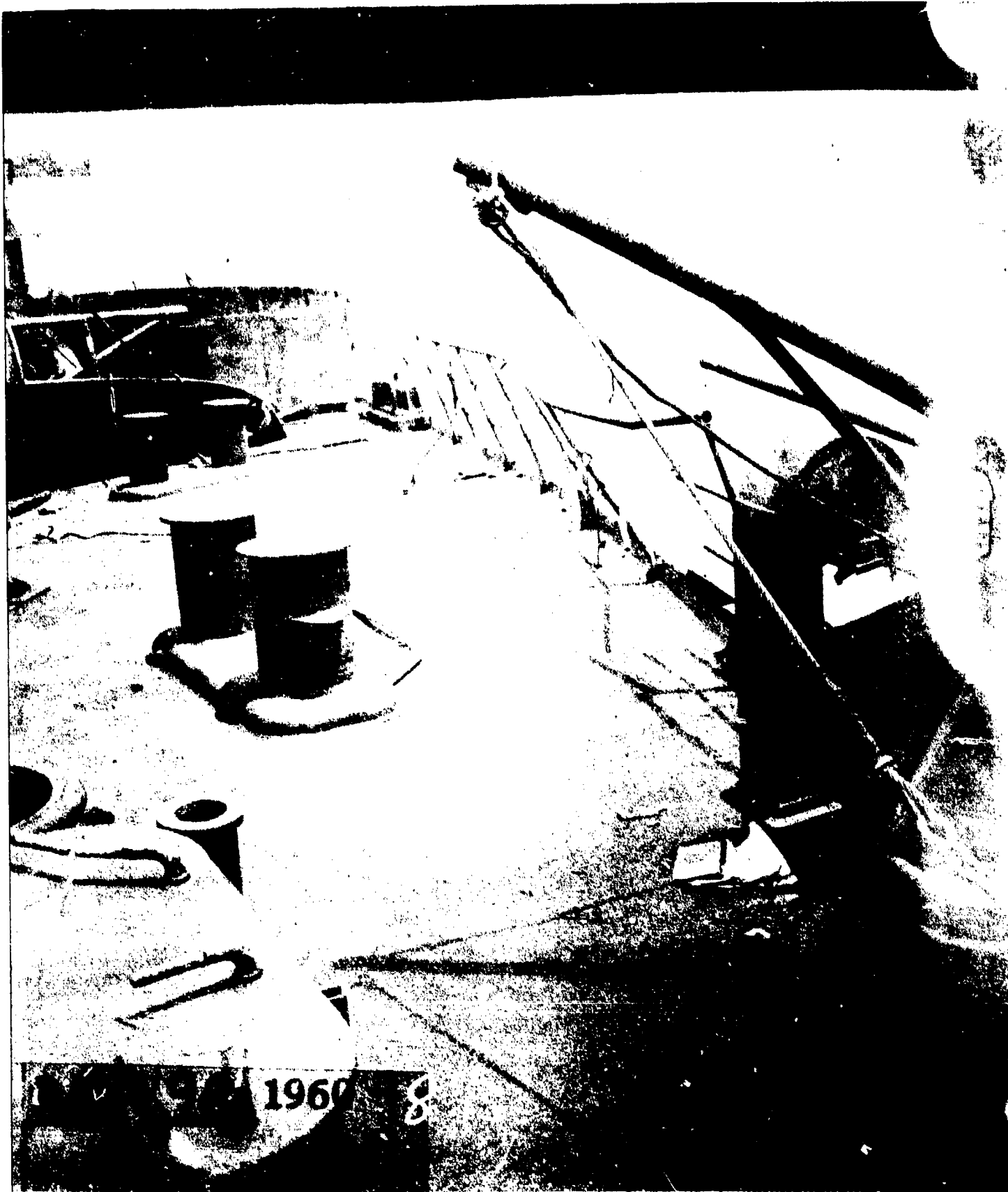
AA-CR-98-1960-8. Looking aft on upper deck, port, from bow, showing damaged railing.
