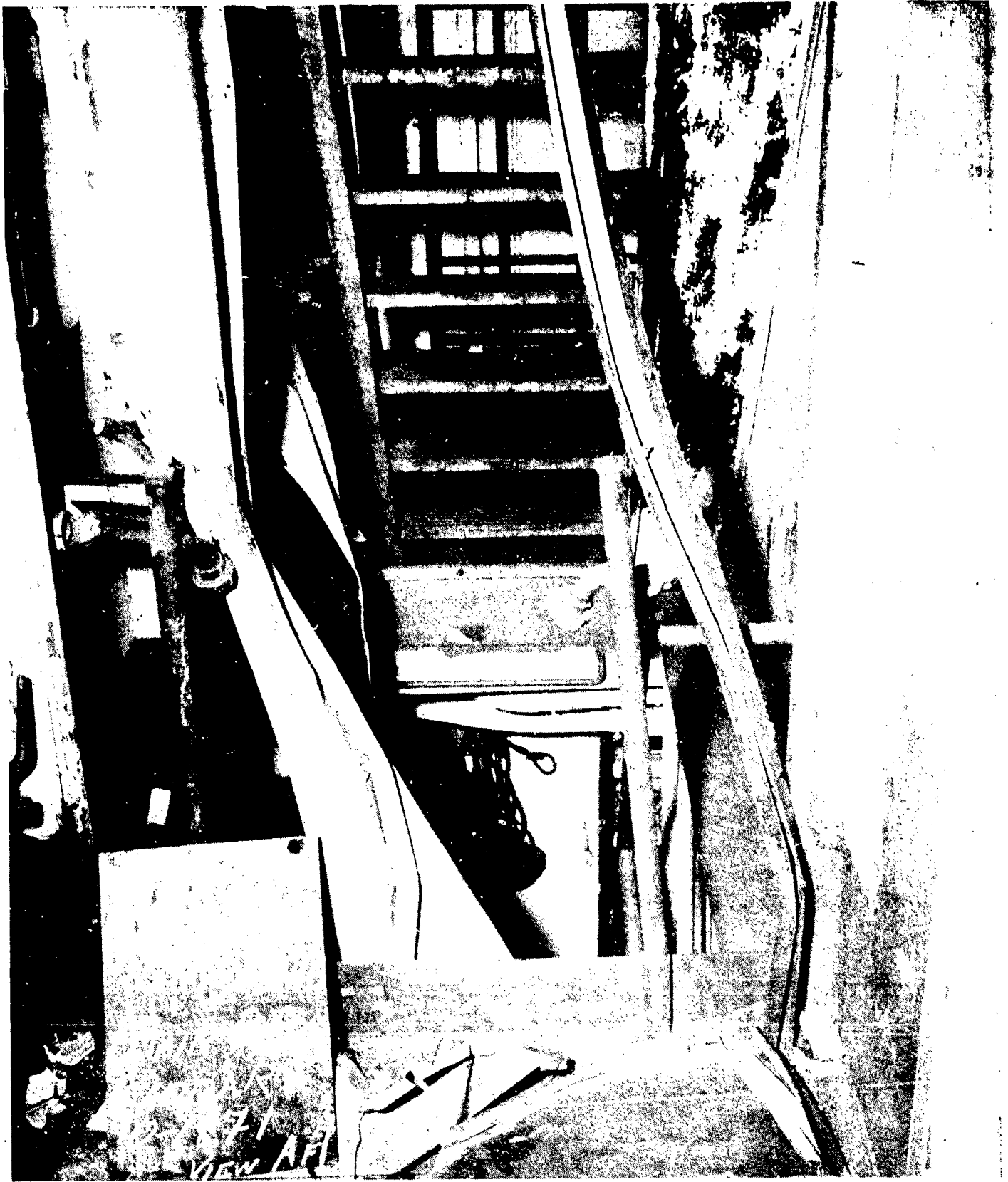
AA-CR-82-1828-12. Main deck, frame 87, starboard. Damage to metal joiner, light lock around ladder 1-87-1.
