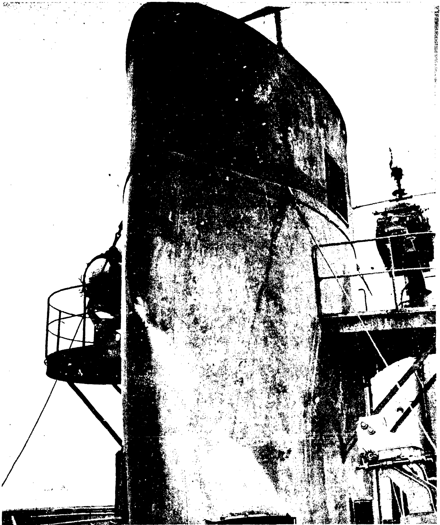
AA-CR-62-2172-12. Looking forward and to port at starboard side of forward stack. Note damaged yoke of starboard 24 inch searchlight.
