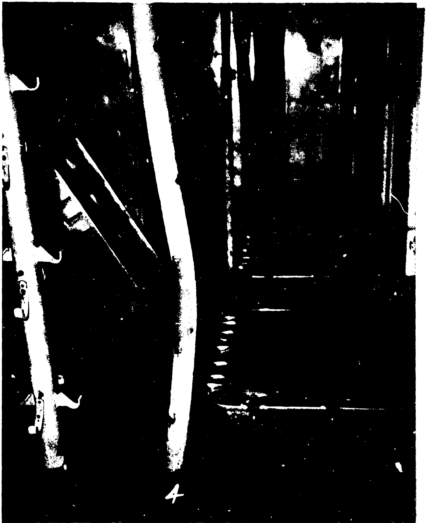
AA-CR-80-1898-4. C-204L. Buckled stanchions at frame 175 between main deck and first platform. Looking to port in crews quarters.
