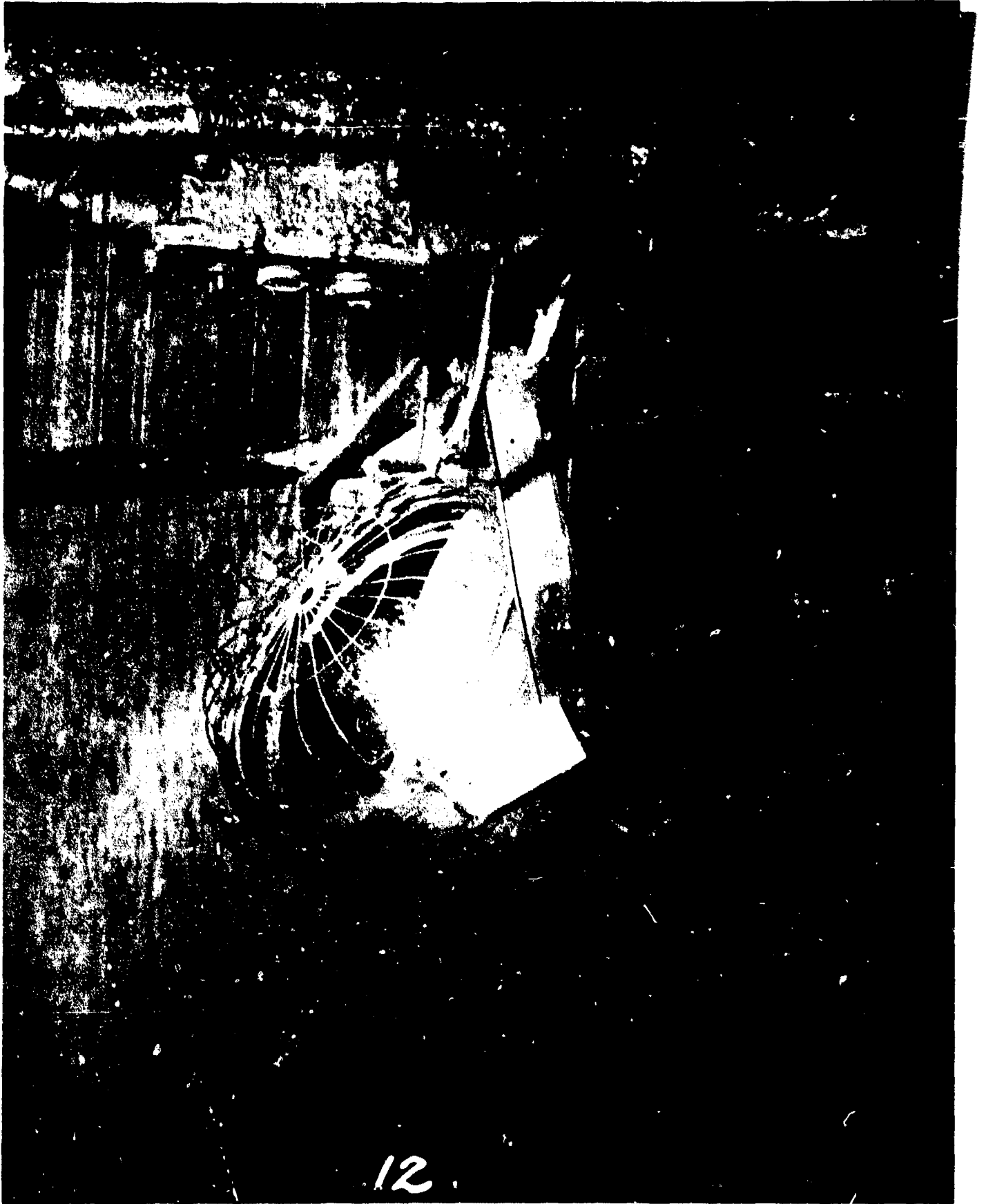
AA-CR-82-1830-12. Floodlight mounted on the starboard side of superstructure deck at frame 69. Shows damage to the floodlight. Picture taken looking to starboard.
