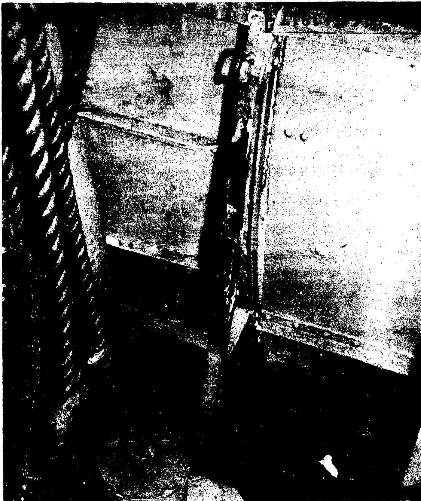
AA-CR-65-1817-3. View of bulwark showing distorted plating and stiffener and charred paint.
