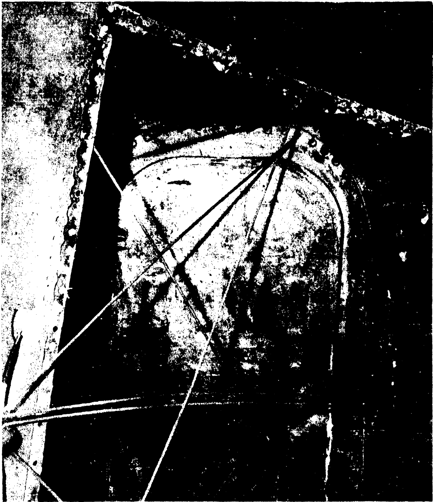
AA-CR-65-1817-4. View showing ruptured aluminum bulkhead in way of CIC door.
