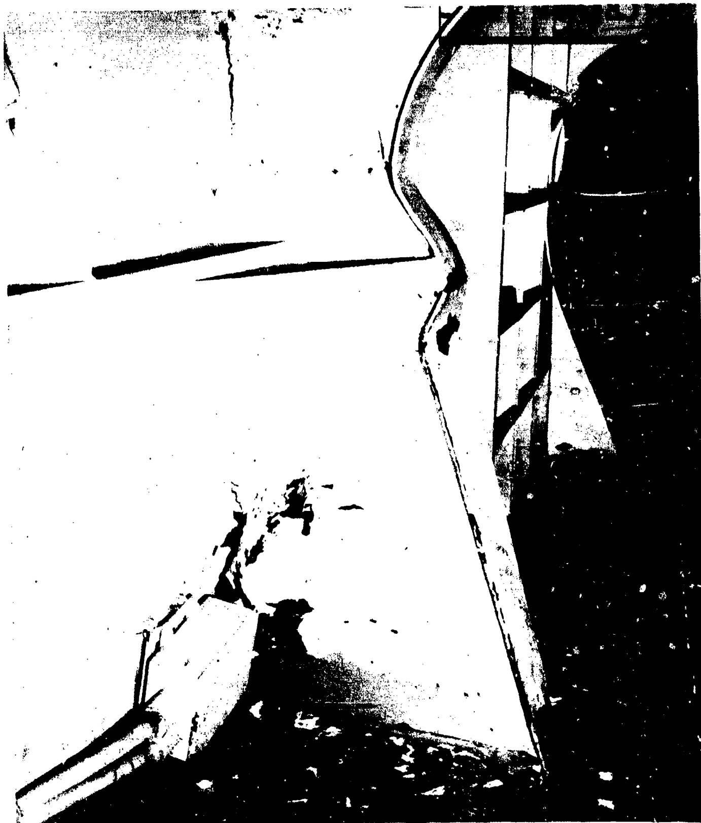
AB-CR-66-146-4. After Baker. Third deck, C-301-L. Crews messing, showing failure of weld joining web of frame 110 to 3rd deck. Port side, looking outboard and forward.
