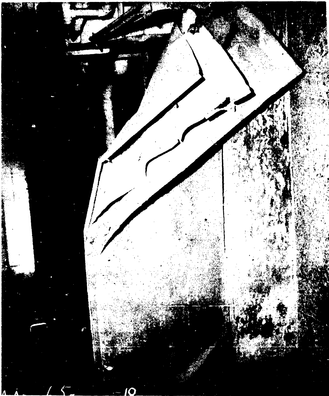
AA-CR-65-1735-10. Second deck, B-201-1L. Buckling of ventilation intake port side, frame 63, looking forward.
