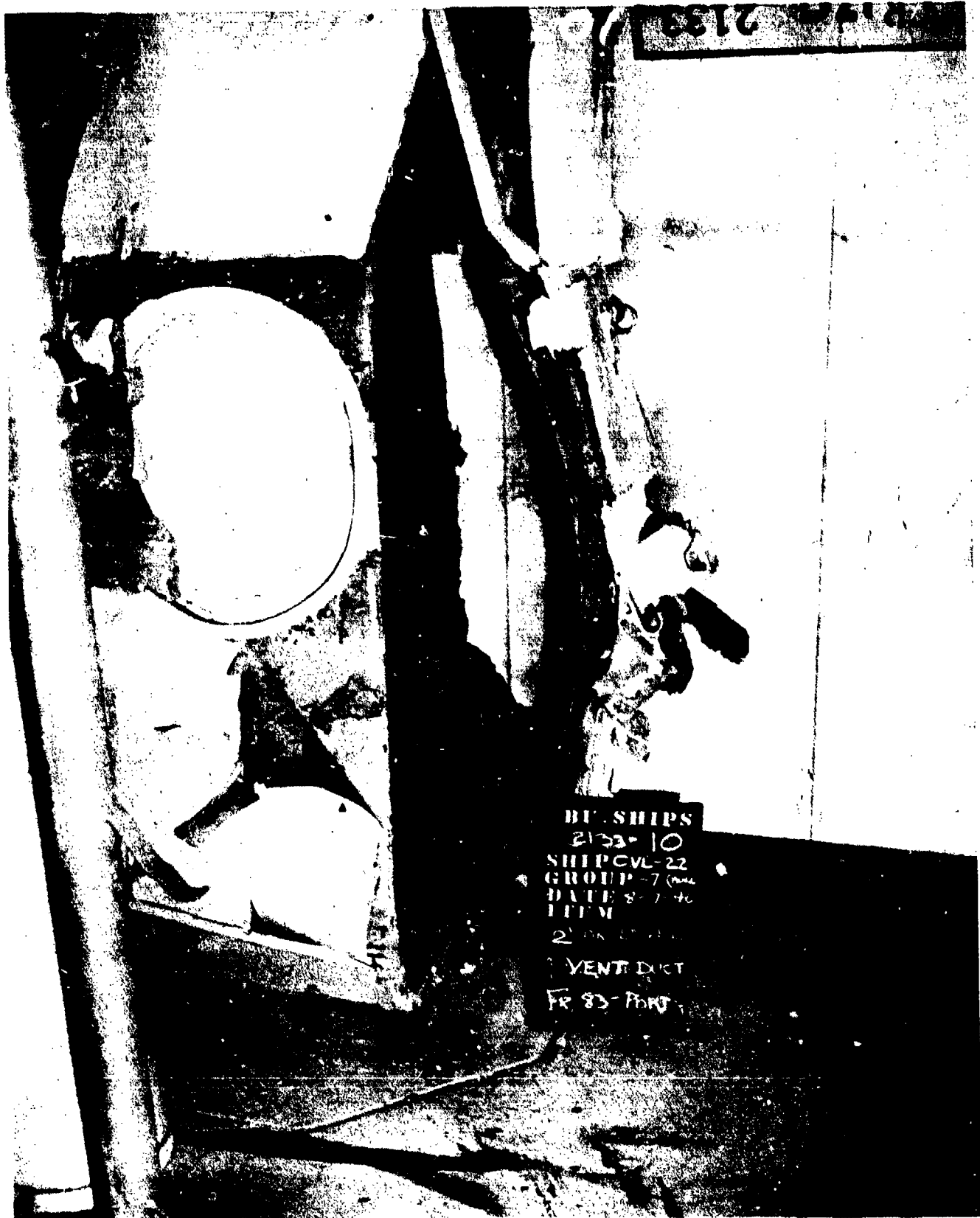
AA-CR-175-2133-10. Second deck, B-203-L. Blast damage to arc welded ventilation duct in mess attendants berthing space on port side at frame 83. Looking inboard and aft.
