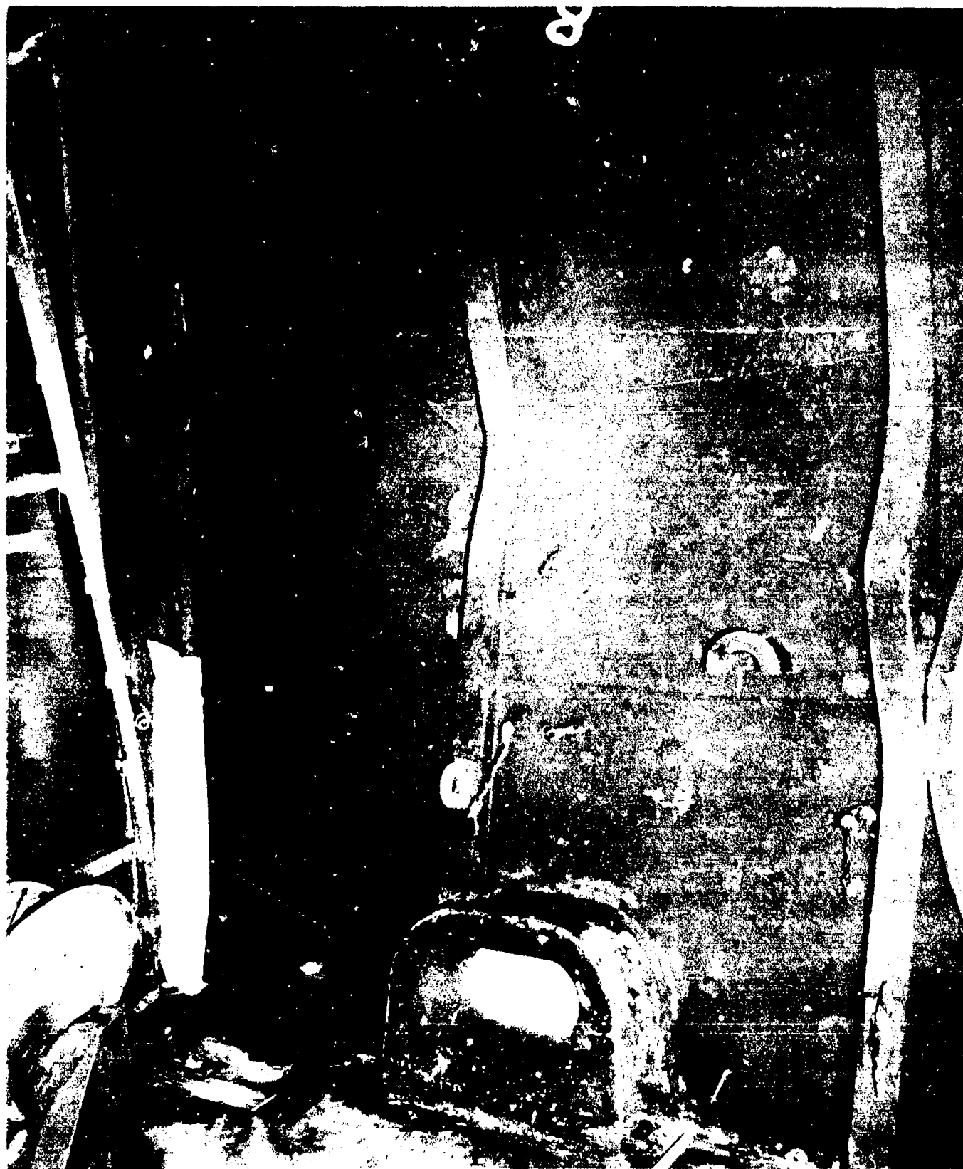
AB-CR-66-146-8. After Baker. Main deck, starboard side, frames 144 to 146, showing failure of welded connection between upper end of stiffeners and overhead poop deck structure; and, failure of welded joint between bulkhead 144 and side plating. Looking outboard and forward.
