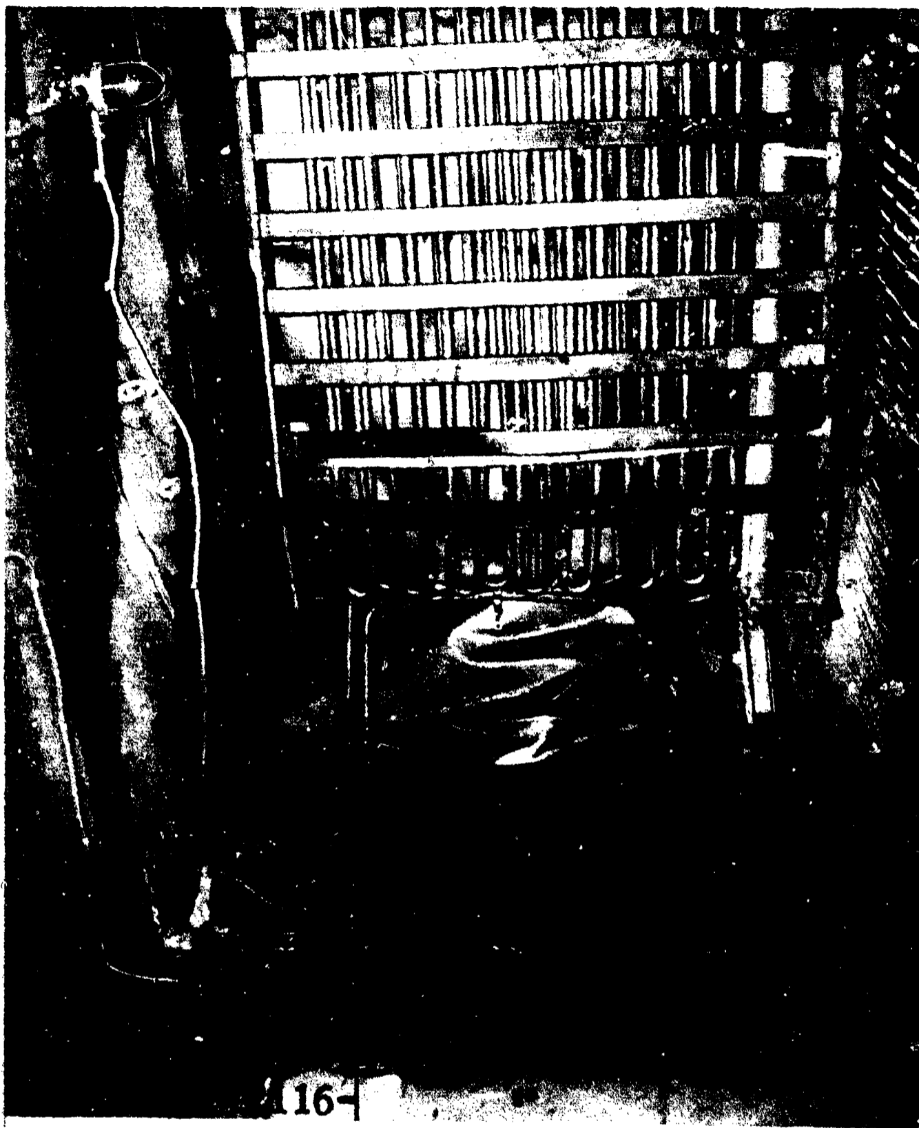
AA-CR-175-2116-3. Third deck. C-308-1A. Looking to port and aft from frame 120. Port corner of bulkhead 123 just visible between columns in left side of picture.
