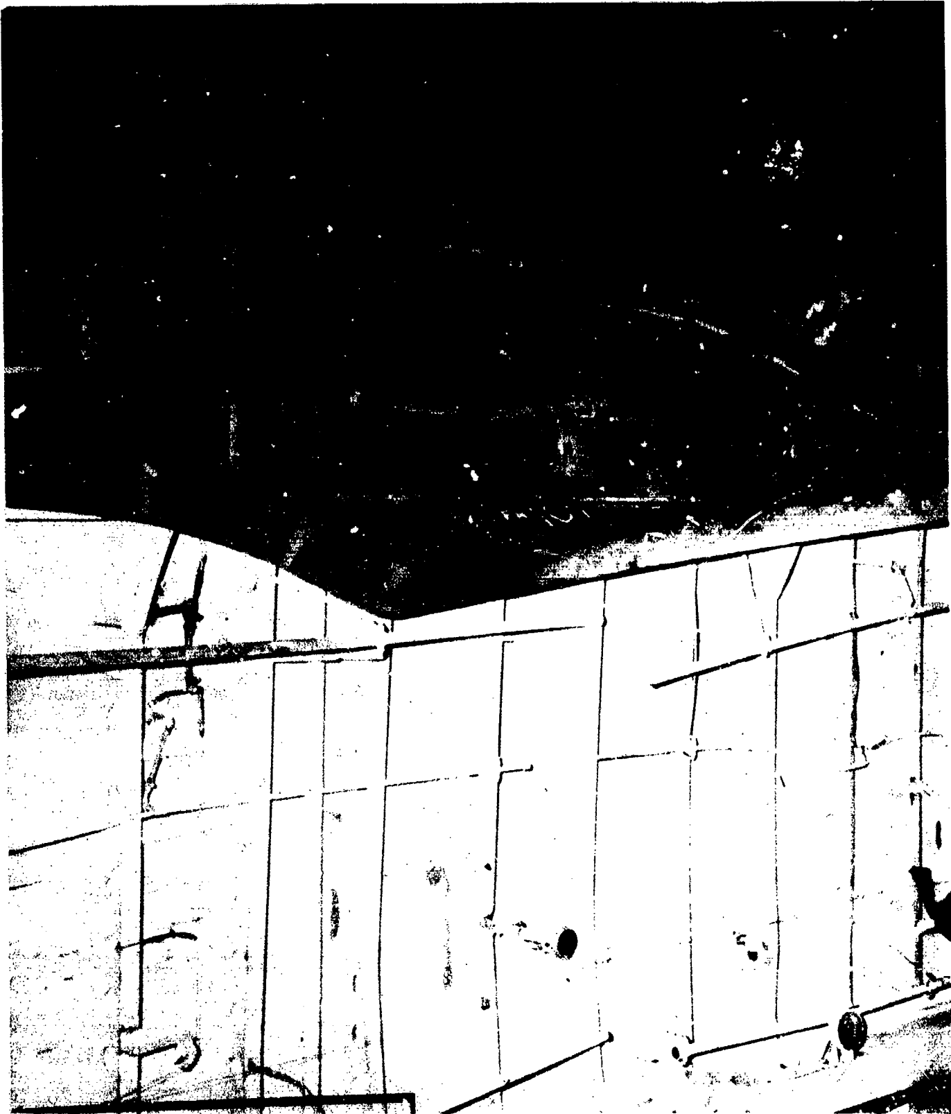
AA-CR-59-4151-7. Flight deck bent girder 107, looking up and to starboard.
