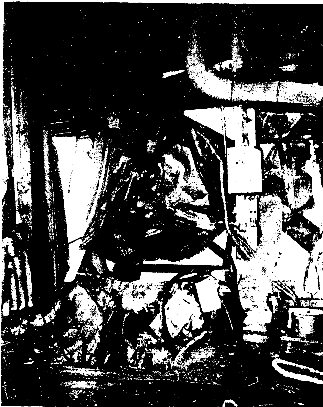
AA-CR-62-1880-2. #1 Uptake between hangar and flight deck.
