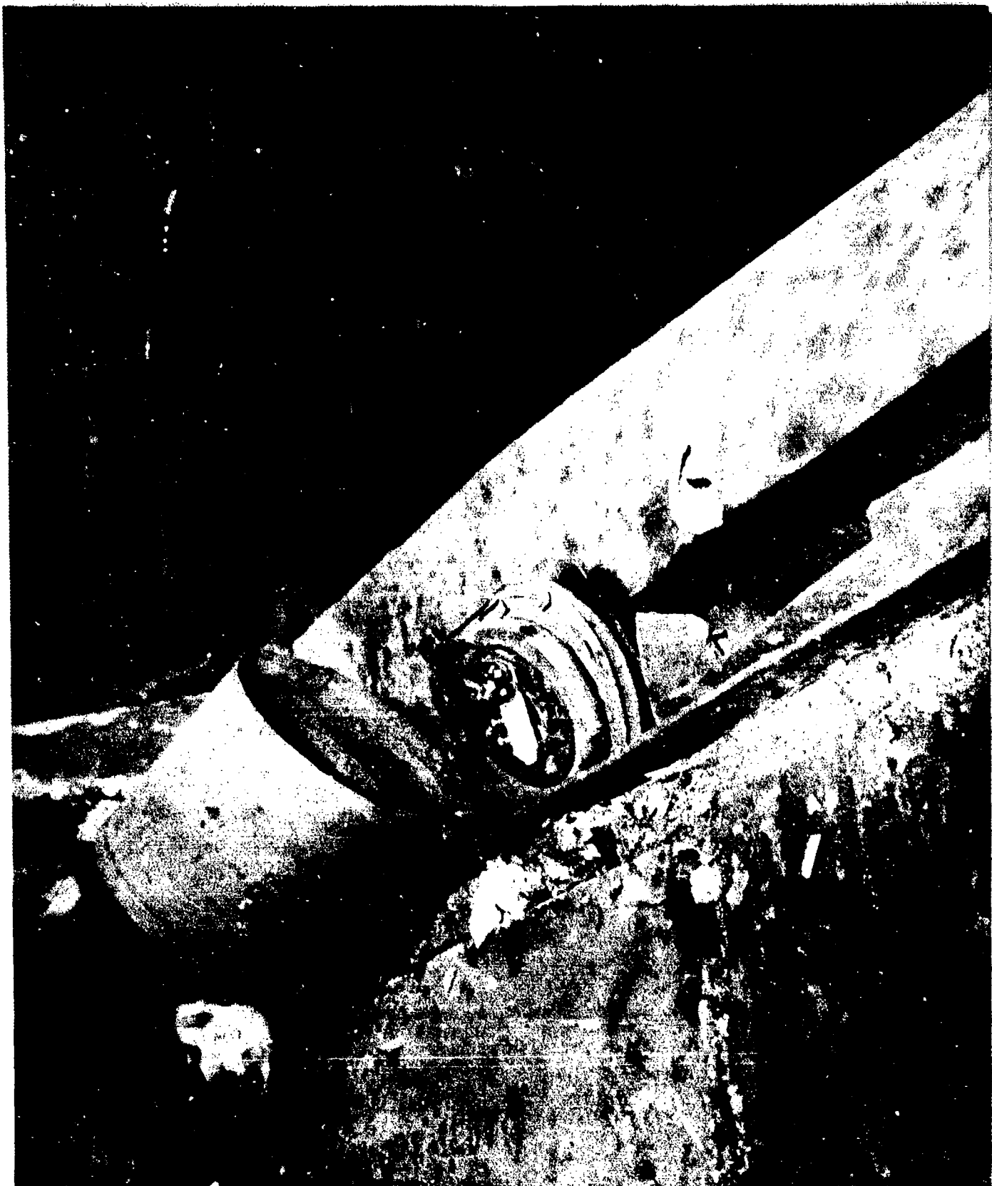
AA-CR-62-1881-4. Damage to deck edge landing light of frame 84 port side of flight deck, view looking aft and outboard.
