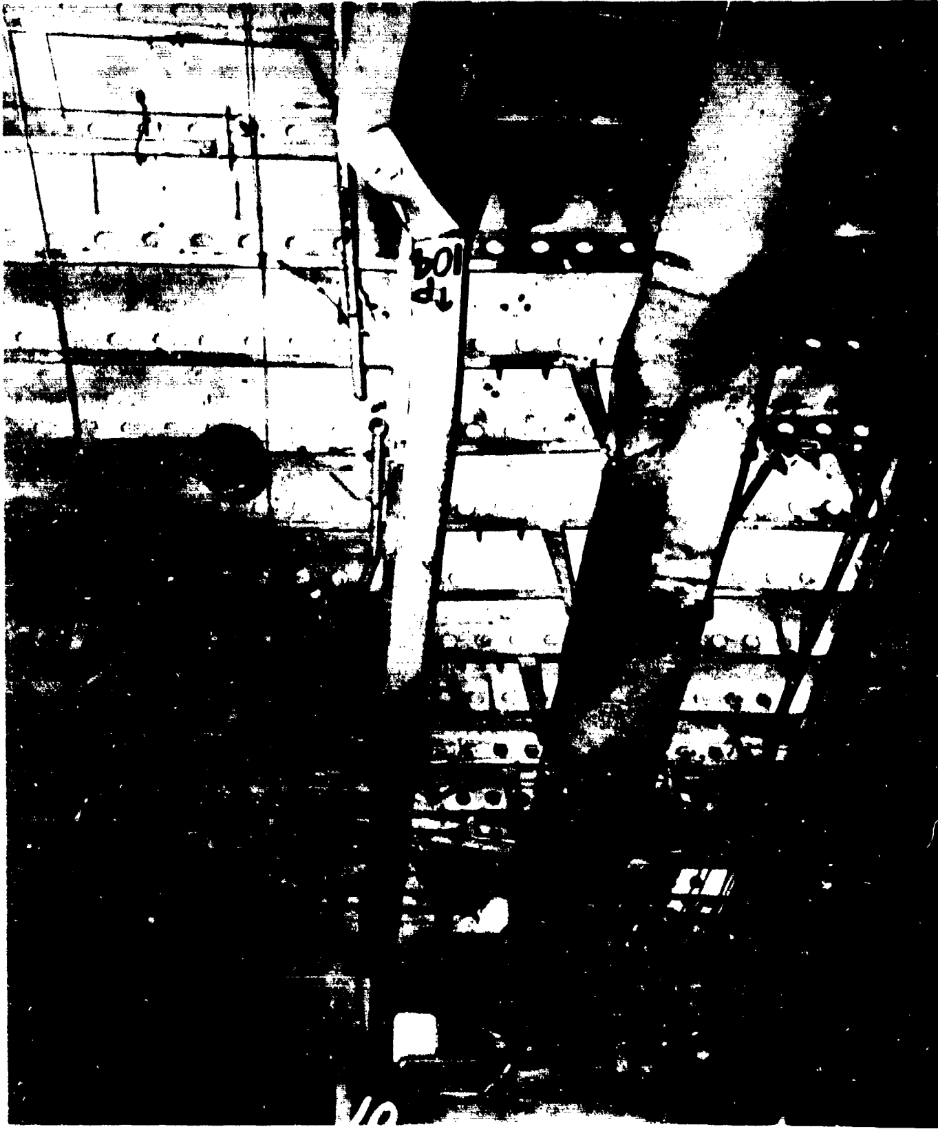
AA-CR-100-4161-10. Underside of flight deck, looking to port, showing deformation of bent girders 104 at centerline.
