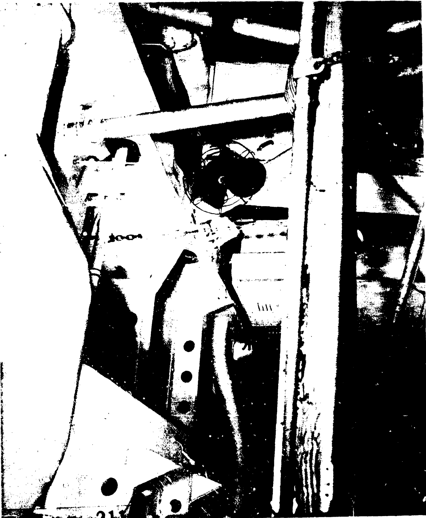
AA-CR-175-211b-8. Second deck, C-201-L, looking to starboard at frame 108.
