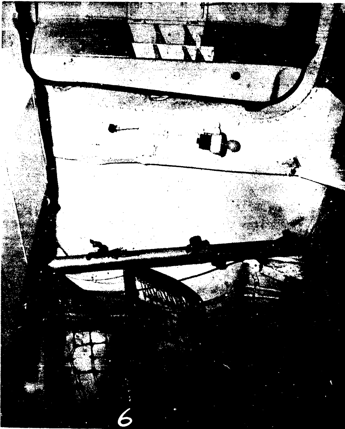
AA-CR-175-2117- 6. Third deck. C-310-L. Aft face of bulkhead 132, port side.
