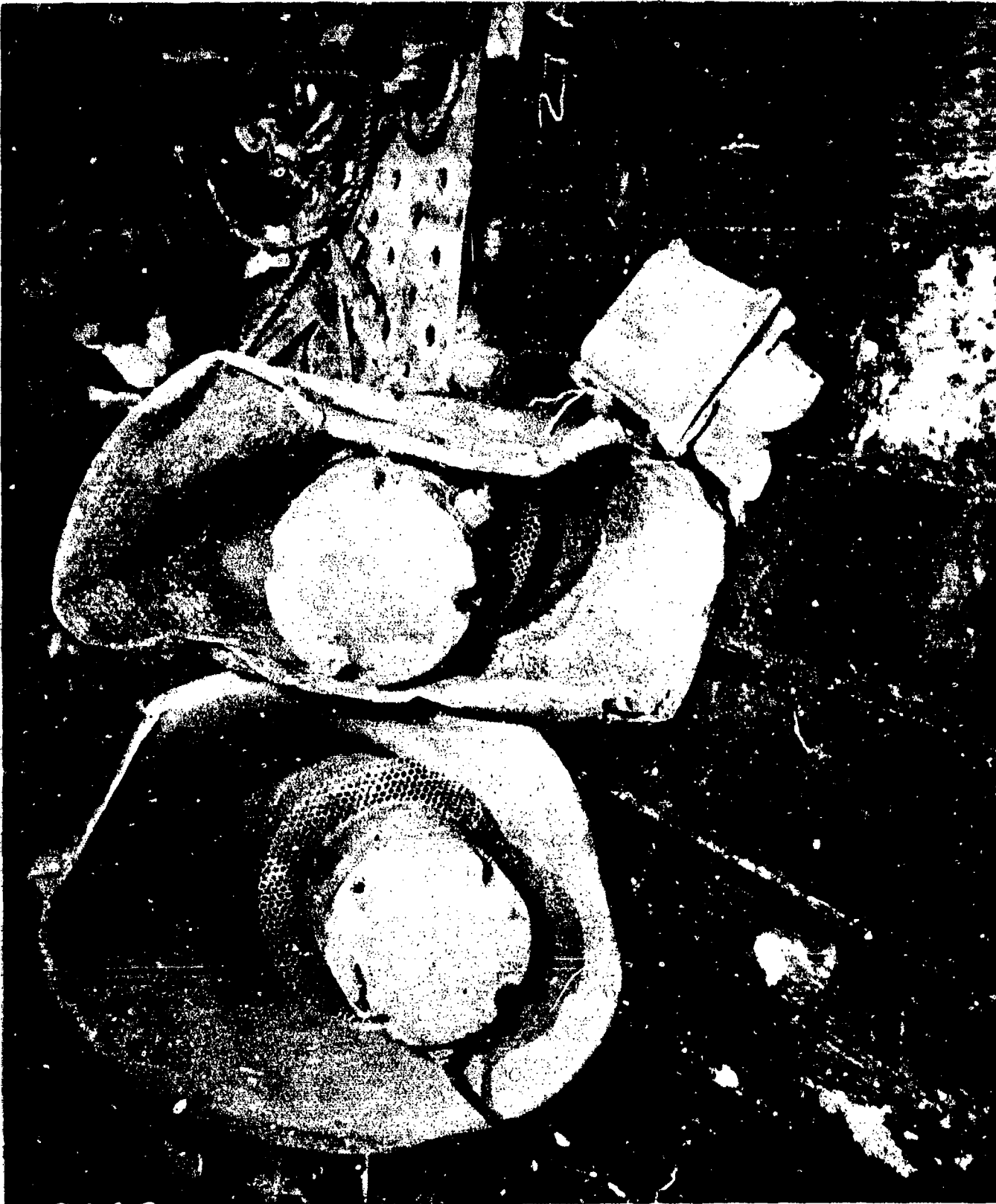
AA-CR-62-1880-10. Two 3MC reproducers laying on flight deck, which were broken loose from foundations on port bulkhead island structure above flight deck, overlooking and down to starboard.
