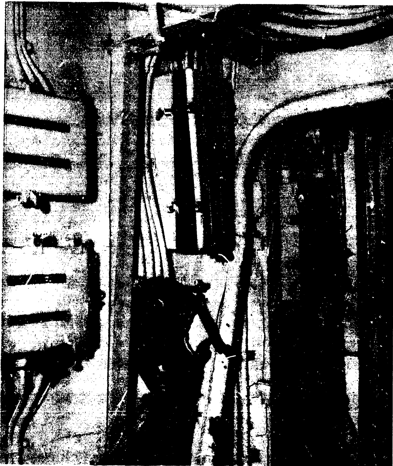
AA-CR-234-1989-8. A 4x and 12x lighting distribution box, frame 54 in flight deck control station. Enclosures damaged by inboard deflection of bulkhead.
