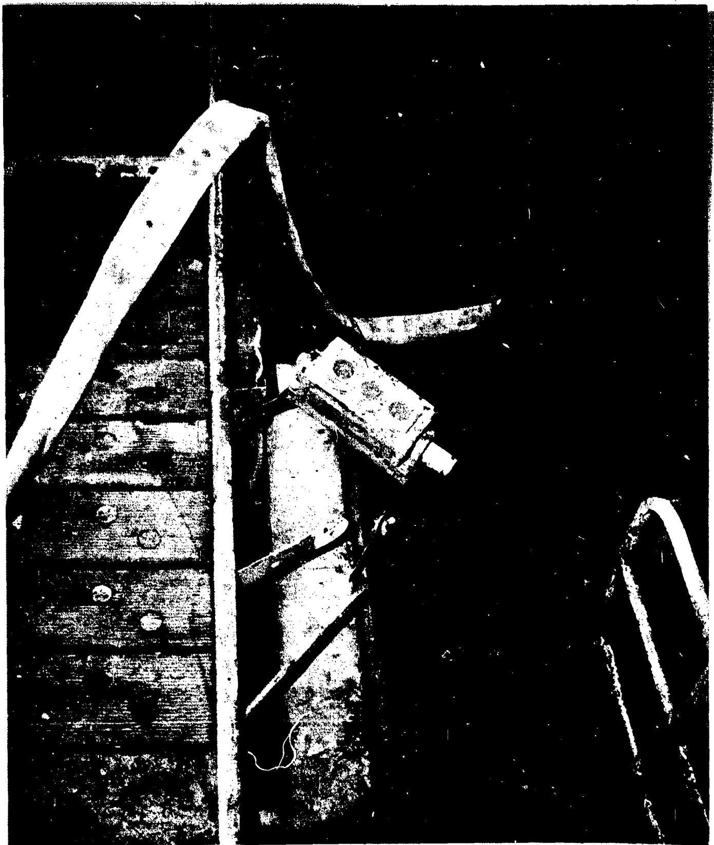
AA-CR-82-1920-9. Catapult ready light indicator frame 22 starboard side flight deck plastic lens damaged by radiant heat of bomb and foundation bracket broken.
