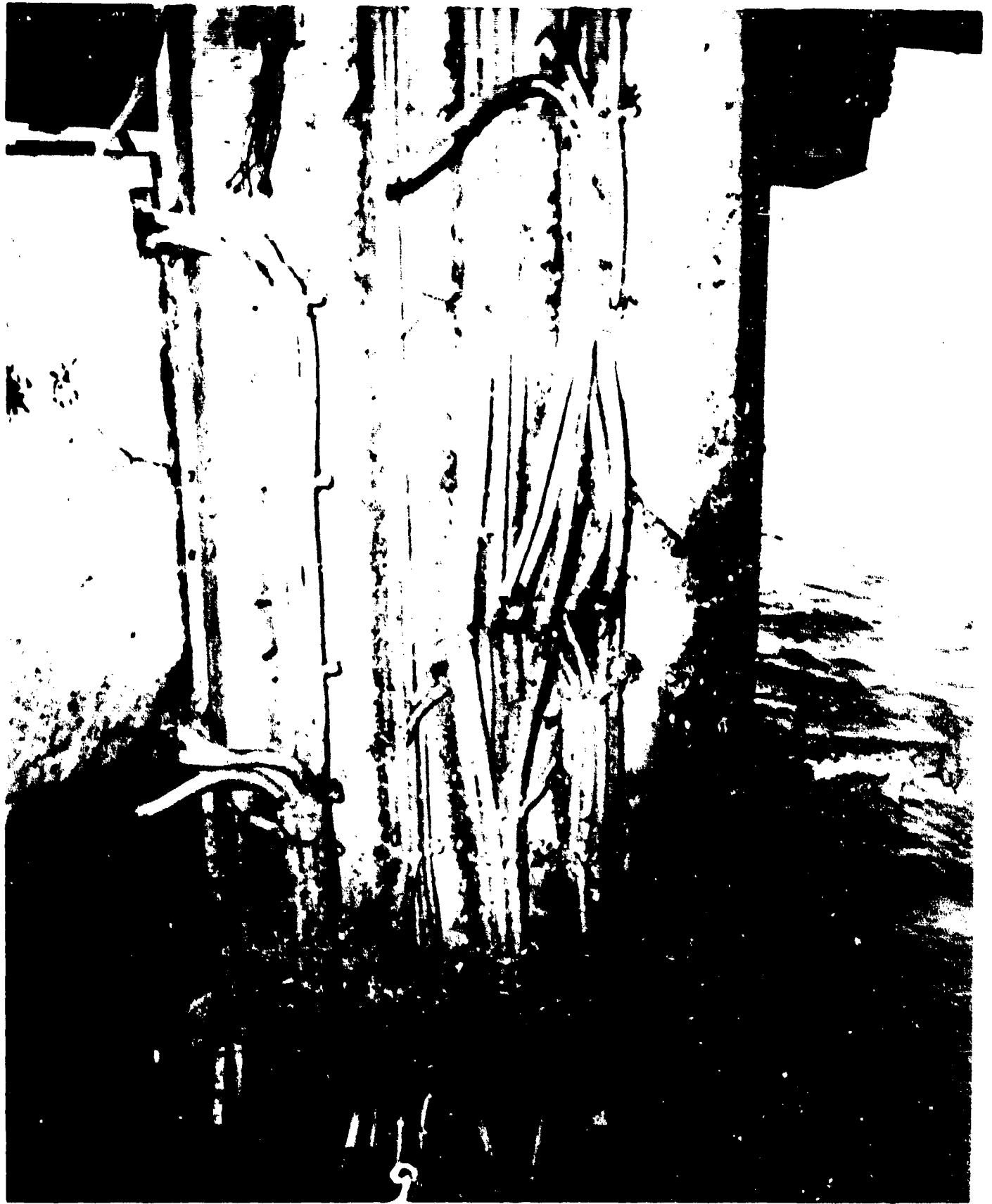
AA-CR-82-1917-9. Vertical wireway through hangar deck frame 92 port side hangar space cable damage due to deflection of bulkhead inboard. View looking aft.
