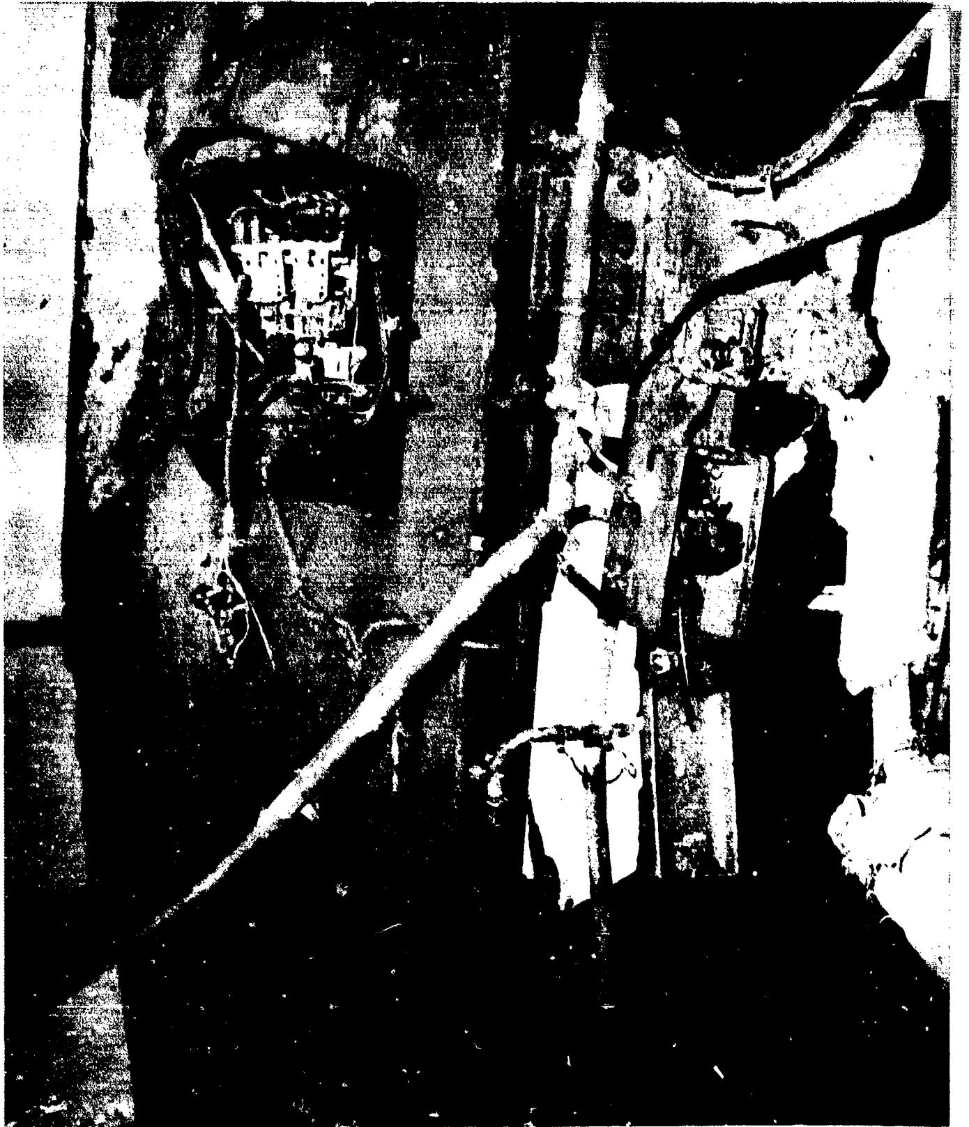
AA-CR-82-1918-6. Damage to ventilation controller and type "C" automatic telephone unit, located at frame 113 starboard side hangar space. View looking aft and outboard.
