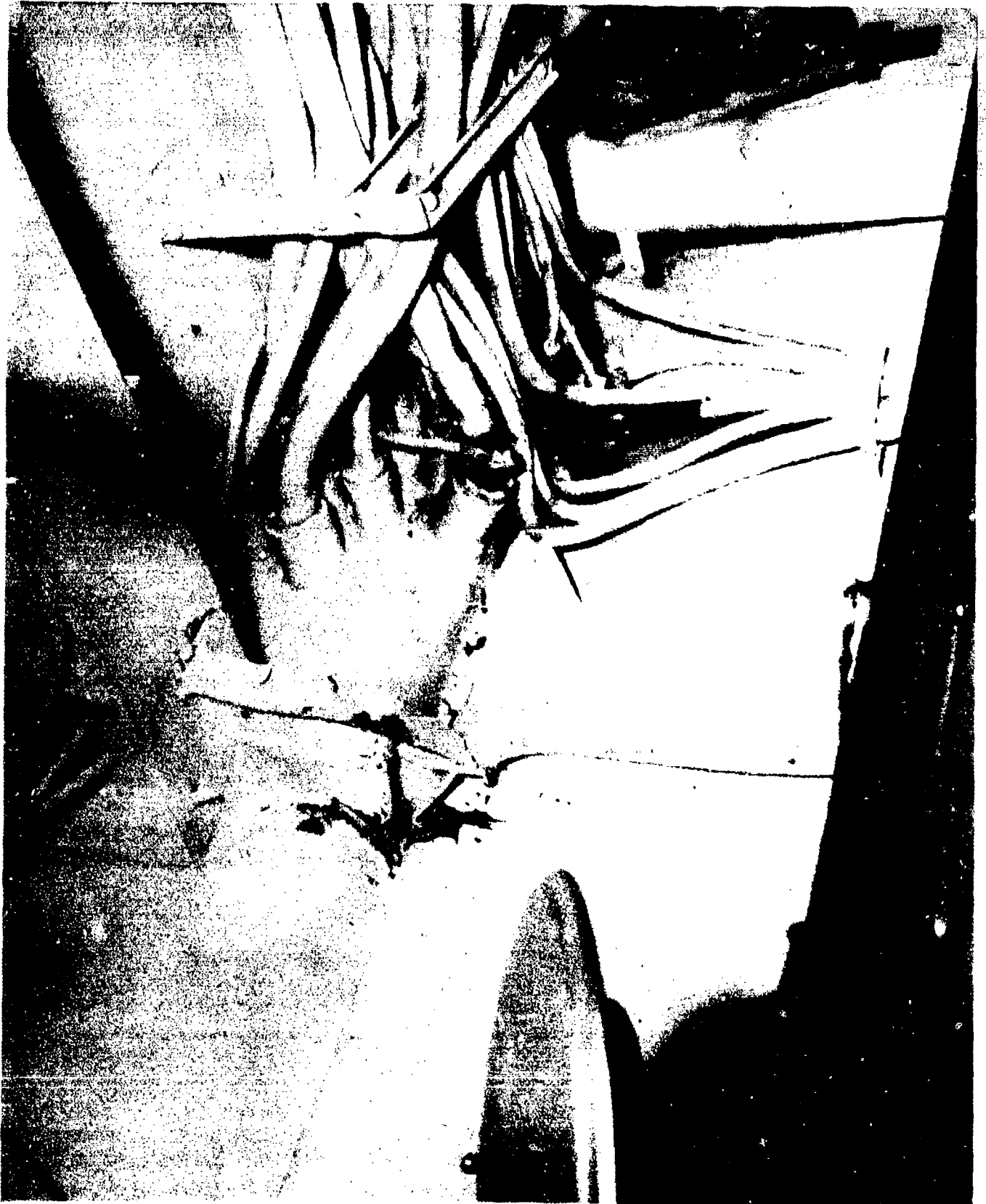
AA-CR-82-1916-3. Stuffing tube area through bulkhead 49 port side, second deck, break in cable due to deflection of tube area, view looking up and forward.
