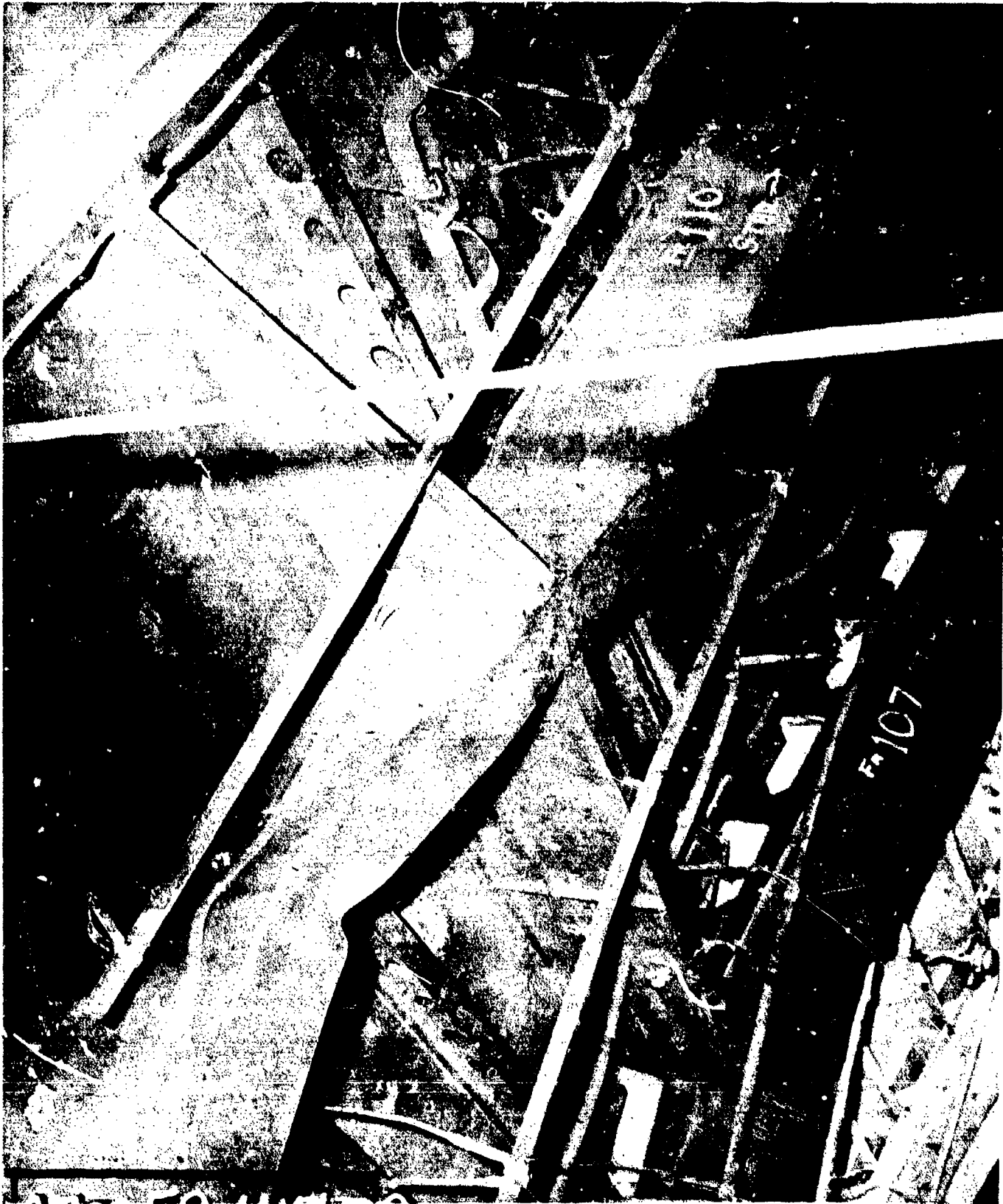
AA-CR-59-4151-9. Flight deck bent girders 104, 107 and 110, showing failures near centerline. Looking forward and to starboard.
