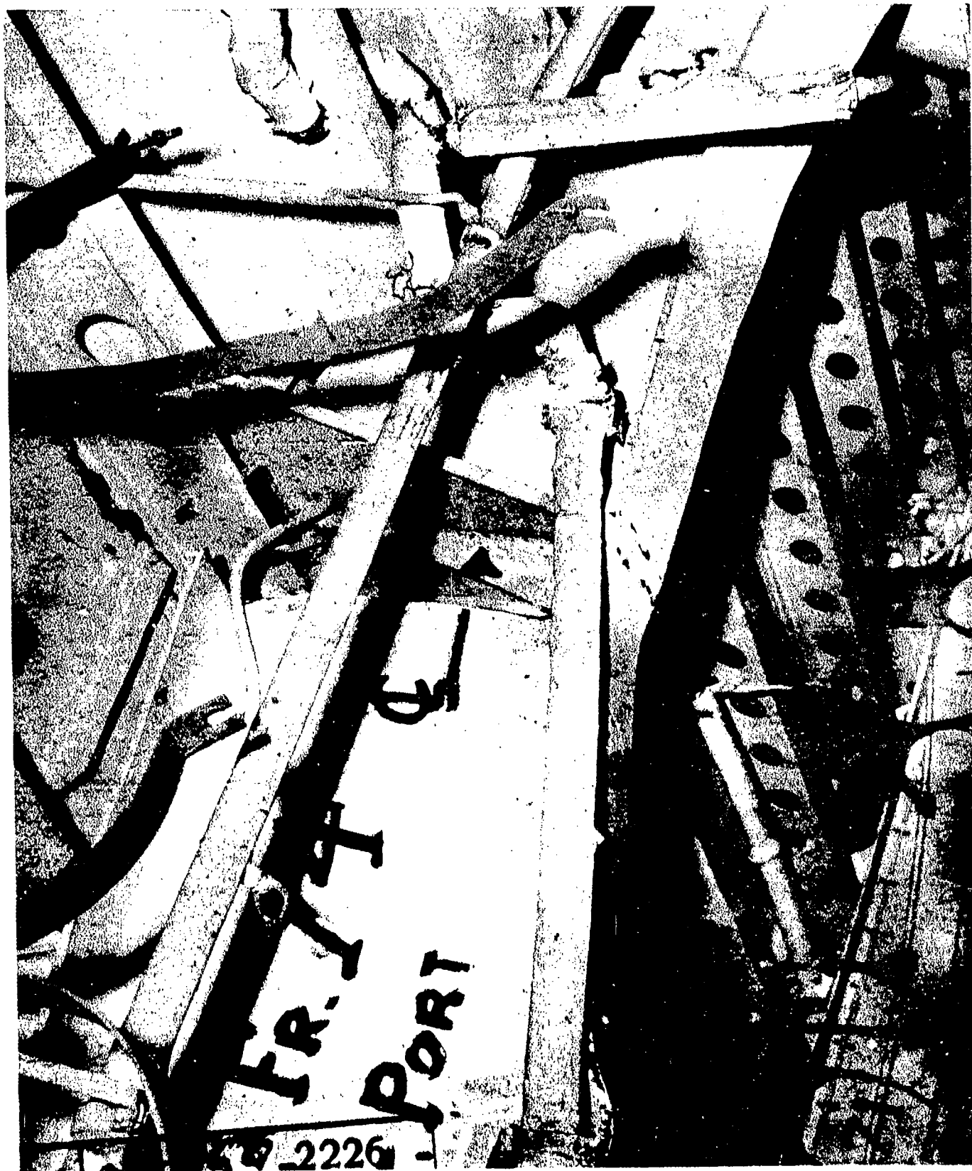
AA-CR-59-2226-9. Flight deck Bent 74, looking forward, showing tear in girder to port of centerline.
