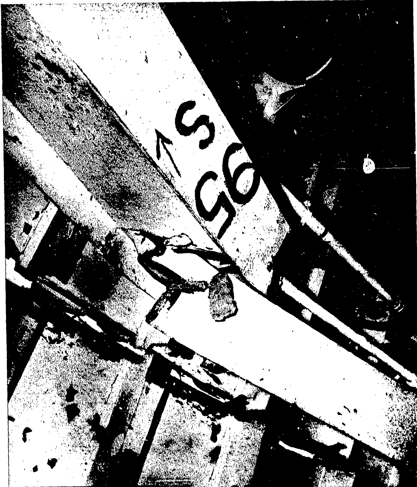
AA-CR-59-4151-3. Flight deck Bent 95, looking to port at centerline break. Note transverse tear in flight deck.
