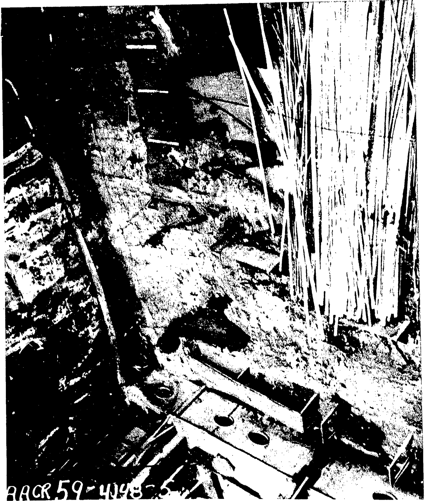
AA-CR-59-4148-5. After elevator pit looking aft and starboard from forward port corner of opening in flight deck.
