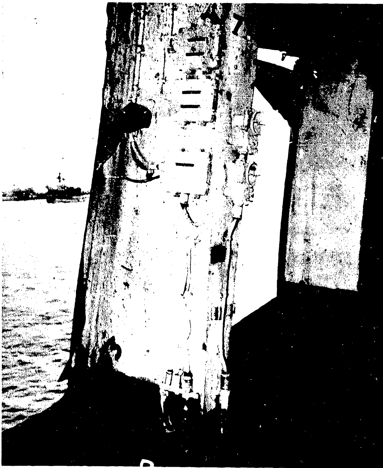
AA-CR-80-4186-8. After Baker - Flight deck Bent 77, port bottom, looking forward.
