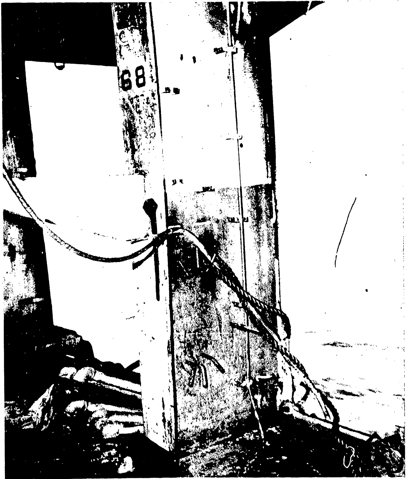
AA-CR-80-4186-3. After Baker - Flight deck Bent 68, port bottom, looking aft.
