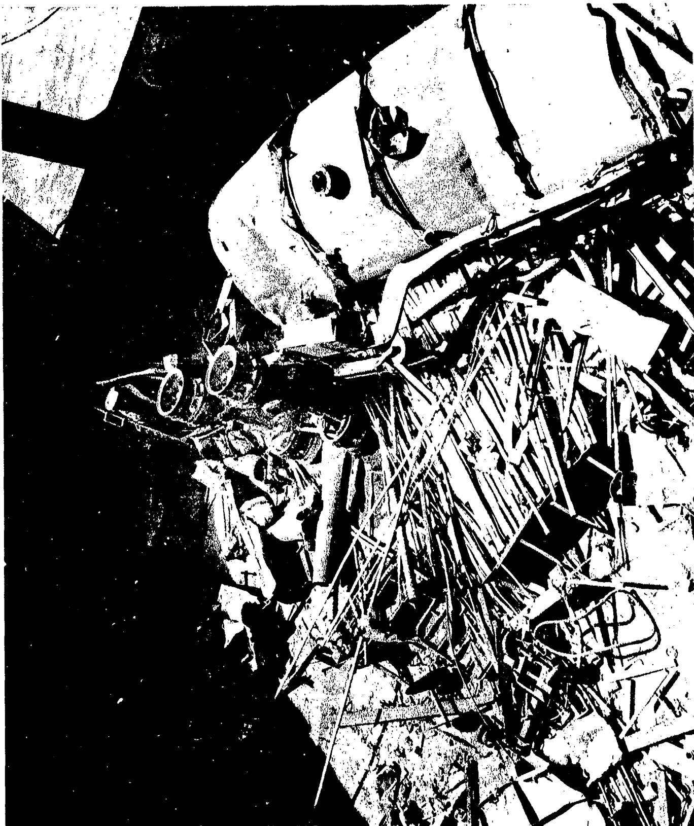
AA-CR-175-2038-9. After elevator pit, looking aft and to port. Note demolished water filled trailer and stack of pipe.
