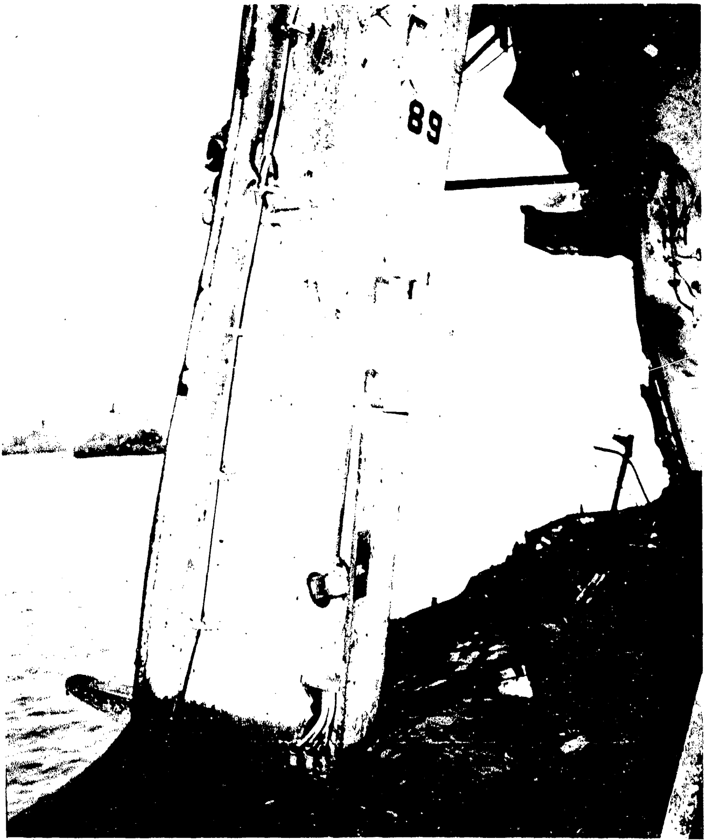
AB-CR-80-4187-6. After Baker. Flight deck Bent 89, port bottom, looking forward.
