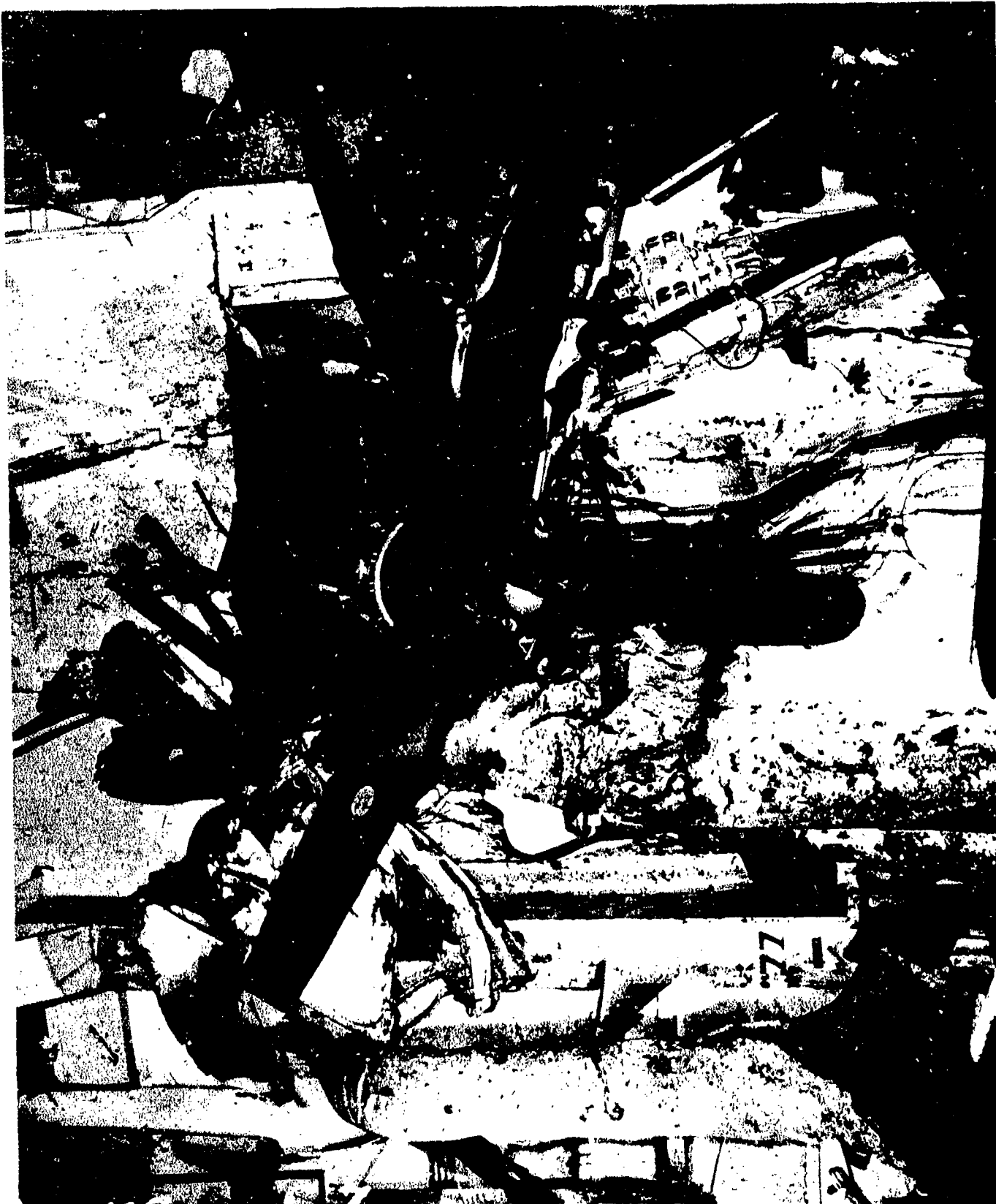
AA-CR-175-2039-7. General view in vicinity of flight deck Bent 77-80, starboard side. Airplane engine blown into intake plating.
