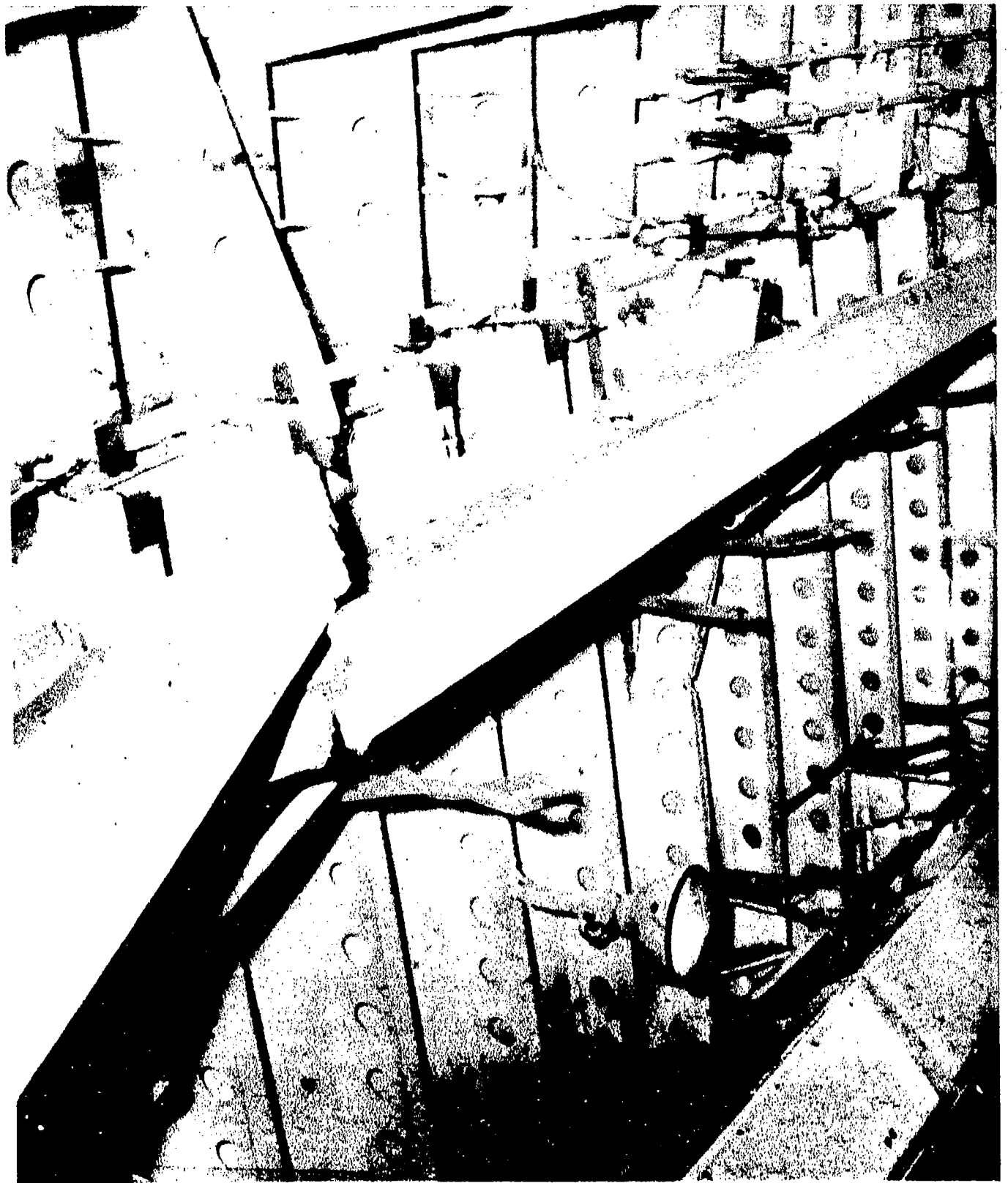
AA-CR-59-2225-1. Flight deck and Bent 95, showing tear in deck and failure of transverse girder at welded centerline butt. Looking to starboard.
