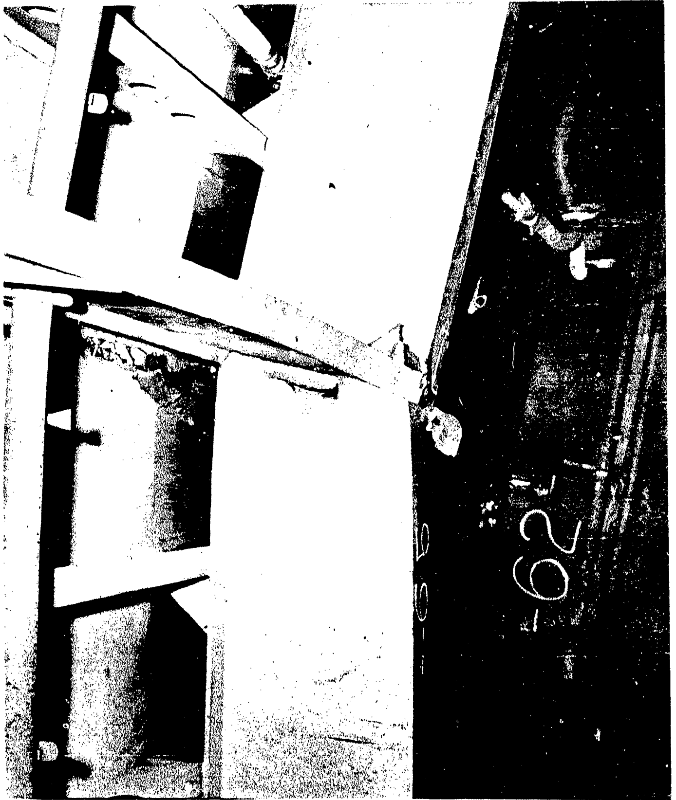
AA-CR-59-2222-2. Flight deck Bent 65, centerline, looking forward. Note joint failure and tear in flight deck plating.
