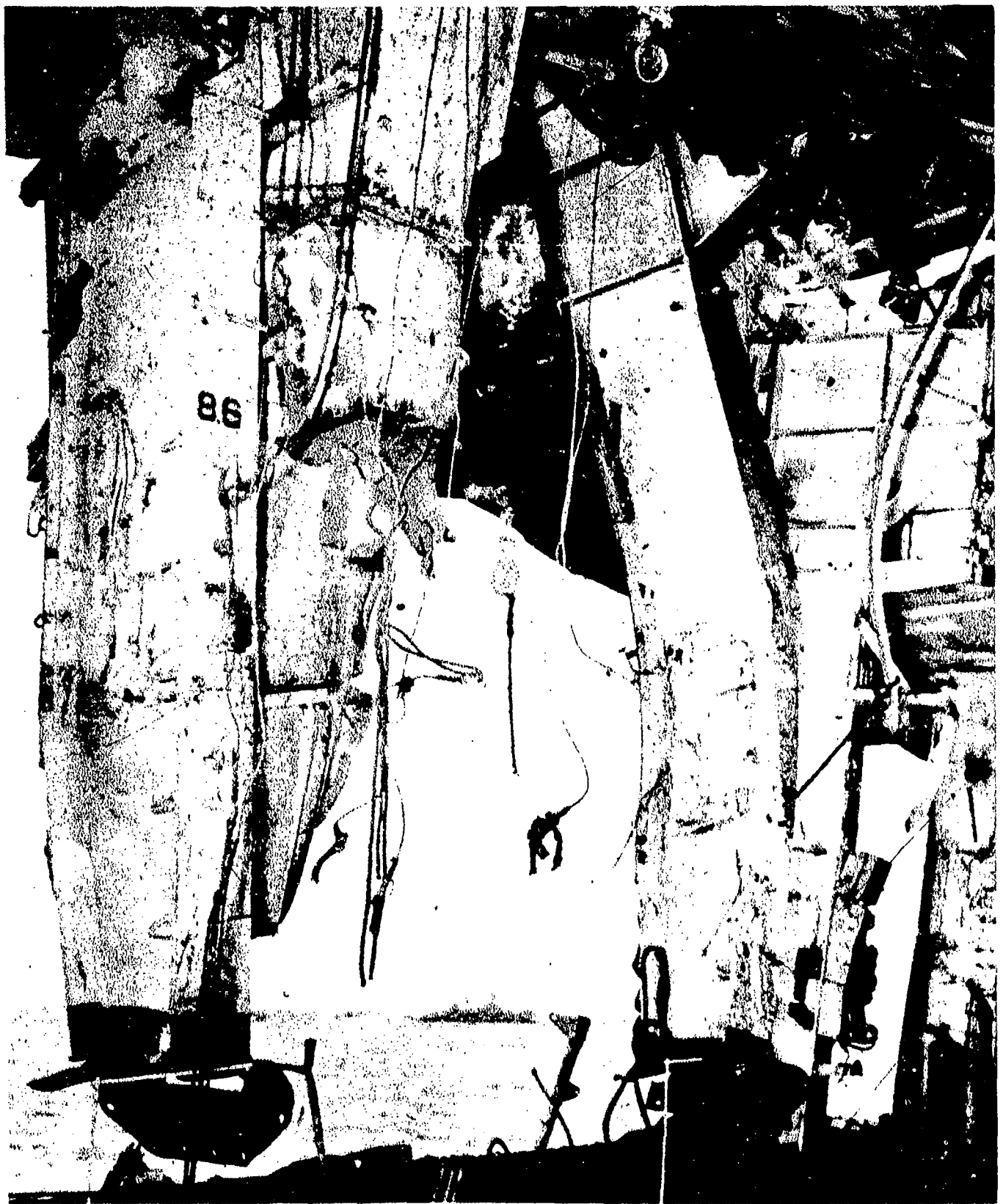
AA-CR-175-2131-5. Hangar. Wobble Bents 83 and 86, port side. Looking forward and outboard from bent 89.
