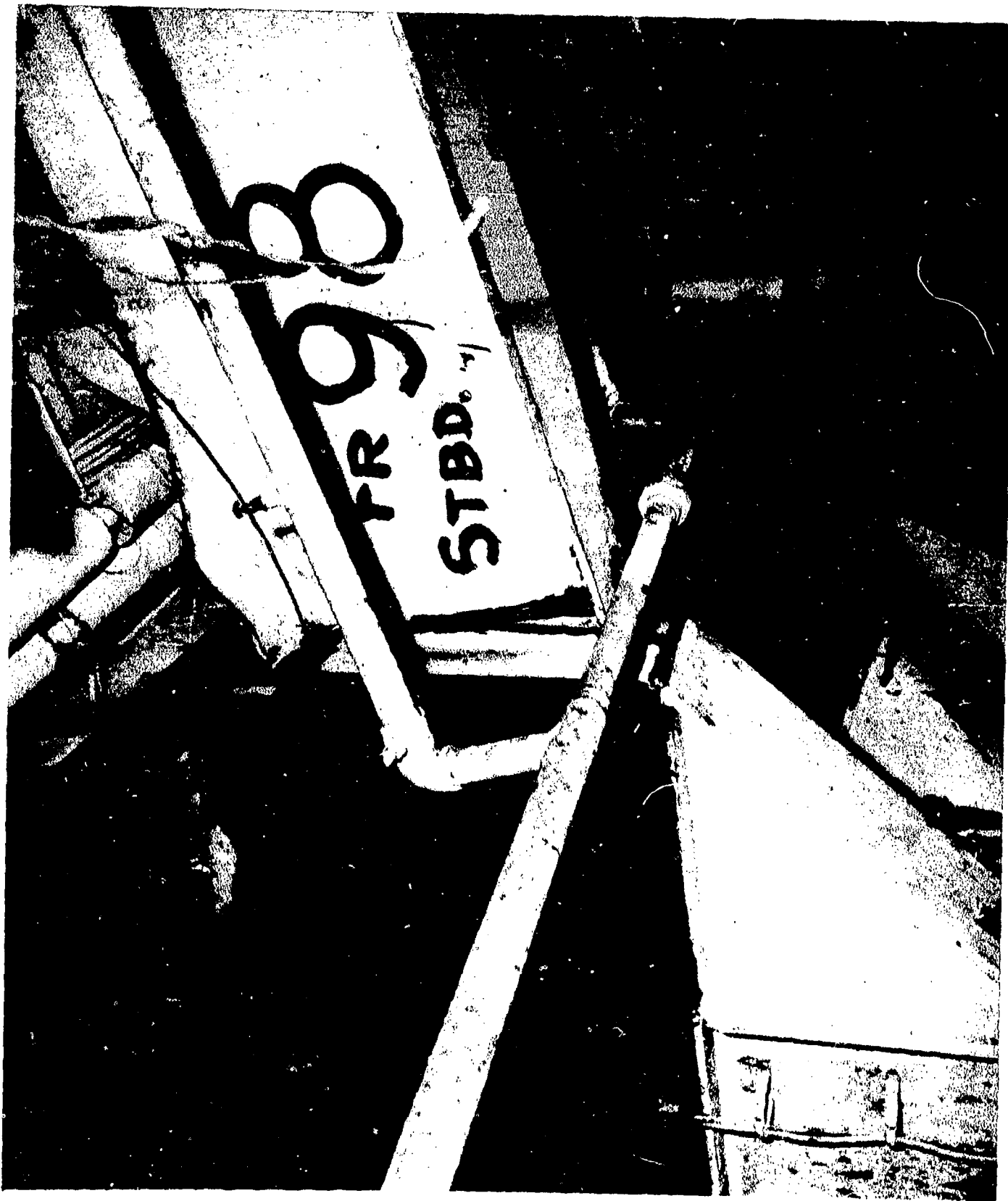
AA-CR-59-4149-9. Flight deck Bent 98, showing failure of overhead connection and origin of failure at edge of weld at top of bracket. Looking aft.
