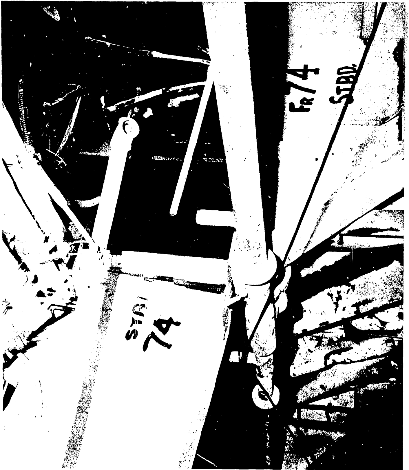
AA-CR-59-4148-11. Flight deck Bent 74, starboard side, showing failure adjacent to weld. Looking forward.
