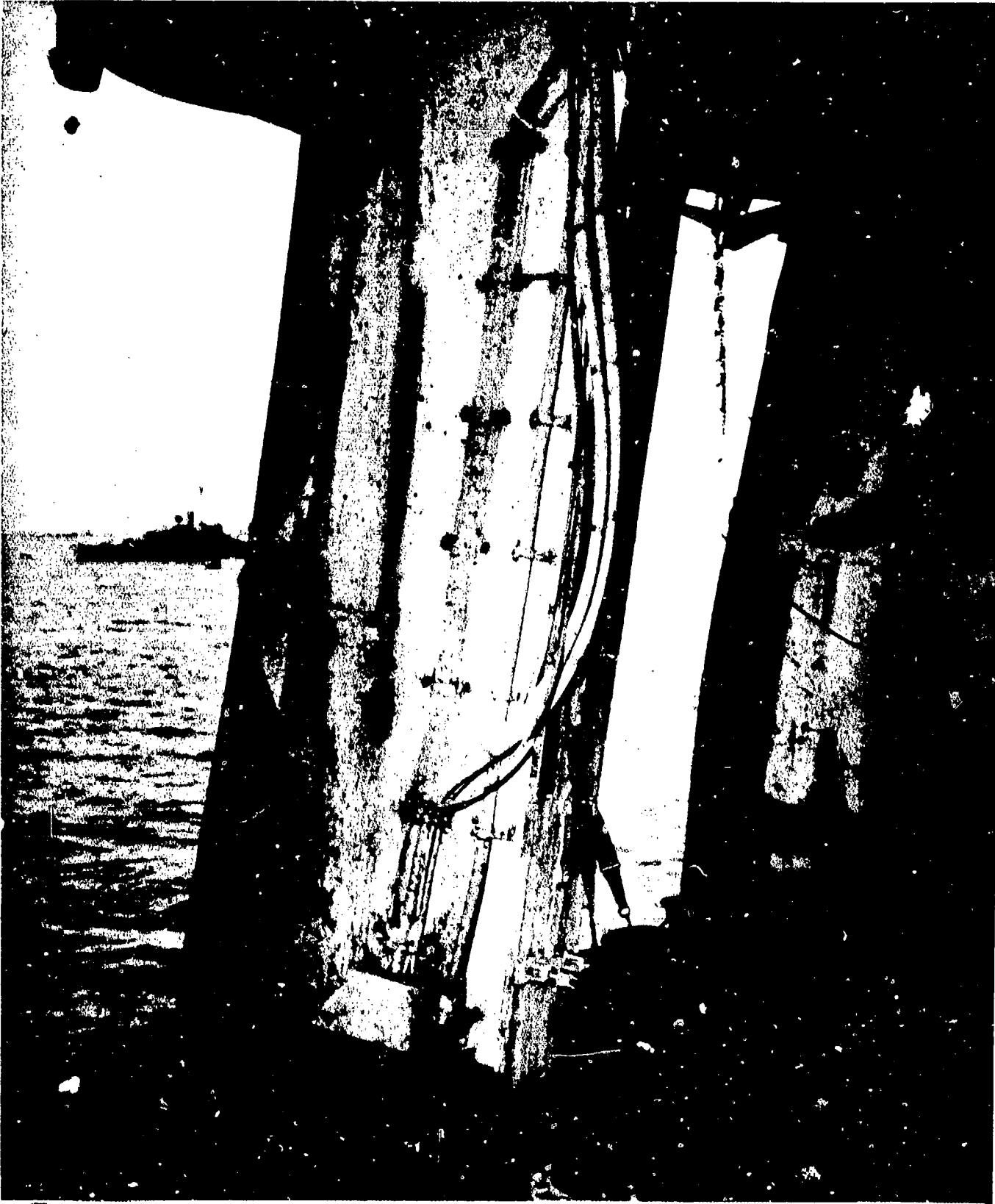
AB-CR-80-170-4. After Baker. Flight deck Bent 101, port bottom, looking forward.
