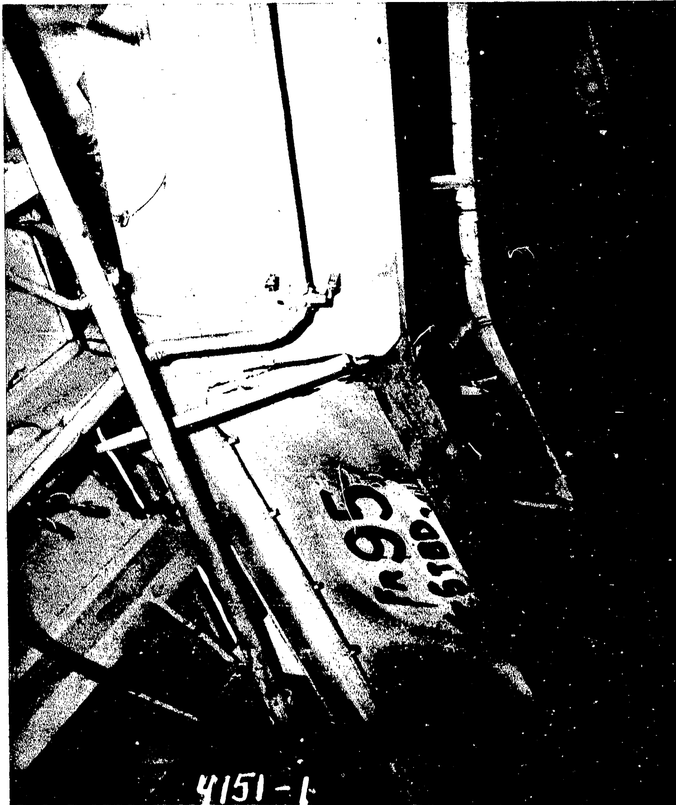
AA-CR-59-4151-1. Flight deck Bent 95, showing failure of transverse girder at welded centerline butt. Looking aft and to starboard.
