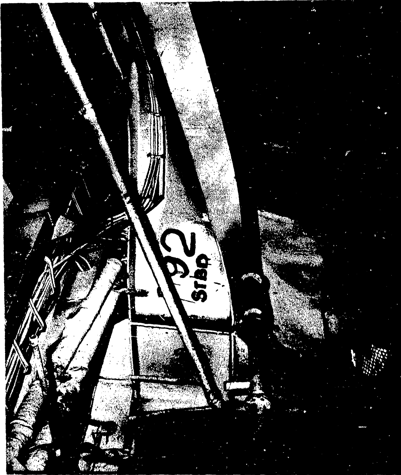
AA-CR-59-4149-7. Flight deck Bent 92. Starboard upper corner, looking aft.
