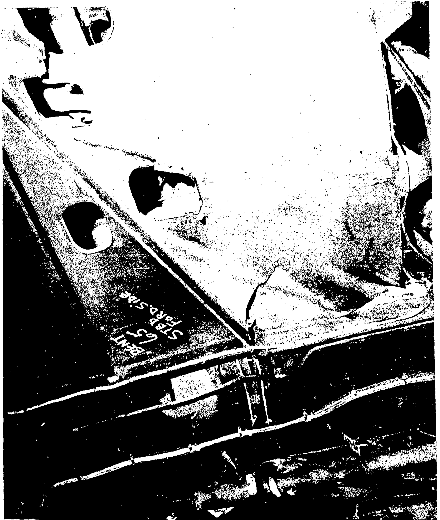
AA-CR-59-2222-5. Flight deck Wobble Bent 65, starboard side. Failure of overhead connection stemming from weld fracture at intersection of bracket and vertical member. Looking aft.
