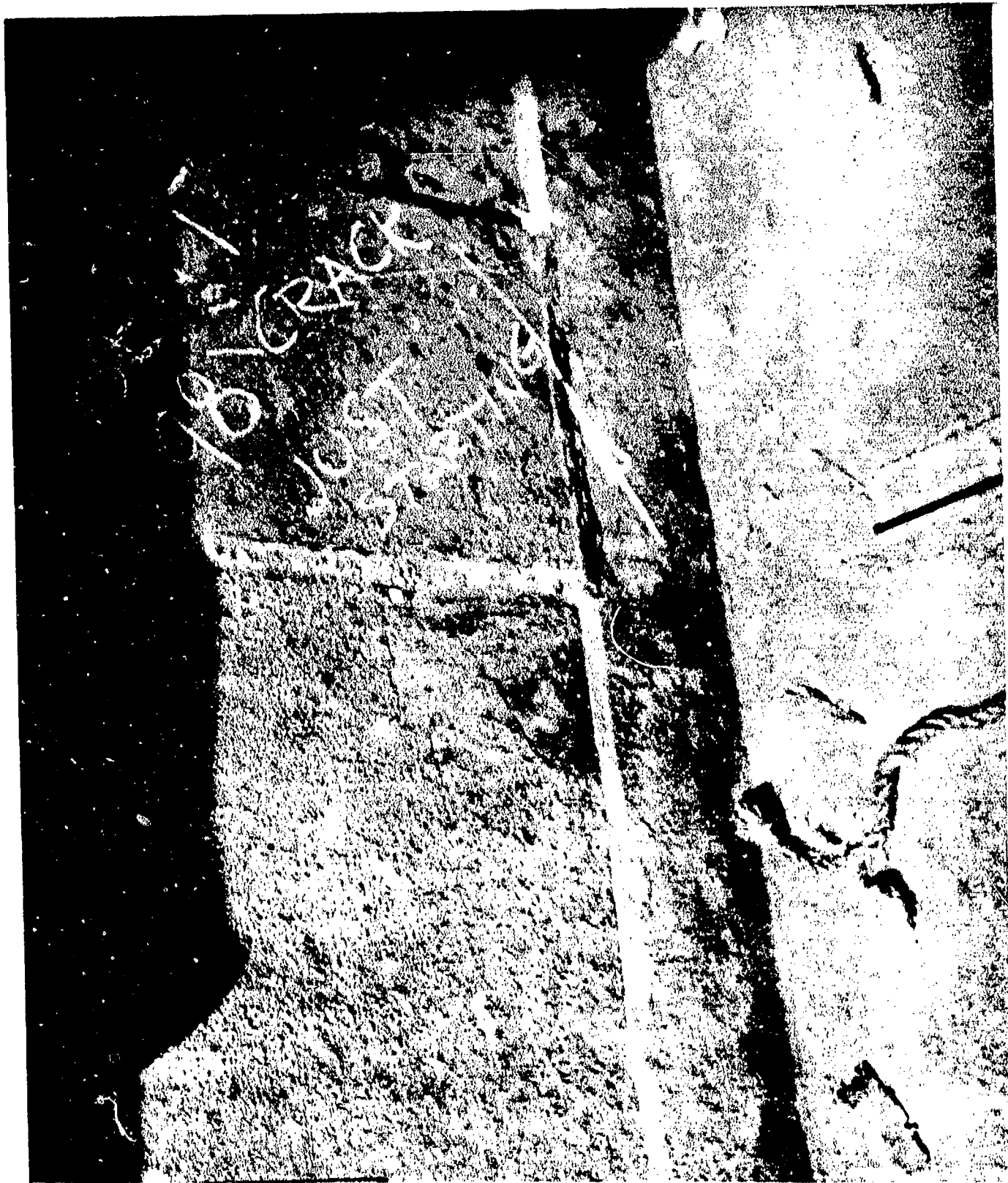
AA-CR-100-4161-2. Weld failure of port side connection of flight deck Bent 98 to S.T.S. shear strake. Looking inboard and to starboard.
