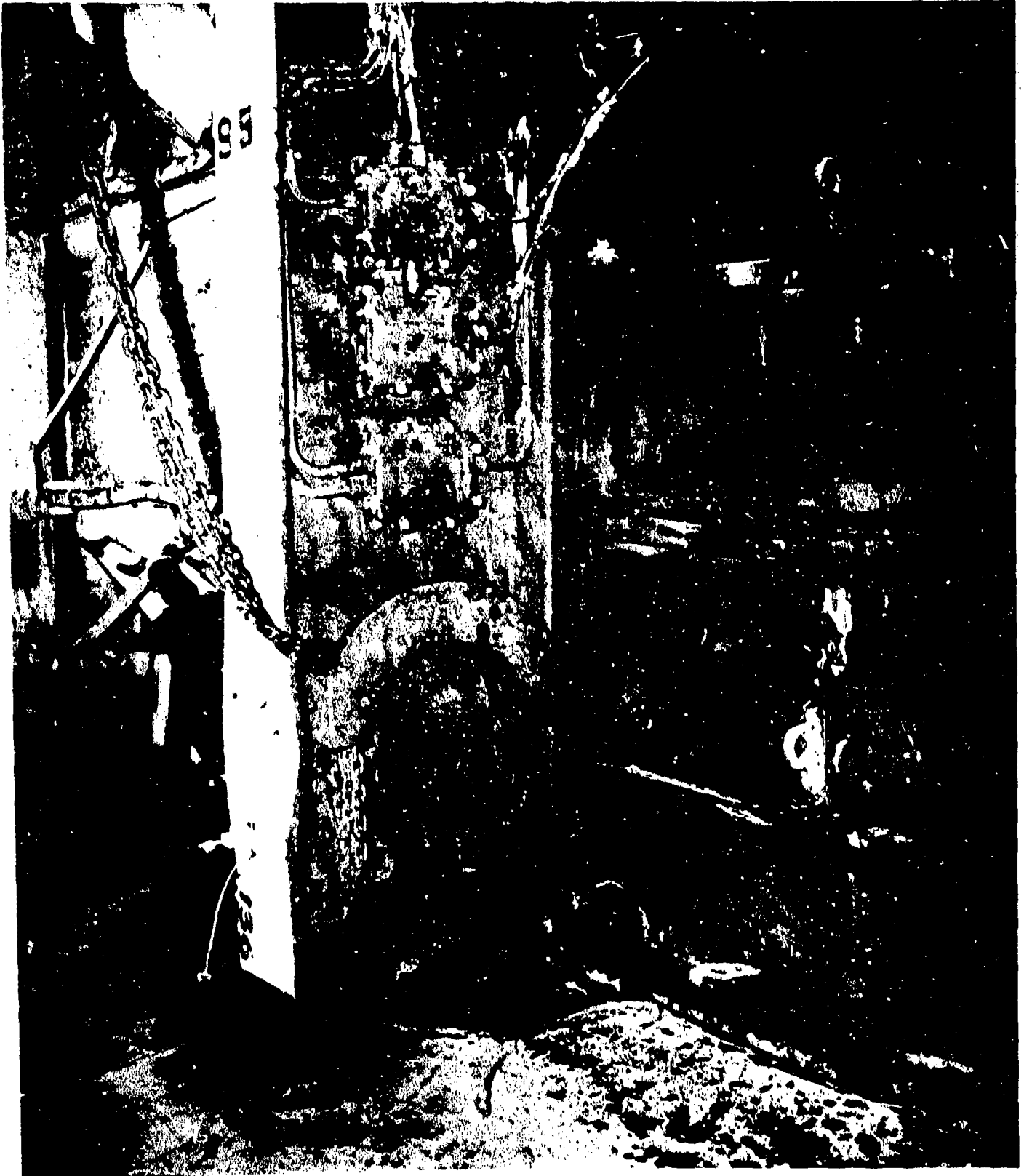
AB-CR-80-4187-12. After Baker. Flight deck Bent 95, starboard bottom, looking forward.
