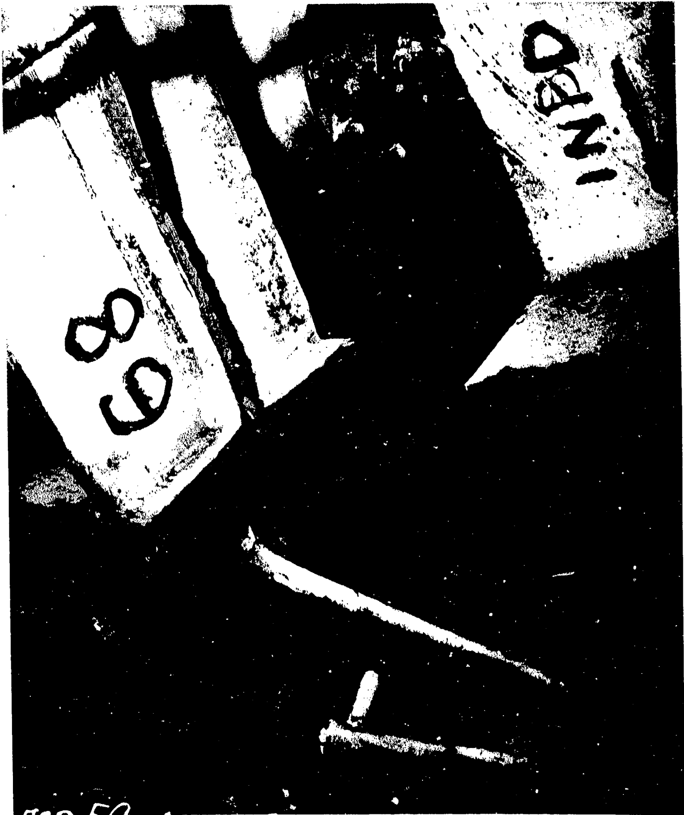
AA-CR-59-4149-5. Flight deck Bent 68, port side, inboard view. Fracture in vertical member below bracket connection. Looking upward and aft.
