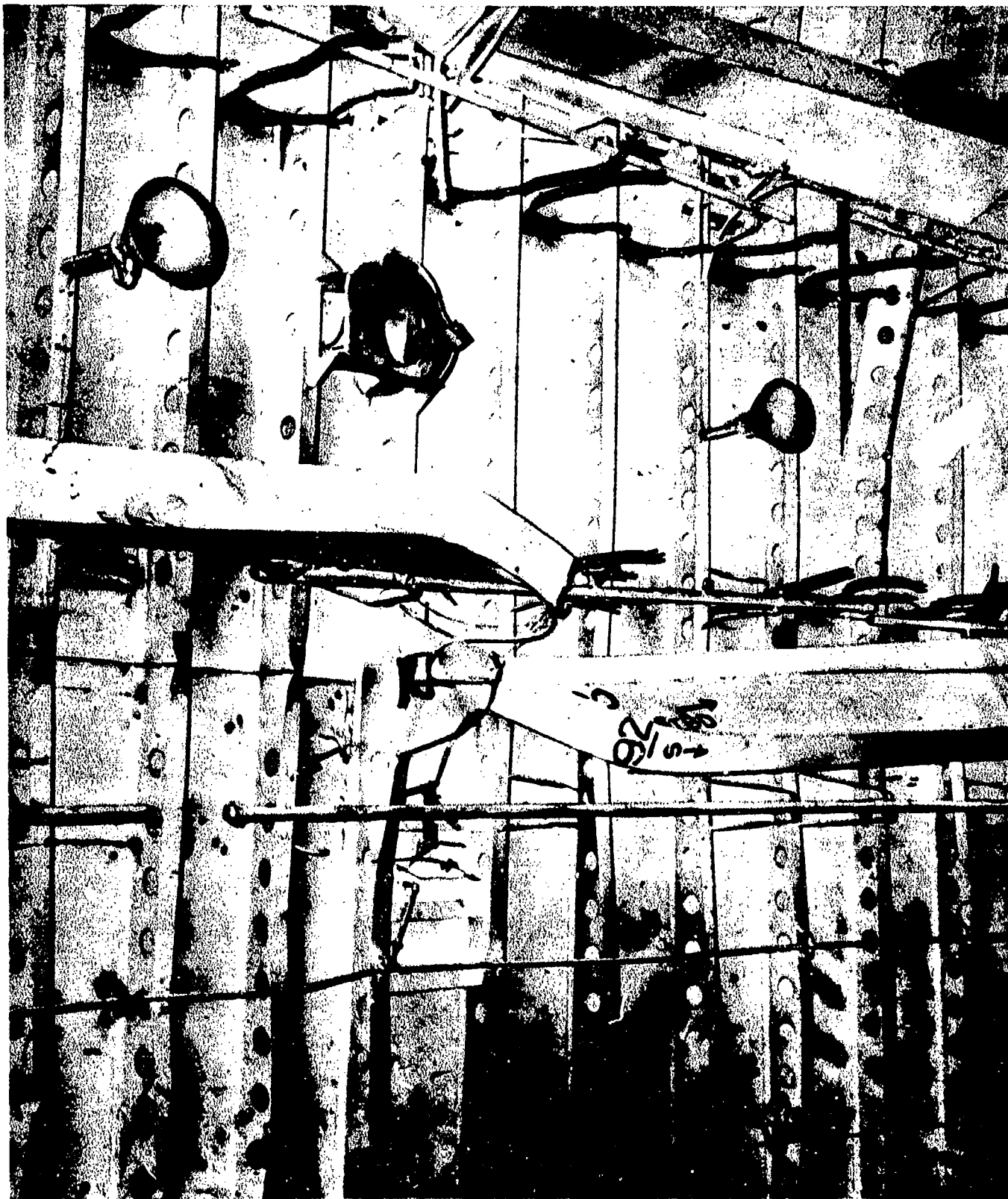
AA-CR-59-2224-9. Flight deck bent girder 92, looking to starboard.
