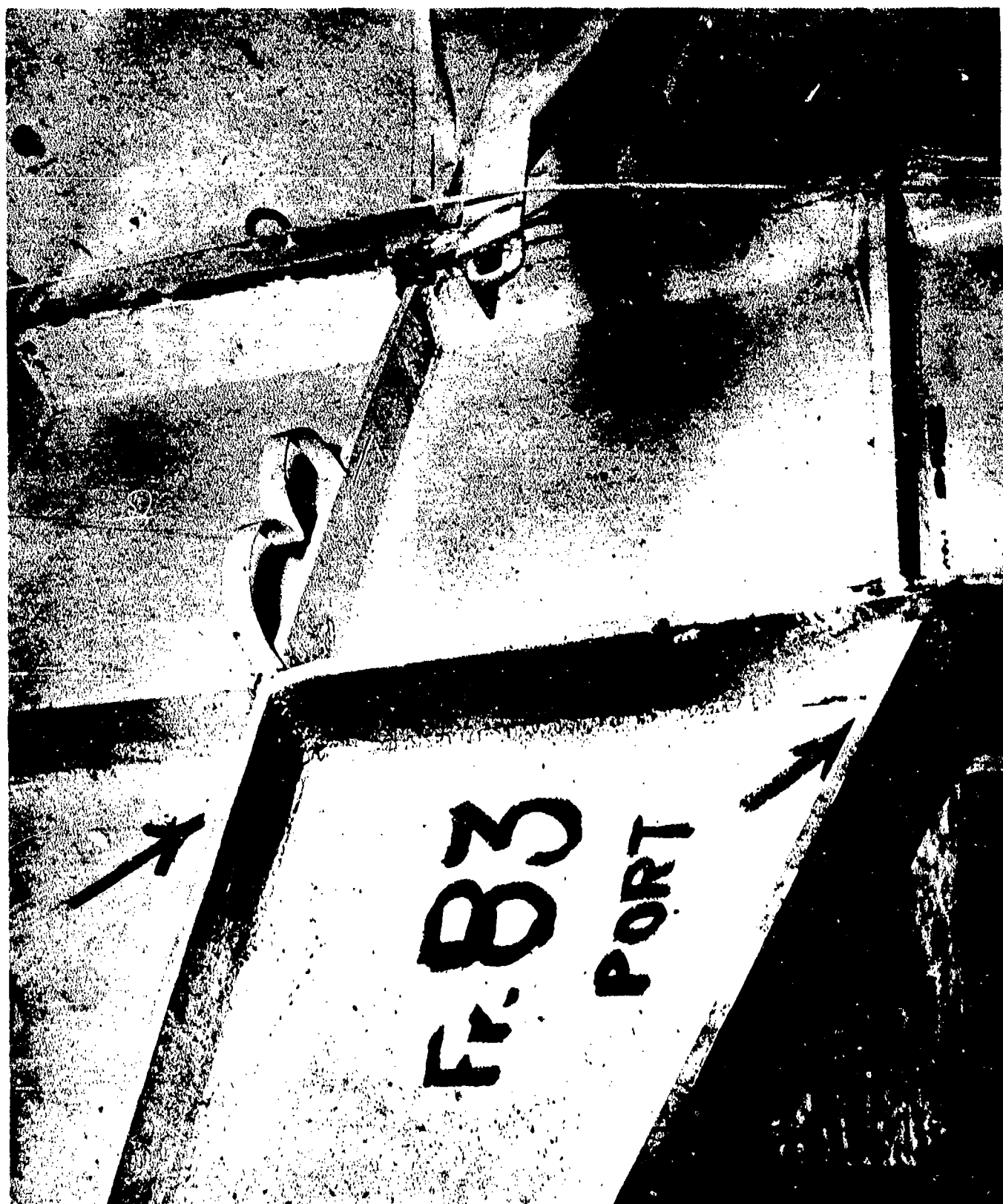
AA-CR-59-2223-7. Flight deck Bent 83, port side failure of welds in overhead connection. Looking aft.
