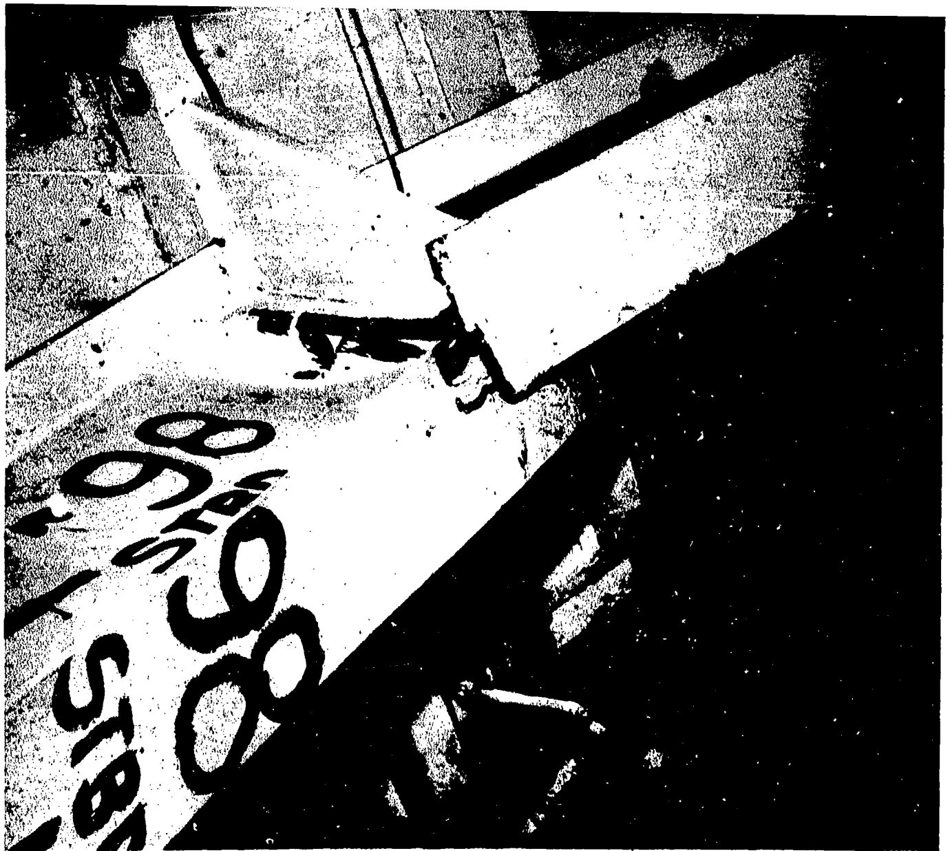
AA-CR-100-4151-4. Flight deck Bent 98, showing failure of centerline butt at weld. Looking aft and to port.
