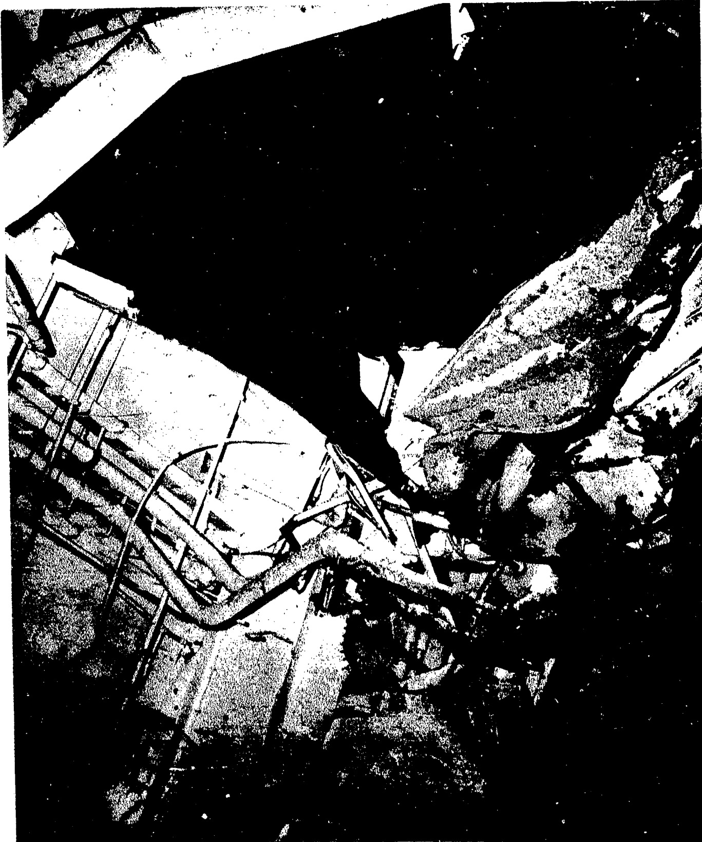
AA-CR-175-2131-1. Flight deck Bents 68 and 71. Failure of starboard overhead connections in welds. Looking forward from frame 73.
