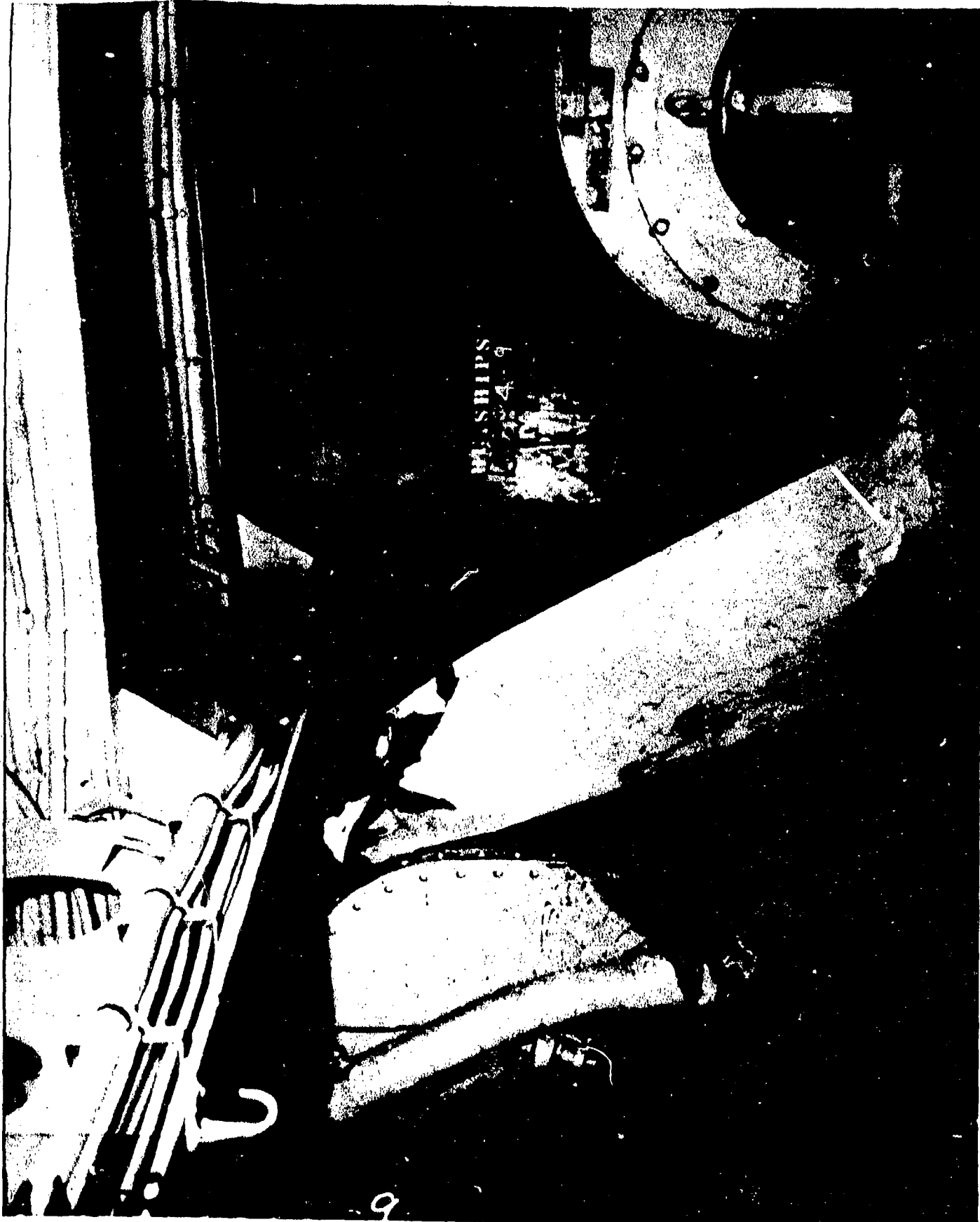
AA-CR-80-1894-9. C-201L. Vent duct crushed by deflected main deck girder, frame 08, starboard.
