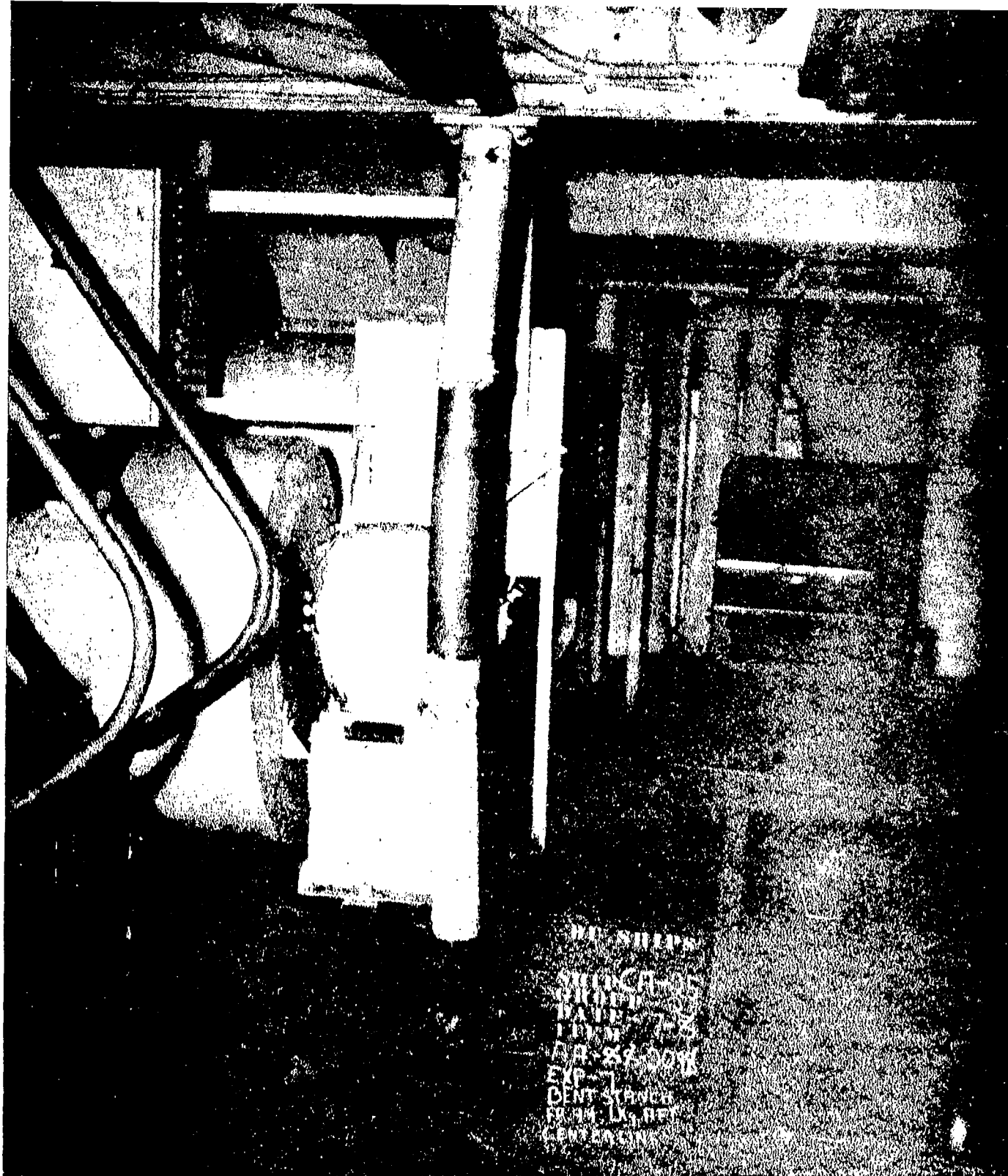
AA-CR-88-2098-7. C-202L. Looking aft at bent centerline stanchion, frame 94.
