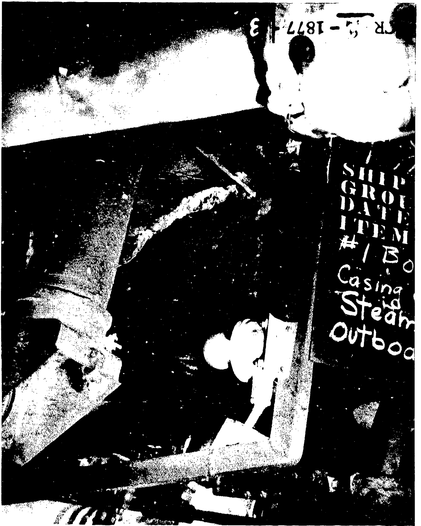
AA-CR-62-1877-3. No. 1 boiler casing at steam drum, outboard side, front.
