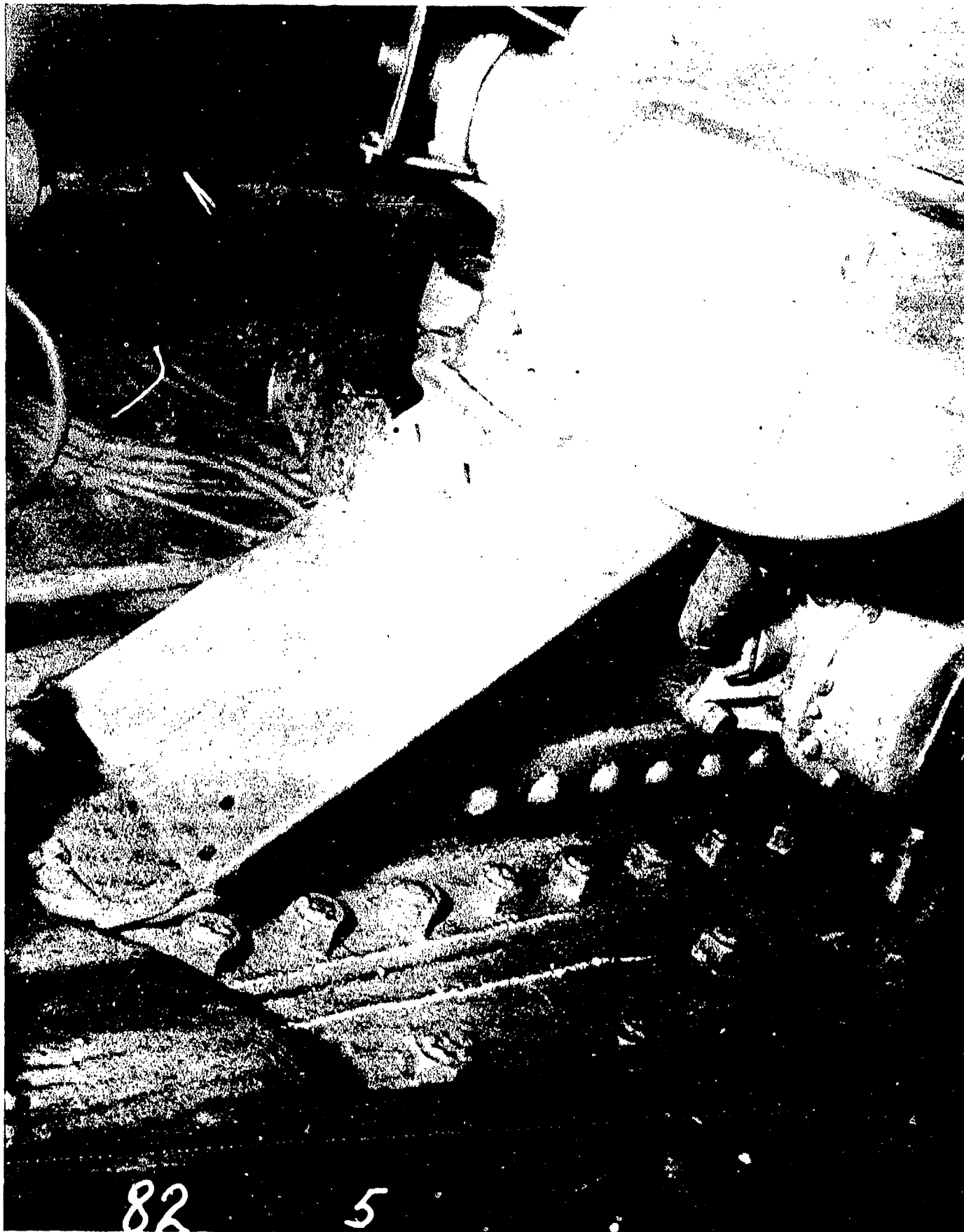
AA-CR-82-1915-5. Mount No. 1, left trunnion to support, looking to right and to rear. Structural bracket bracing the trunnion support to the shelf plate.
