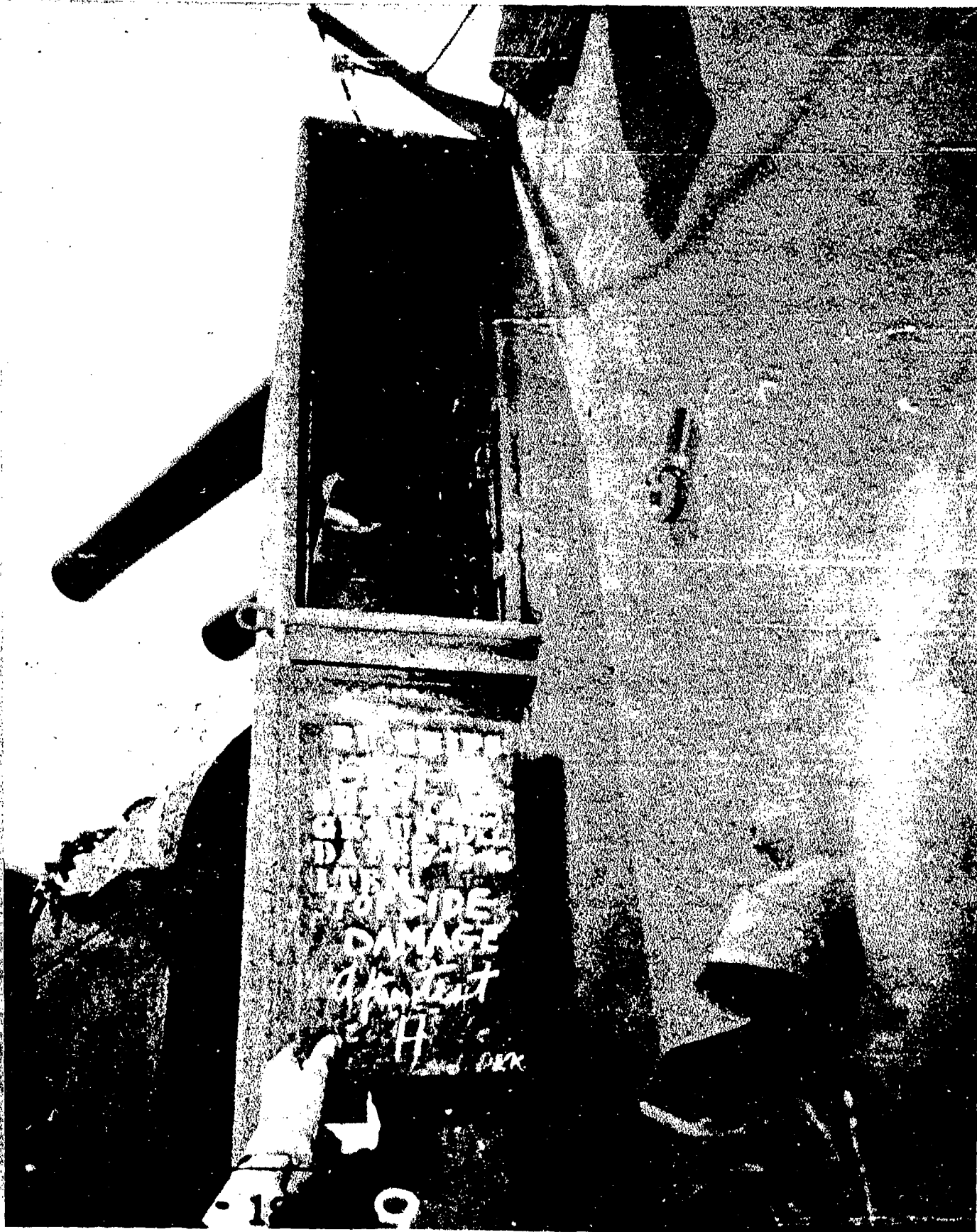
AA-CR-62-1861-9. Pushed in vent duct cover at frame 30, port, main deck.
