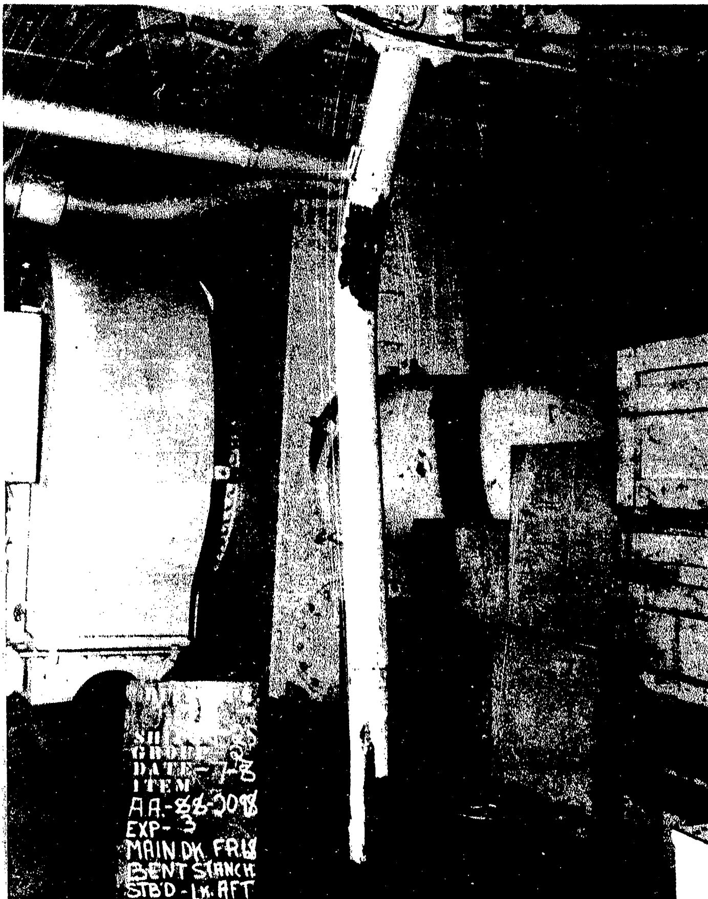
AA-CR-88-2098-3. C-201L. Looking aft at bent stanchion under main deck at frame 68, starboard.
