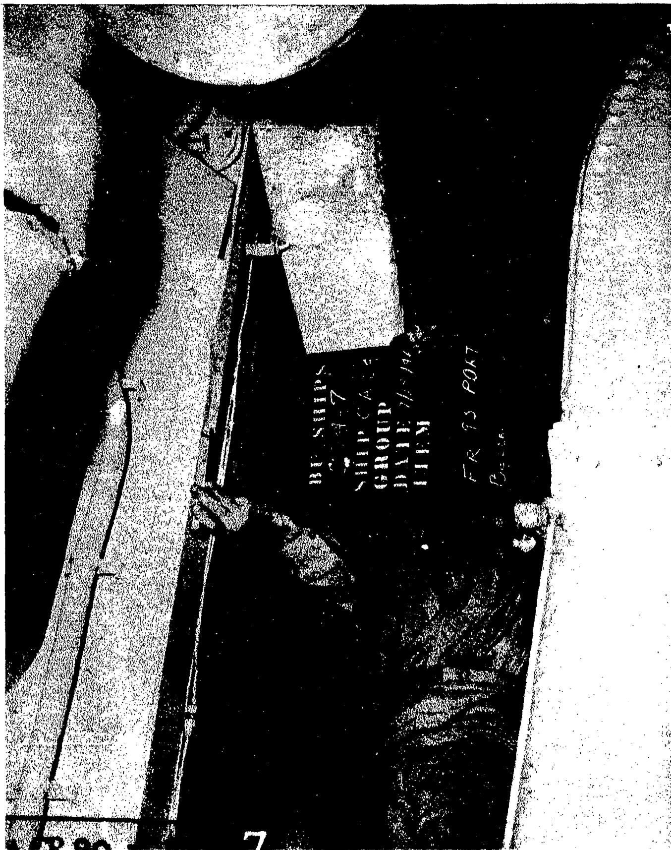
AA-CR-90-574-7. C-2. Looking aft in after engine room, port side, showing buckle in flange of transverse girder at frame 93 under 2nd deck.
