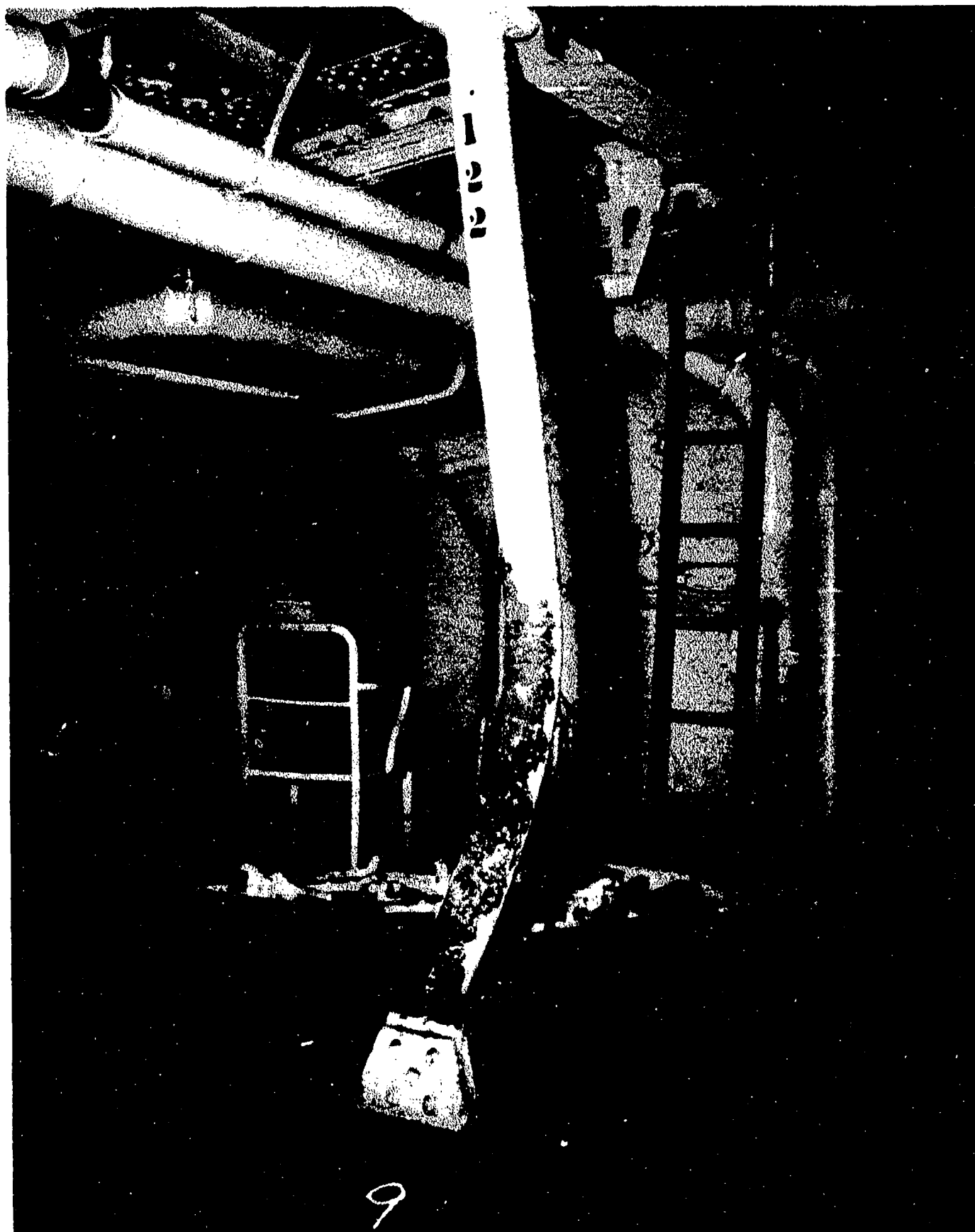
AA-CR-175-2178-9. Looking aft and to port on 2nd deck, starboard side, showing stanchion failure at web frame 122.
