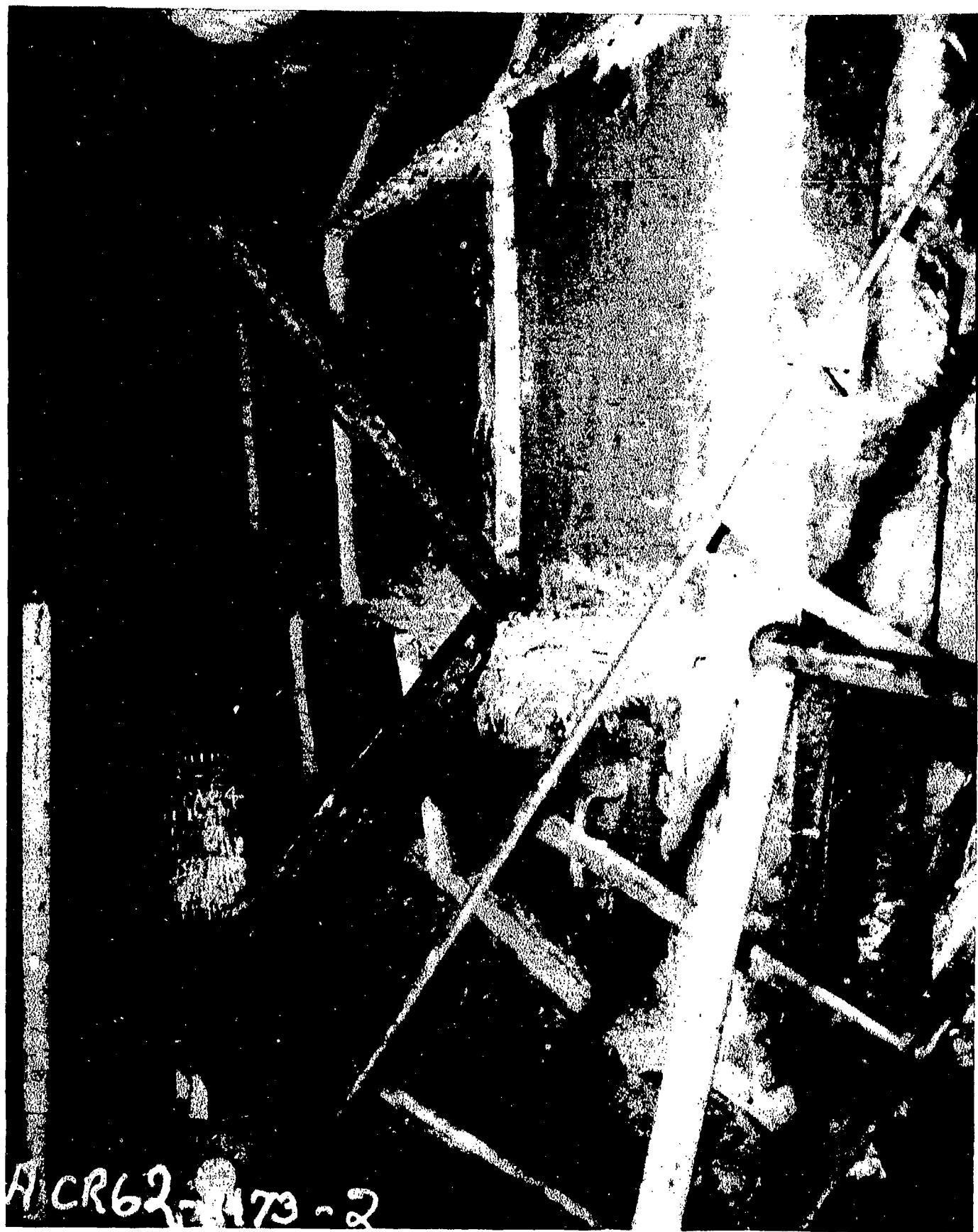
AA-CR-62-2173-2. #7 Boiler, repaired outboard casing.
