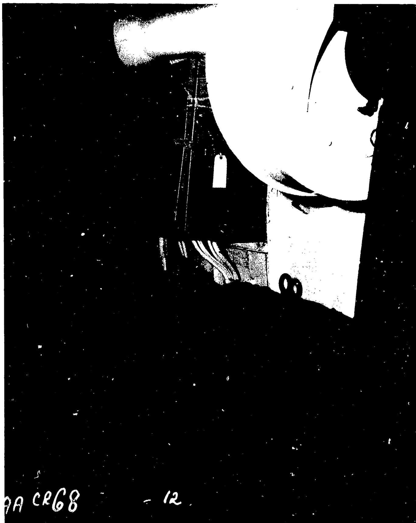
AA-CR-68-1755-12. Motor controller for radio motor generator, panel is cracked due to distortion of supporting bulkhead.
