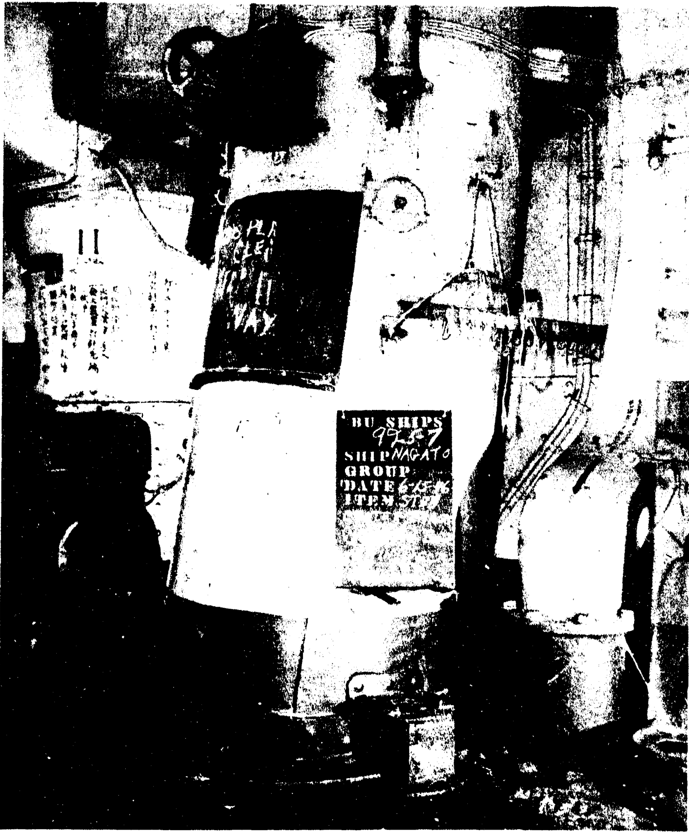
BA-CR-78-925-7. Center leg, starboard side, main deck, sextipolar mast. Base at frame 107.
