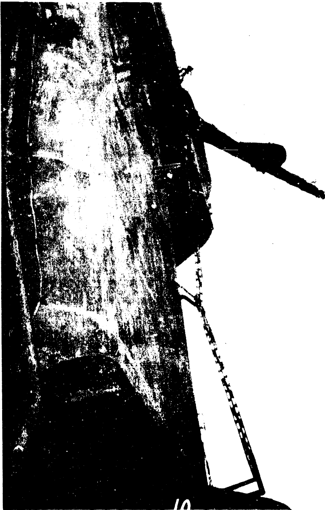
AA-CR-79-1816-10. Looking upward at after face of foremast structure showing light dishing of panel and bending of ladder.
