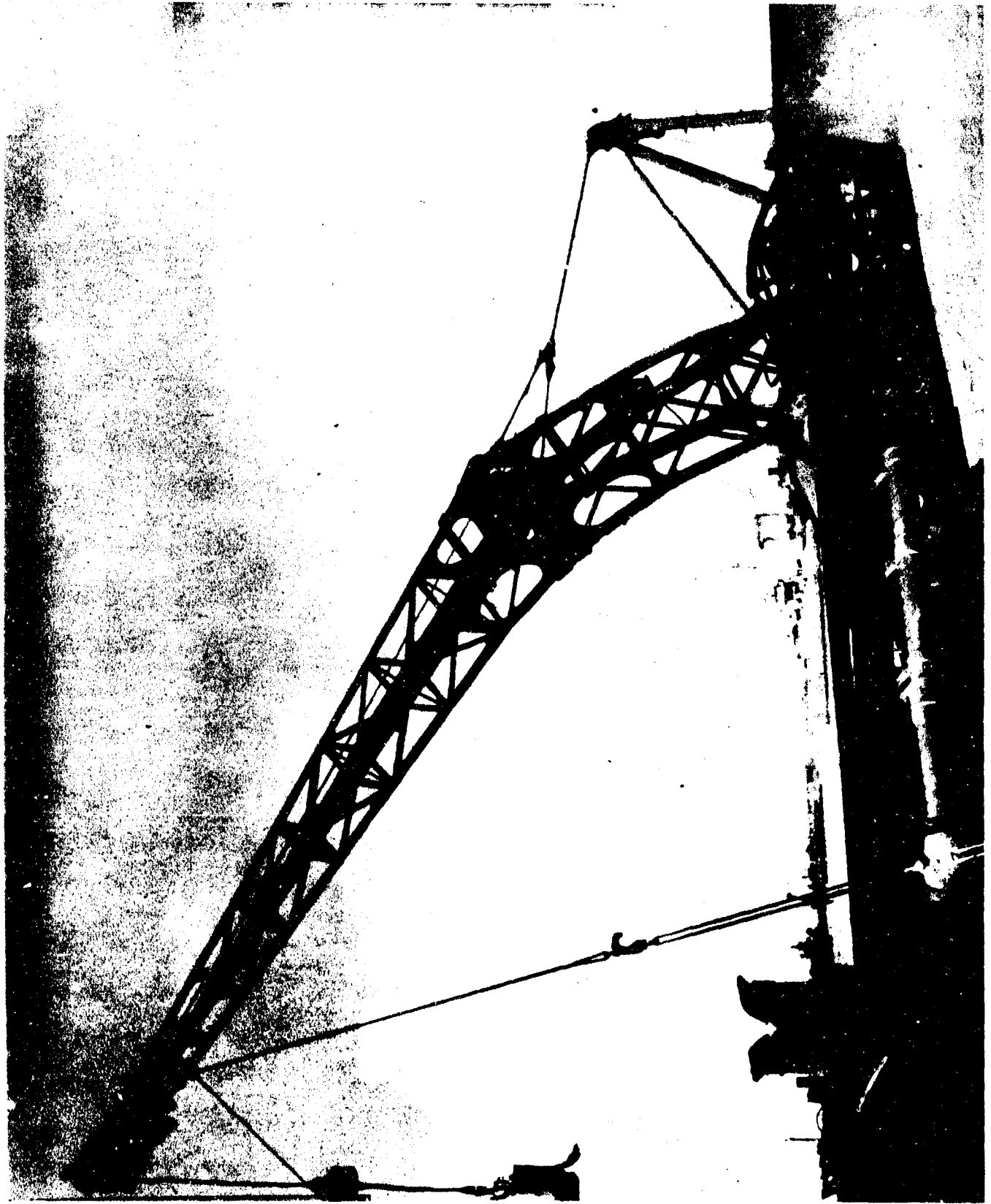
AA-CR-100-1889-9. Stern crane, showing lower section buckled and resting on the catapult. Looking aft and to starboard.
