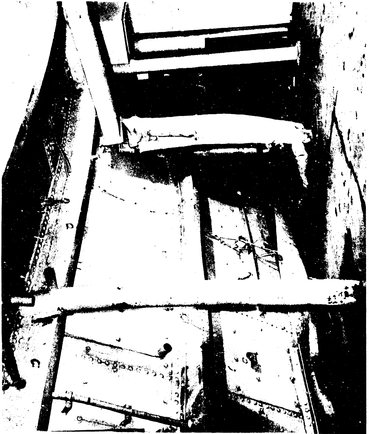
AA-CR-175-2136-10. Compartment C-291-1L. Looking forward and to starboard on second deck at after portion of collapsed main deck (port side of frames 86-91). Note buckled stanchion at frame 91.
