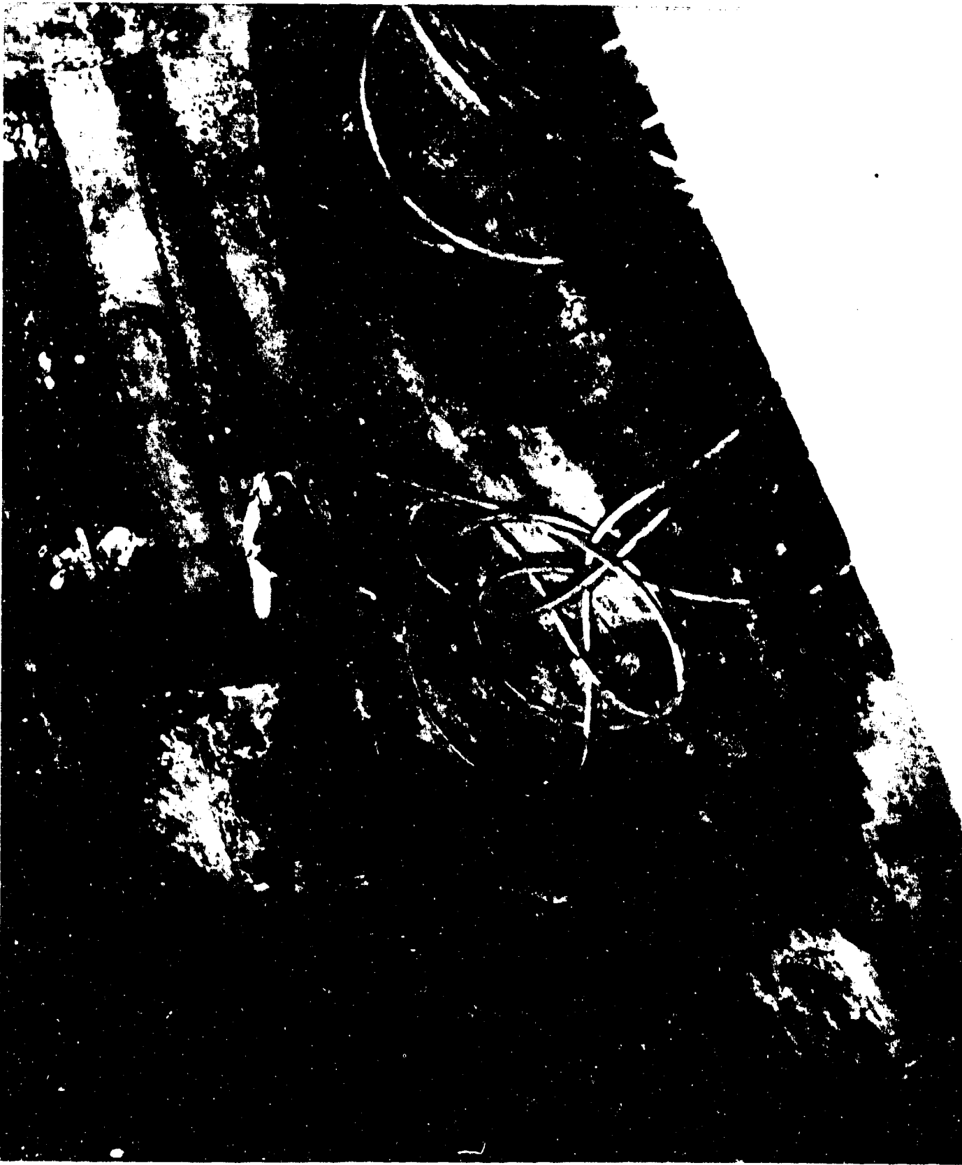
AA-CR-65-1817-1. Burned area on main deck, frame 144, starboard, under burned coil of line.
