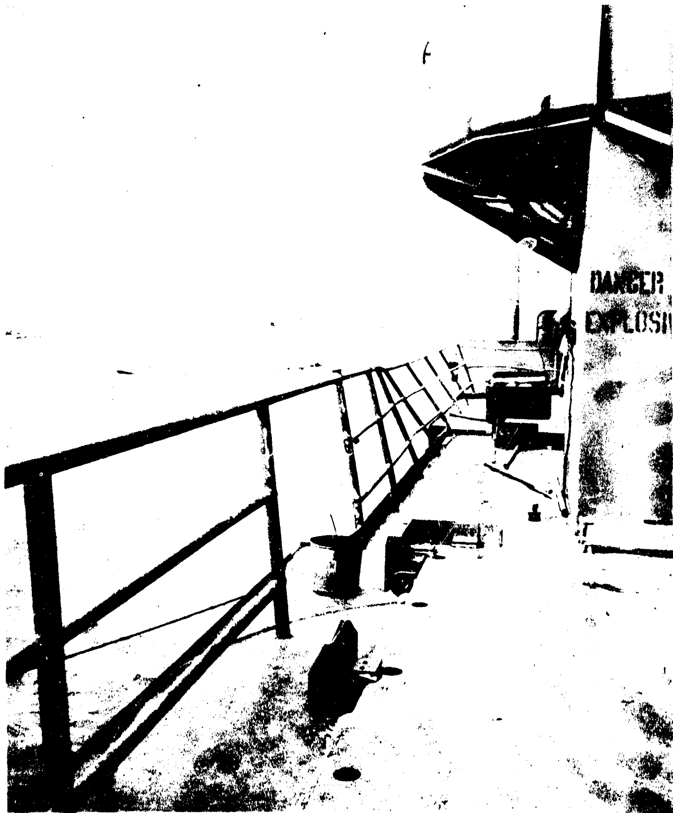
AA-CR-175-2154-11. Looking aft along starboard side of superstructure deck from frame 62 showing damage to the handrail.
