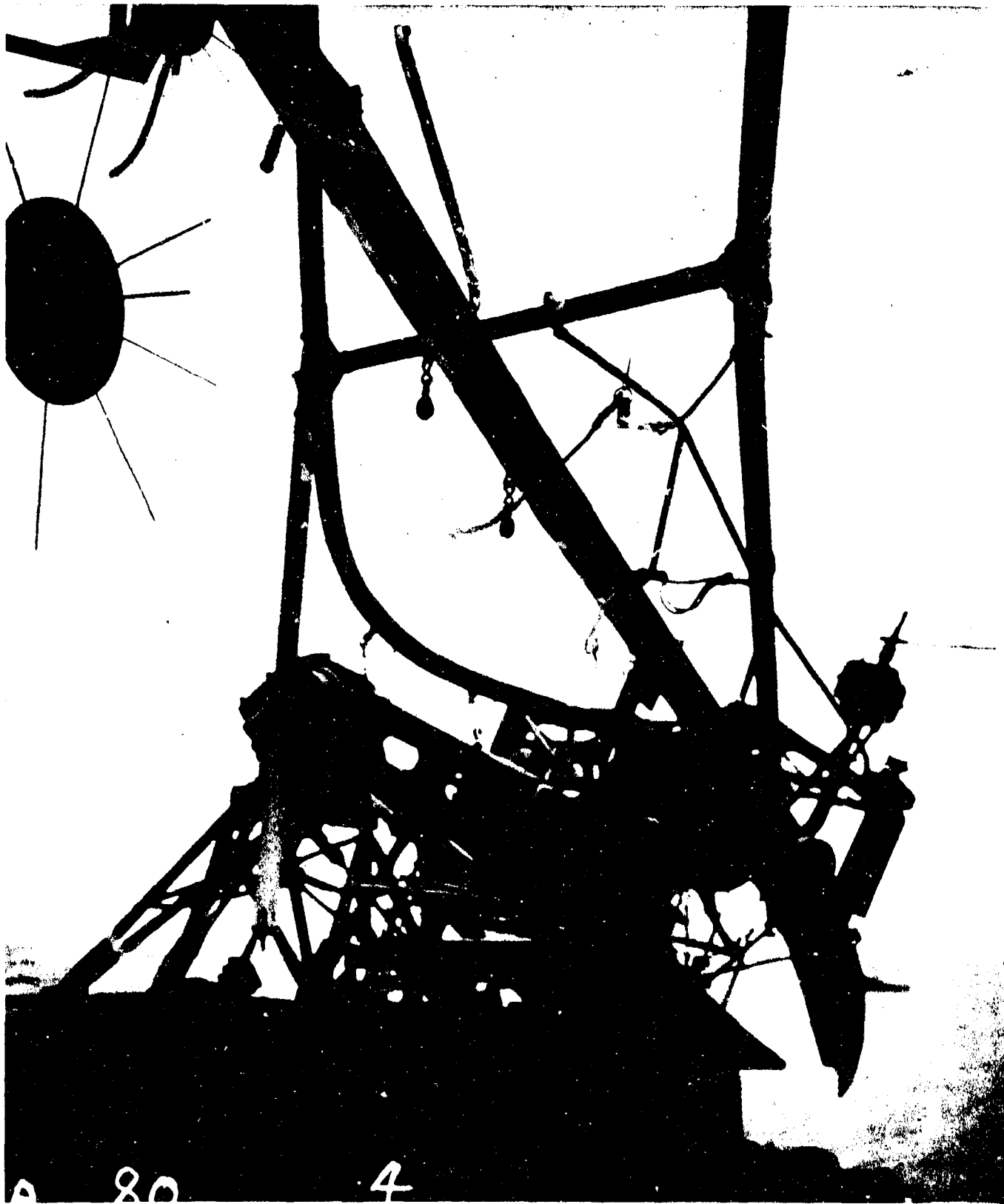
AA-CR-80-1900-4. Forward tripod, view looking forward at wreckage of starboard yardarm. Main member, truss and forward strut.
