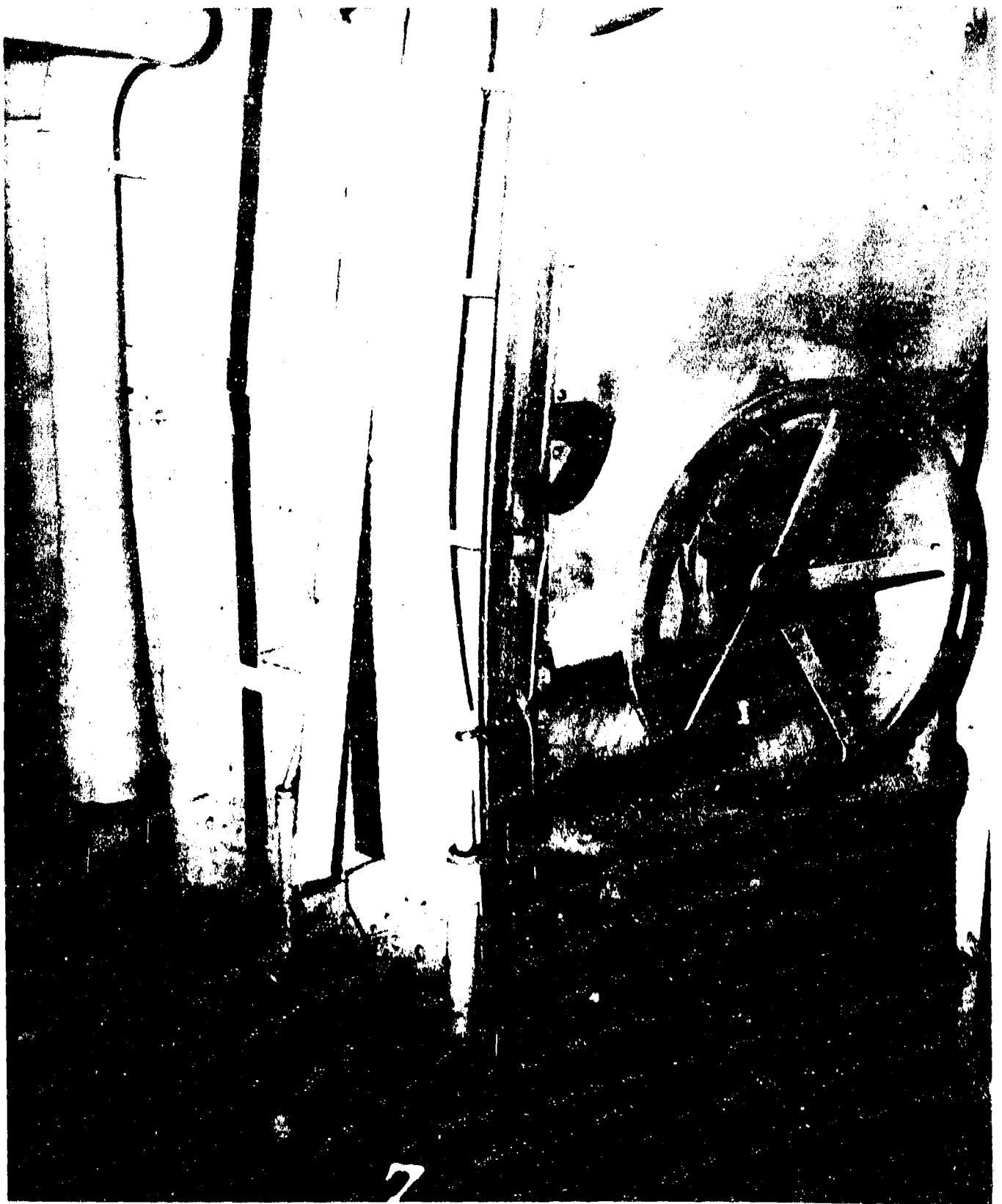
AA-CR-175-2136-7. Quick acting watertight door, in port side of bulkhead 97, looking forward and to port. Door is buckled aft 3 1/2 inches.
