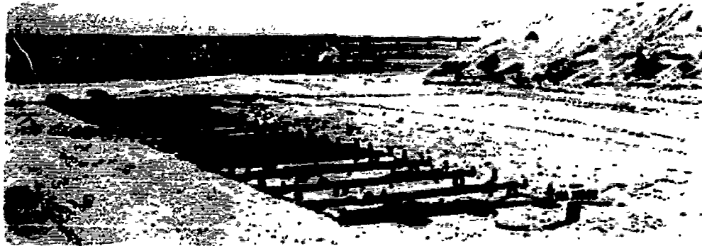
Figure 3.10 Pretest view of one-way slabs at Station 360.02, range 3,100 feet. Ground zero is to the left.
