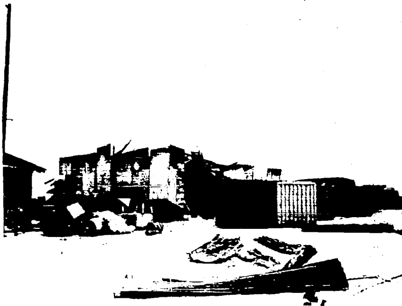
Fig. 3.28 Bulk Storage Warehouse from Northwest, Tare Island, Postshot, 14-3/4 Miles from GZ
