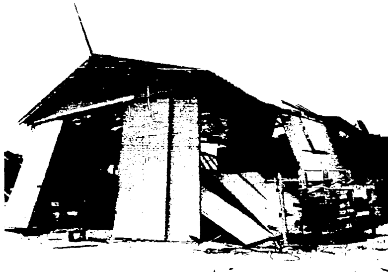
Fig. 3.24 Bin Storage Warehouse Looking Southwest, Tare Island, Postshot, 14-3/4 Miles from GZ
