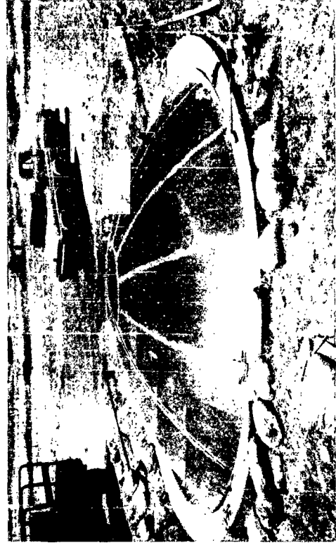
Figure 3.33 Foundation for aluminum dome. Two halves of shell are shown in background.
