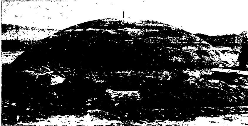
Figure 3.30 Finished concrete dome. Entrance to inside of dome shown through foundation.
