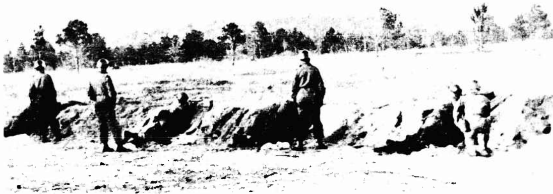
Fig. 4—SALVO II Firing Line Showing Modified Prone Position
