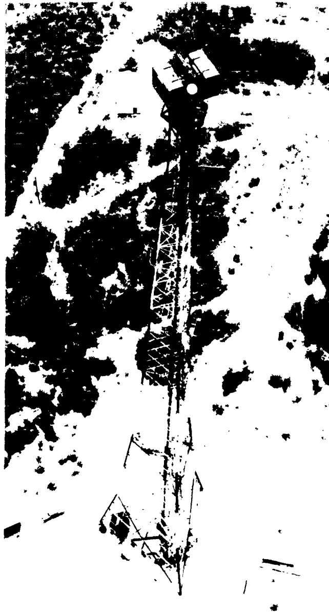
Fig. 15. Oakhurst tower (400 feet high) (U)
