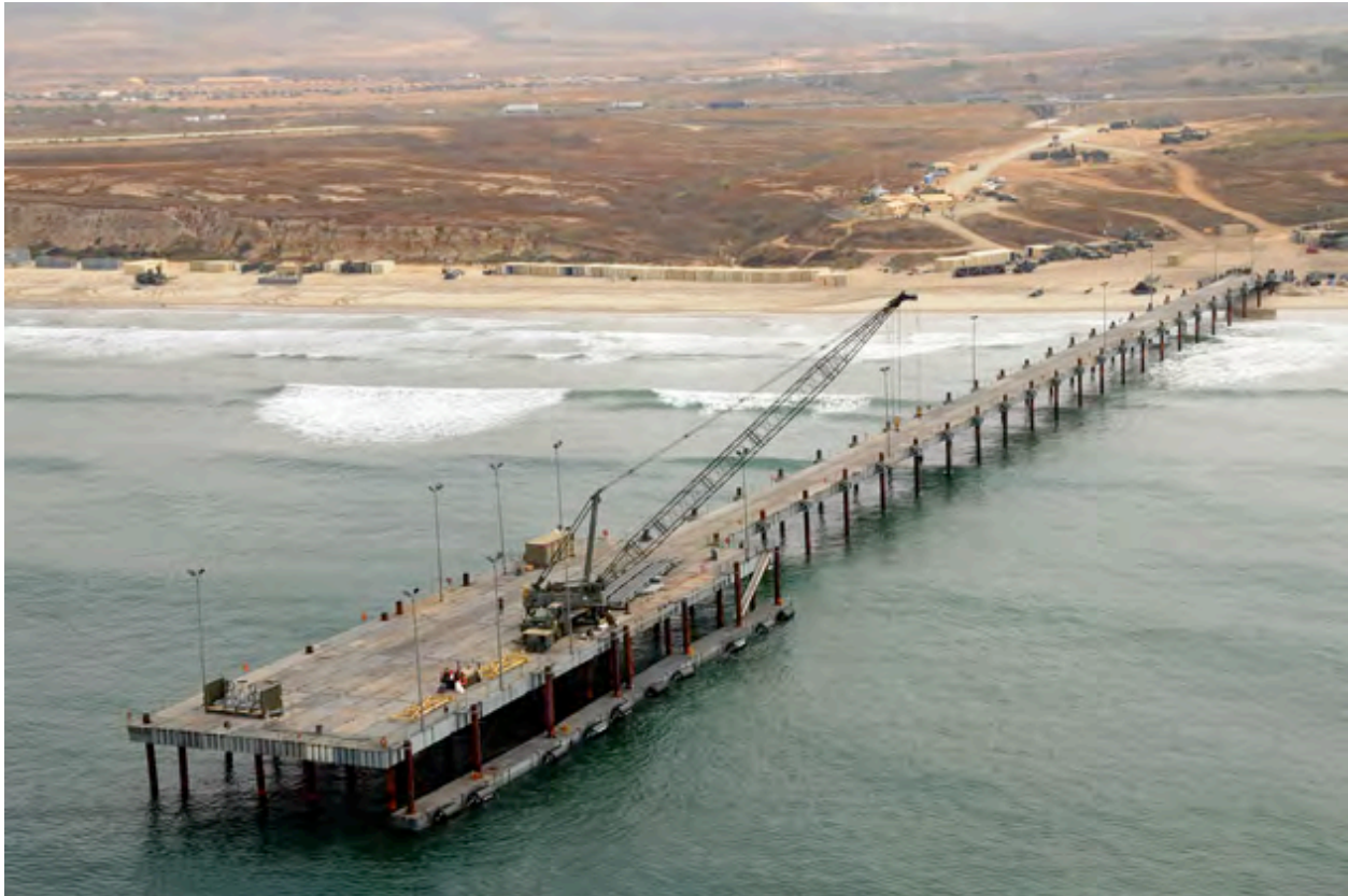
Figure 4 - Elevated Causeway (ELCAS) Photo 25
