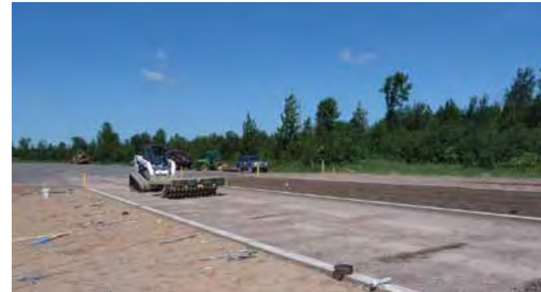
Image 2. SCAMP Roller with Bobcat T-250 prime mover.
