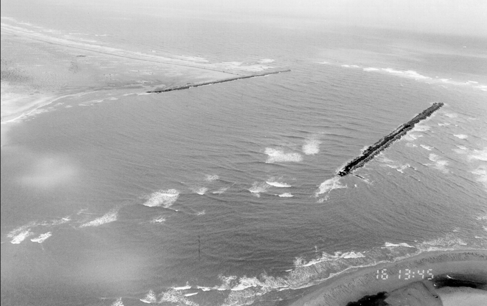
Figure 4. Example of flanked jetty at Mezquital Inlet, Mexico, creating channel competition to the Gulf of Mexico. (Photograph by N.C. Kraus, 1996.)
