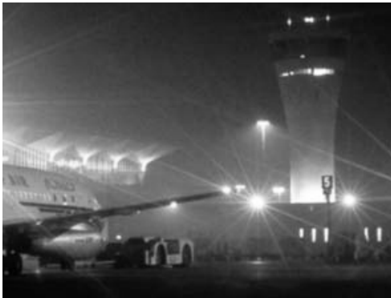
Figure 9: Glare from airport ramp lighting.
