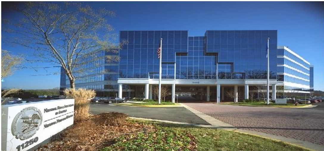
Figure 17. NRA Headquarters- Fairfax, Virginia
