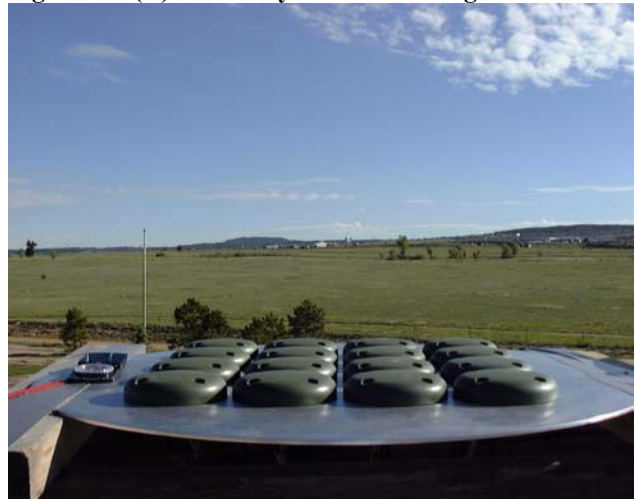
Figure 2 Sixteen Element HAGR Antenna Array
