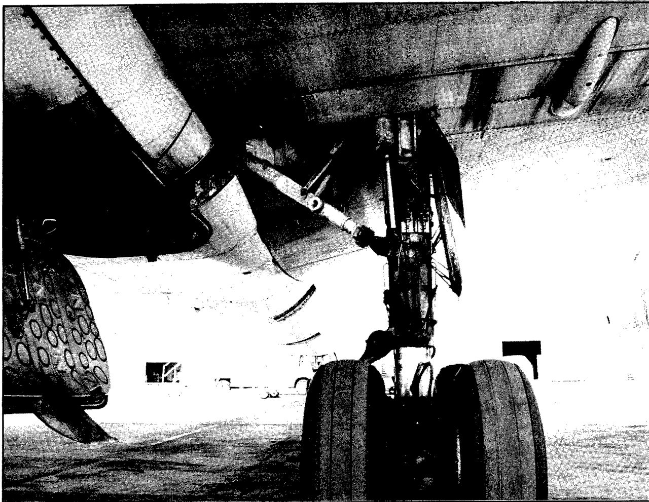
Figure 1. Wheel-Well Passenger Stow-Away Space. it is forward of DC-8 Right Main Landing Gear, Wing Root Area.
