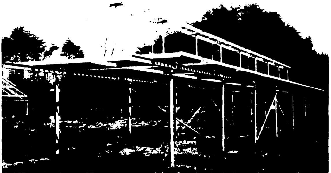
Figure 2 — A108-Mc Minitrack antenna
